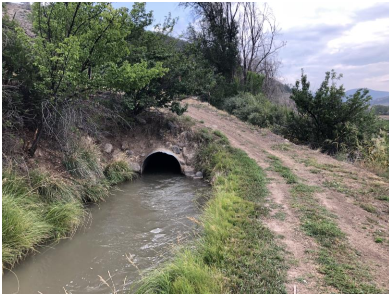
Lower end of 600-foot culvert at the Loadout (Farmers Ditch)
