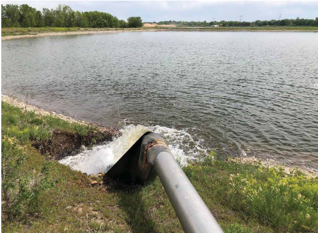
Photograph #1. DRMS inspection photograph of inlet water being discharged into the north reservoir.
