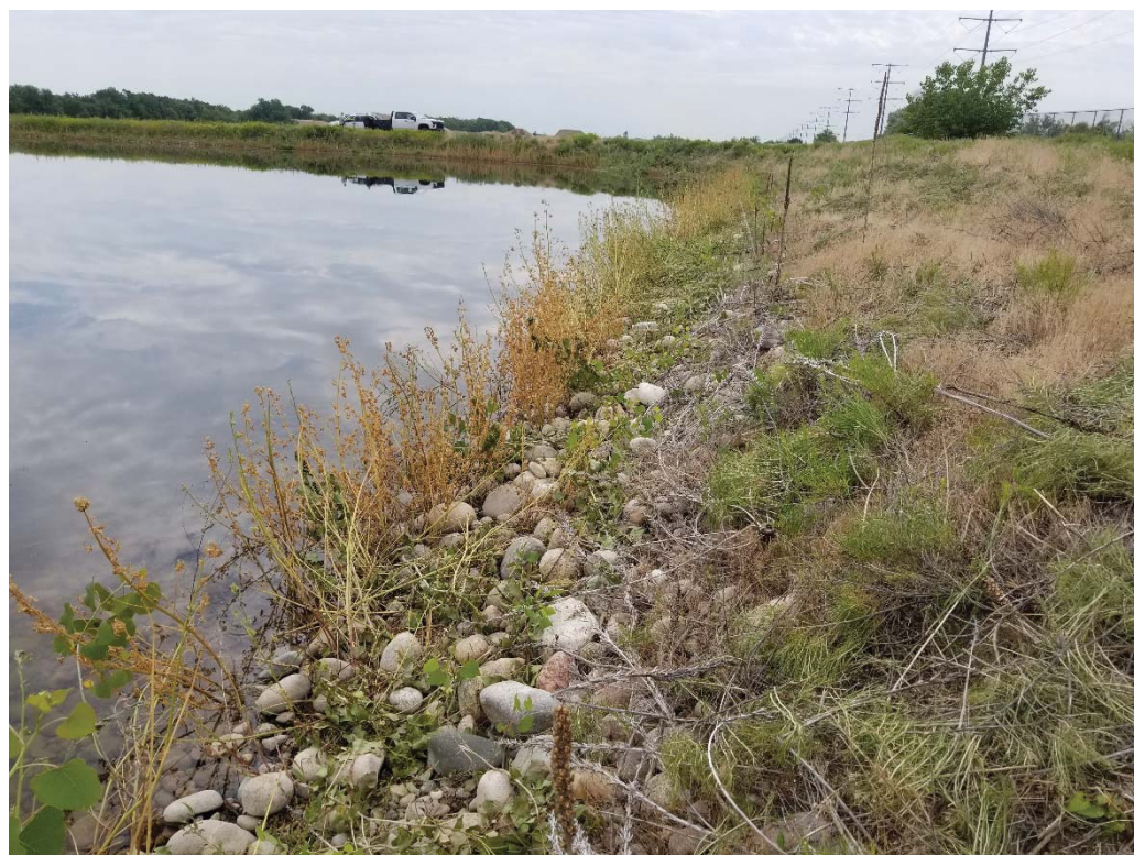
Photograph #6. Hand trimming on reservoir side slopes.
