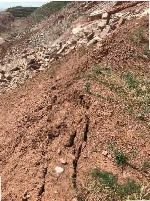
2. CRACKING ON FILL SLOPE
