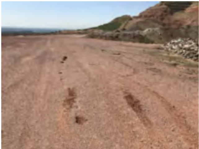
1. RECENT CRACKS ON PRODUCTION FLOOR AFTER RAIN
