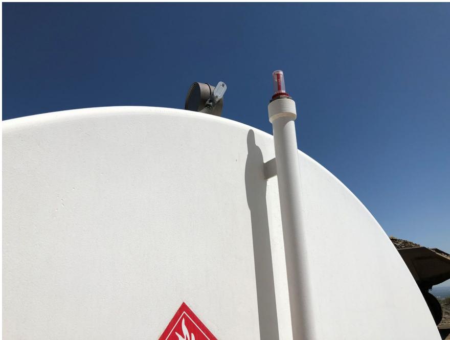
Leak detection on 12,000 gallon double-walled AST
