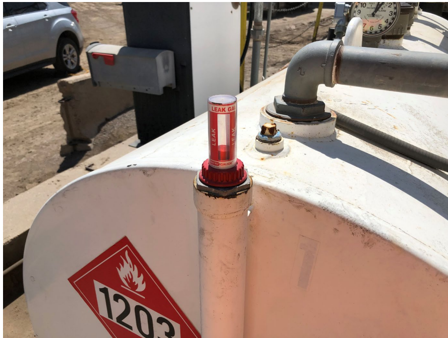
Leak detection on 1,000 gallon double-walled AST
