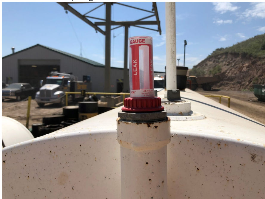
Leak detection on 3,000 gallon double-walled AST
