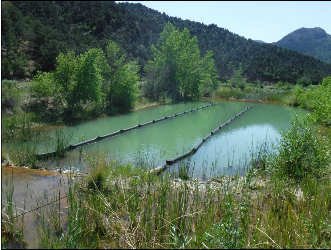
Photo 5: The first of five sedimentation cells, flow away from viewer
