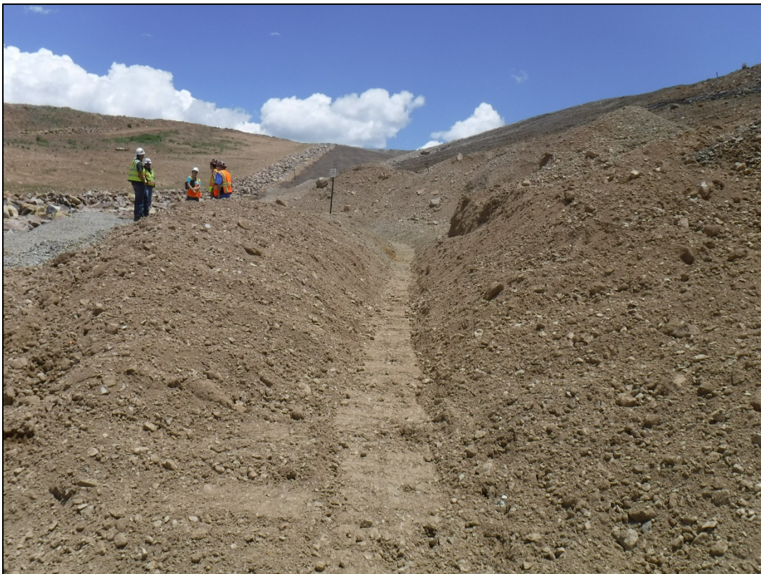
Photo 20: Berm and compacted trench to help prevent material and solution from migrating off liner
