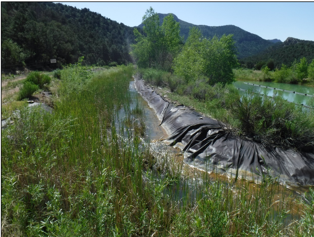
Photo 4: The lined channel coming from the initial holding pond to the sedimentation ponds, flow is towards viewer
