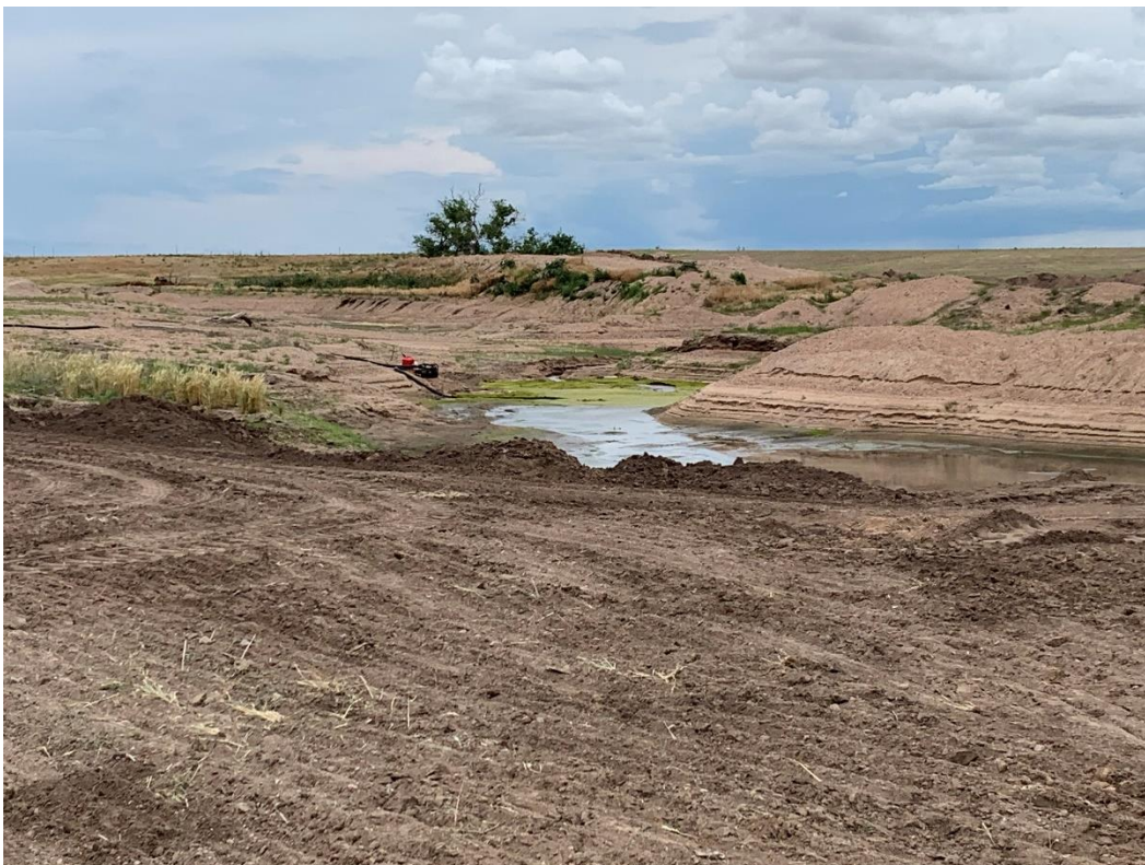
Photo 2 – Water in Coyote Creek with pump removing water
