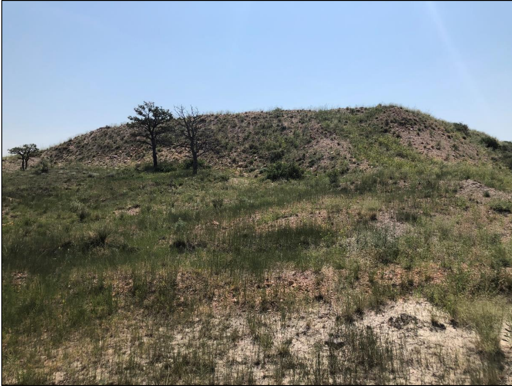
Photo 5. View looking south at large overburden stockpile stored in West pit disturbance area. This stockpile appeared to be stable with good vegetative cover.
