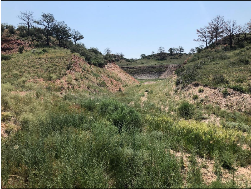
Photo 13. View looking southeast at western entrance to East pit. Note portion of unmined ridge visible at left, which can be utilized for highwall backfill material.
