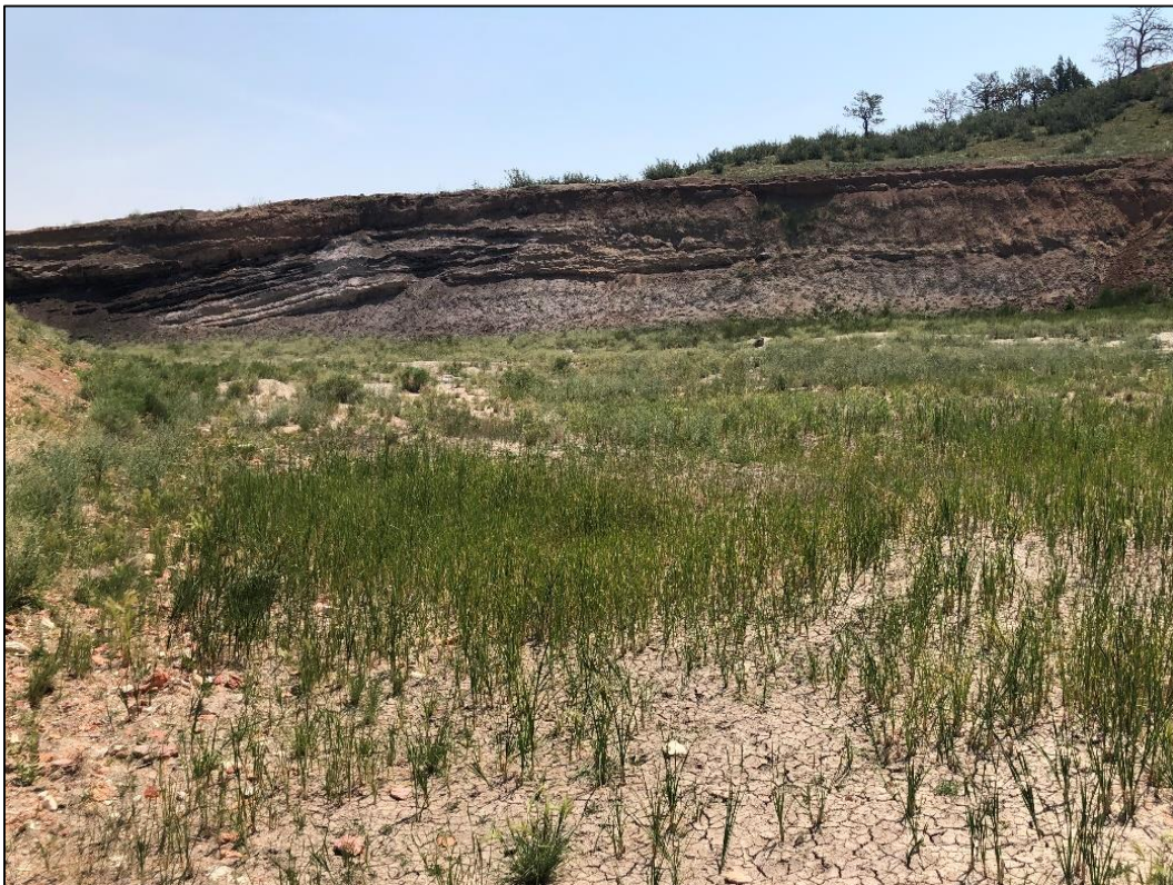
Photo 16. View looking east at eastern highwall of East pit, approximately 15-20 feet in height with near vertical to 1H:1V slopes.
