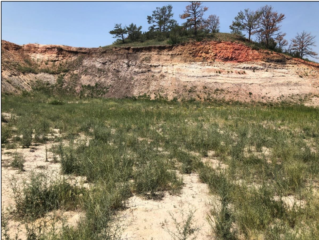
Photo 14. View looking west at western highwall of East pit, approximately 25 feet in height with near vertical slopes.
