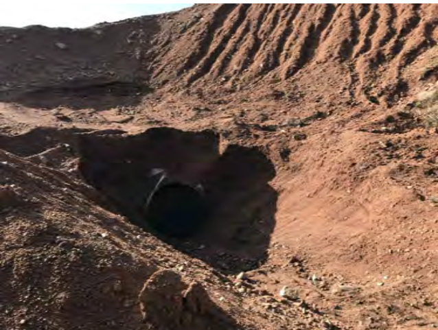
1. CULVERT PARTIALLY CLEARED, LIGHT COMING THROUGH
