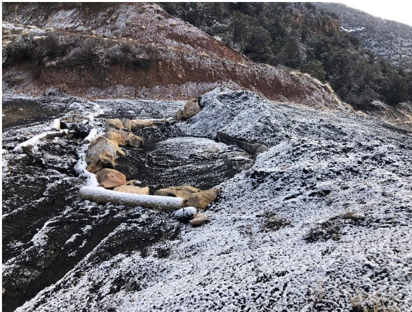
Sediment trap on Gob Pile #2
