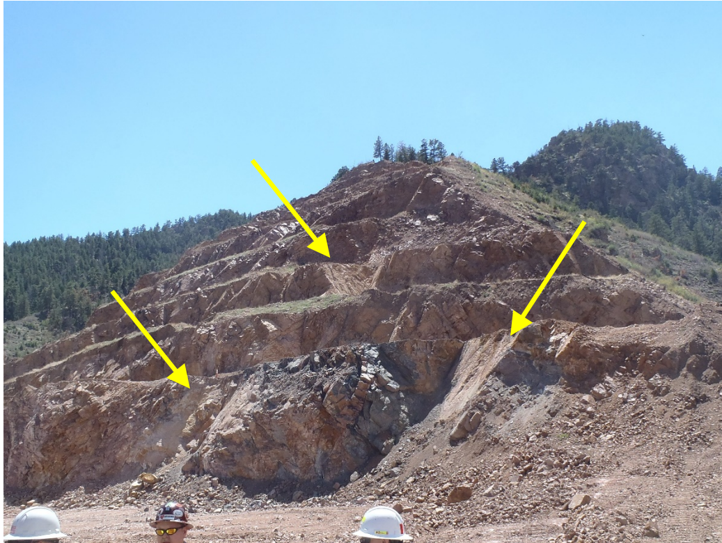
Photo 4. Evidence of larger block movement/slides (looking SW at west highwall).
