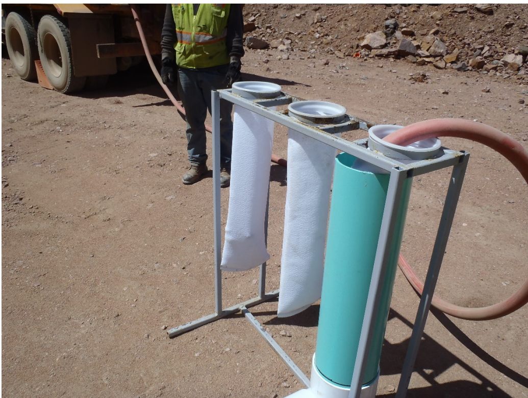
Photo 9. Filter socks for sediment pond water discharge demonstration.
