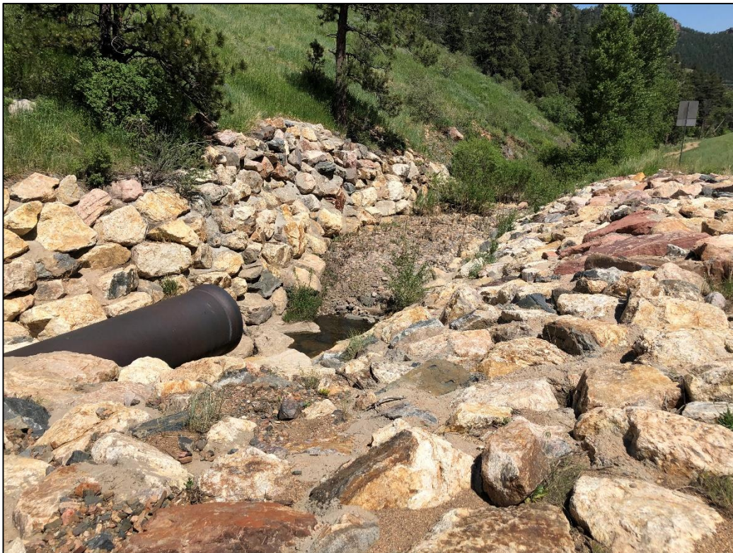
Photo 10. View looking downstream from upgradient cutoff wall in Ralston Creek, showing creek channel dry downstream of cutoff wall during site visit.
