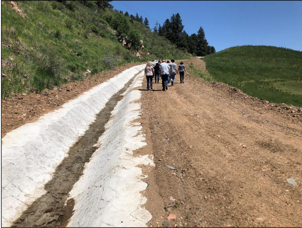
Photo 5. View looking upgradient at diversion channel installed along northern edge of North Waste Rock Pile (NWRP). Construction of this channel was completed in November of 2020.
