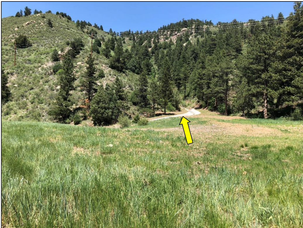
Photo 6. View looking east/northeast across top of NWRP. Note portion of diversion channel visible in background (indicated).
