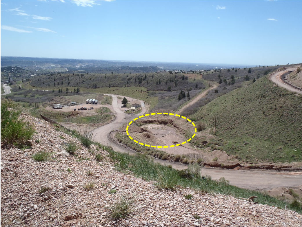
Photo 5. Sediment pond 514 (TR-07 designation) likely to need maintenance soon.
