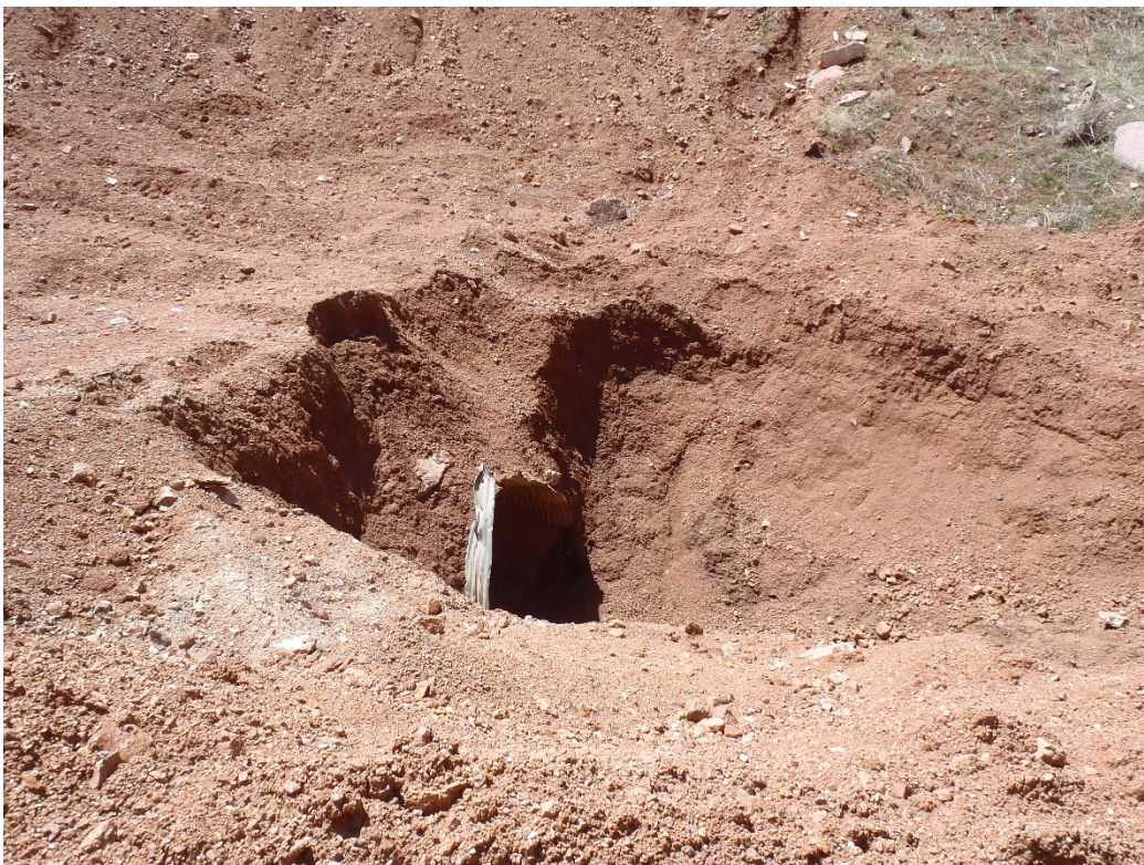
Photo 6. Partially unblocked northwest culvert.
