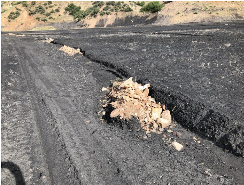
Check dams on Gob Pile #2 (in need of repair)
