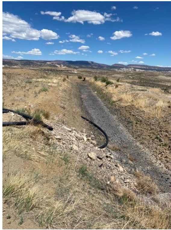
Photo 2: The inlet of the first cell of the B Seam No. 2 Dewatering System.
