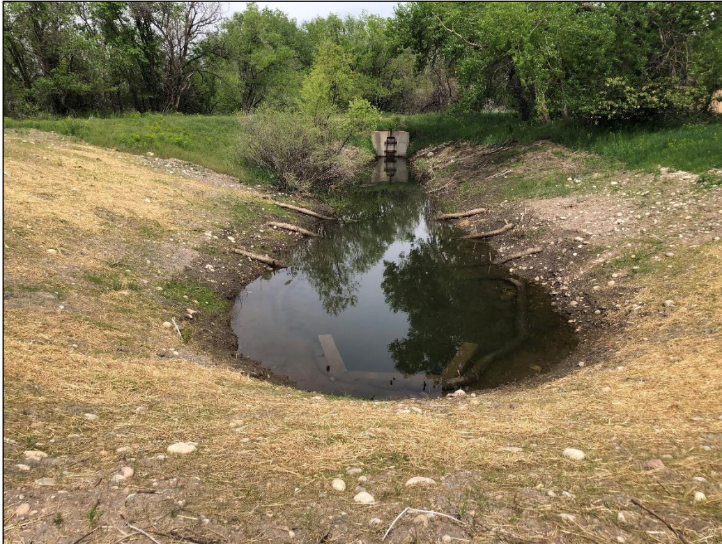
Photo 17. View looking northeast at outlet structure recently installed at northeastern edge of South Reservoir. The reclamation plan and map need to be updated to address any permanent water management structures installed on the affected lands.
