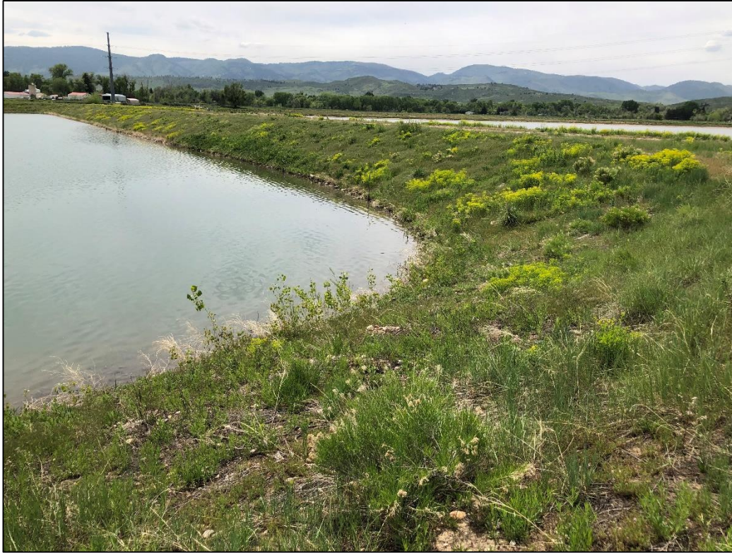
Photo 5. View looking west at western shoreline of South Reservoir, graded 3H:1V or flatter and stable with good vegetative cover. Operator will need to implement weed control plan in this area for state-listed noxious weed species.
