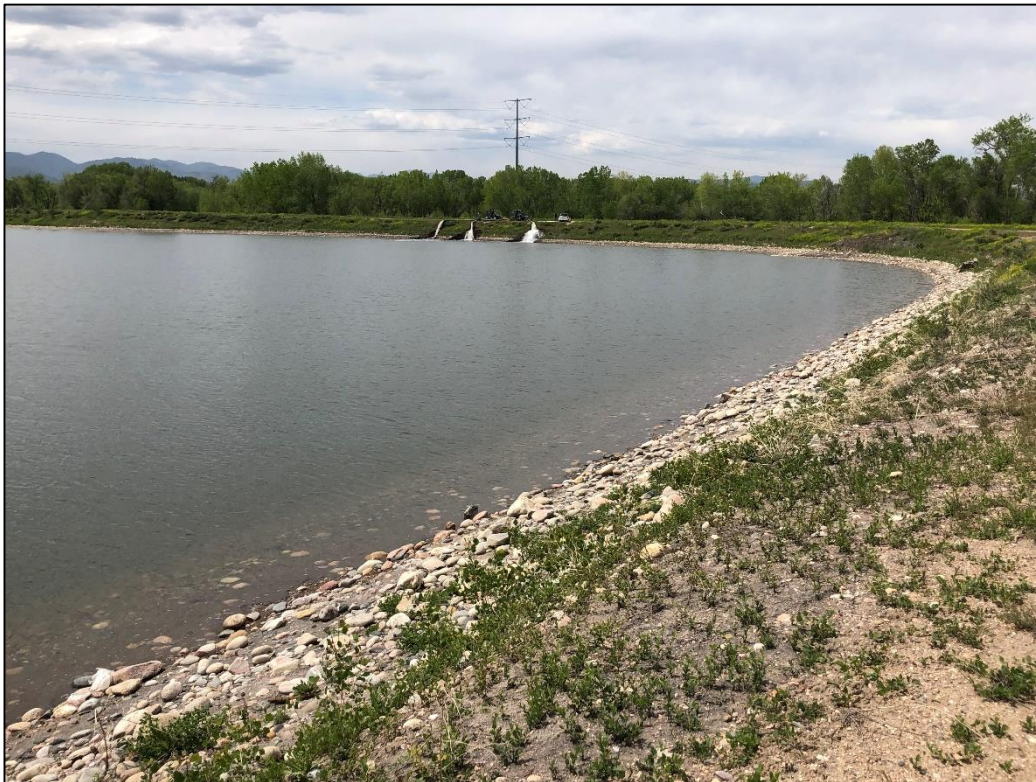
Photo 22. View looking northwest across eastern shoreline of North Reservoir, graded mostly 3H:1V or flatter with very sparse vegetative cover consisting primarily of volunteer cottonwood trees. Operator will need to remove trees, repair any erosion rilling, and reseed shoreline as needed. Weed control must also be implemented in this area for state-listed noxious weed species.
