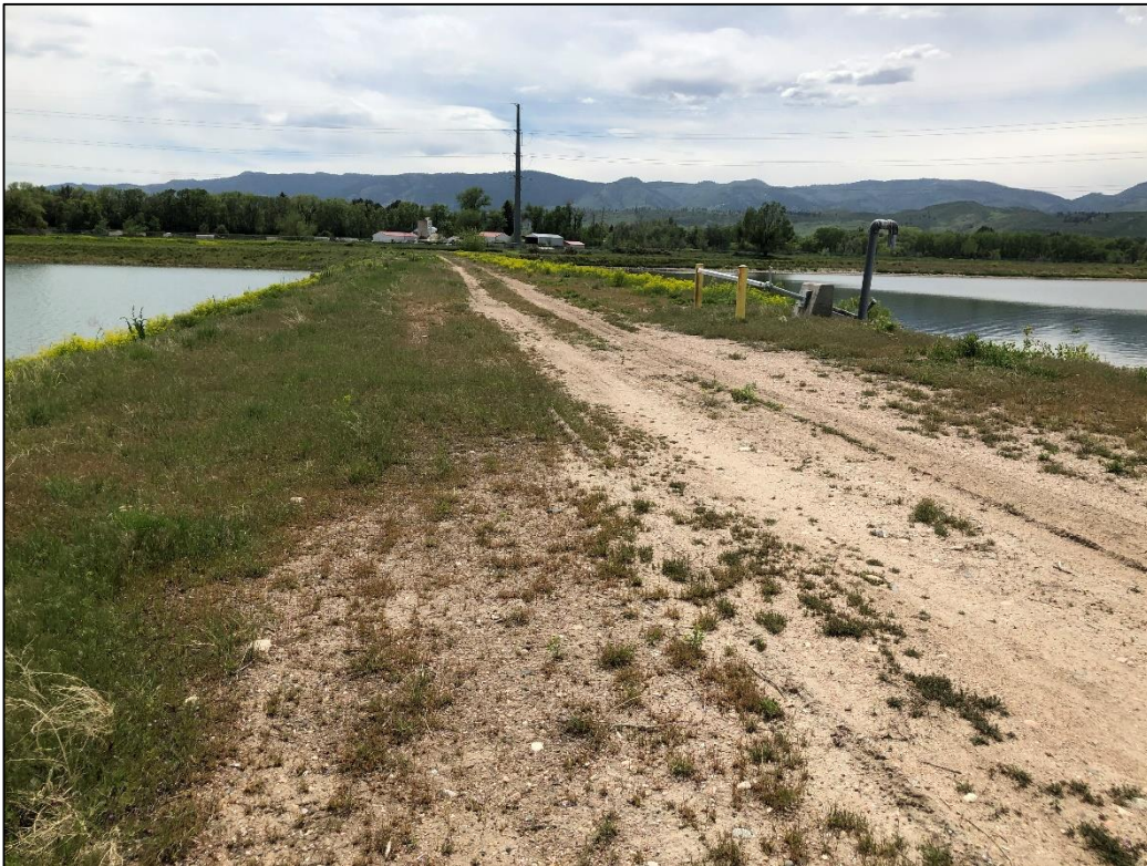
Photo 8. View looking southwest across land separating the two reservoirs. According to the operator, two interconnect pipelines are installed in this area. The reclamation plan and map need to be updated to address any permanent water management structures installed on the affected lands.
