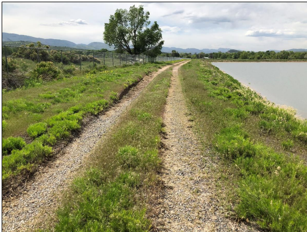
Photo 28. View looking northwest at dirt road along southern edge of North Reservoir which will remain for reclamation. Note fencing at left which delineates southern permit boundary.
