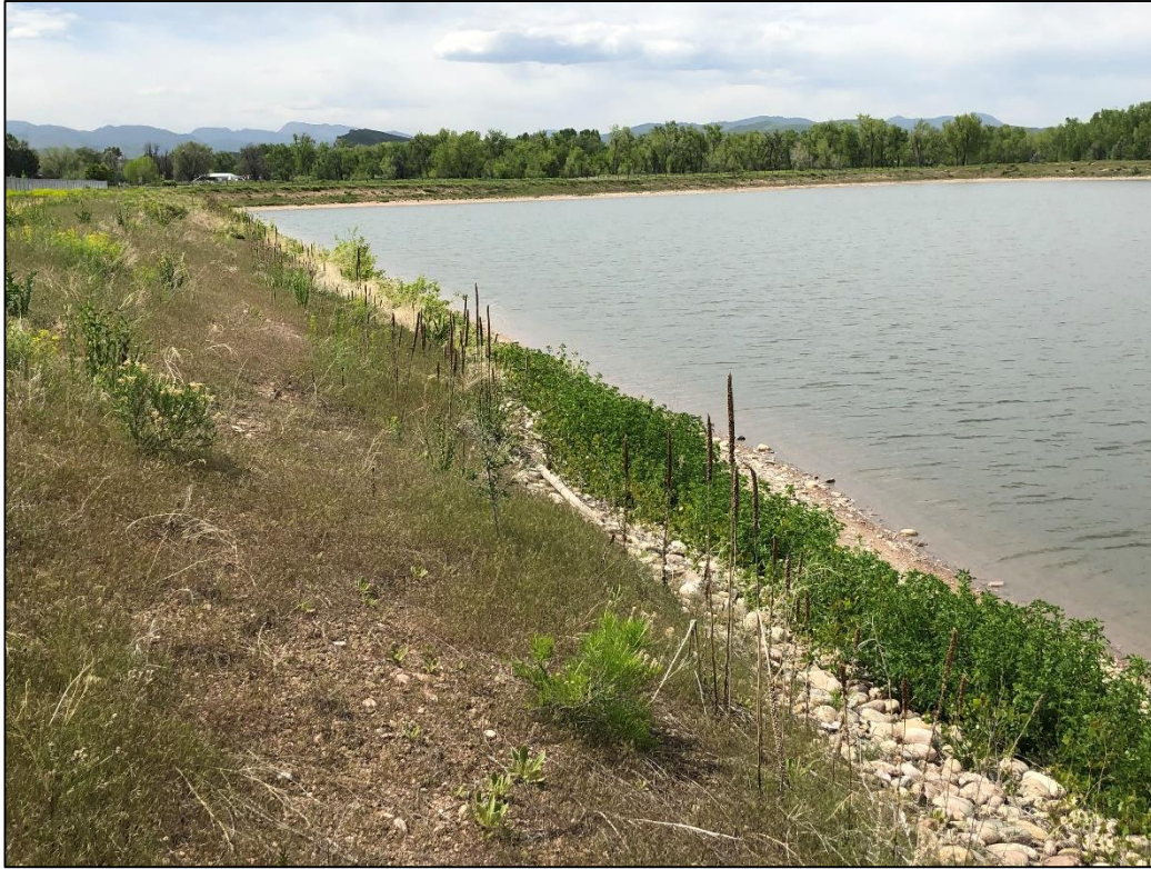
Photo 31. View looking northwest across southwestern shoreline of North Reservoir, graded mostly 3H:1V or flatter with dense cluster of volunteer cottonwood trees. Operator will need to remove trees, repair any erosion rilling, and reseed shoreline as needed. Weed control must also be implemented in this area for state-listed noxious weed species.
