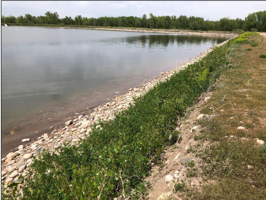
Photo 25. View looking northeast across southeastern shoreline of North Reservoir, graded mostly 3H:1V or flatter with dense cluster of volunteer cottonwood trees. Operator will need to remove trees, repair any erosion rilling, and reseed shoreline as needed. Weed control must also be implemented in this area for state-listed noxious weed species.
