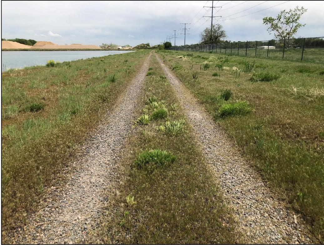
Photo 11. View looking southeast at dirt road along southern edge of South Reservoir which will remain for reclamation. Note fencing at right which delineates southern permit boundary.
