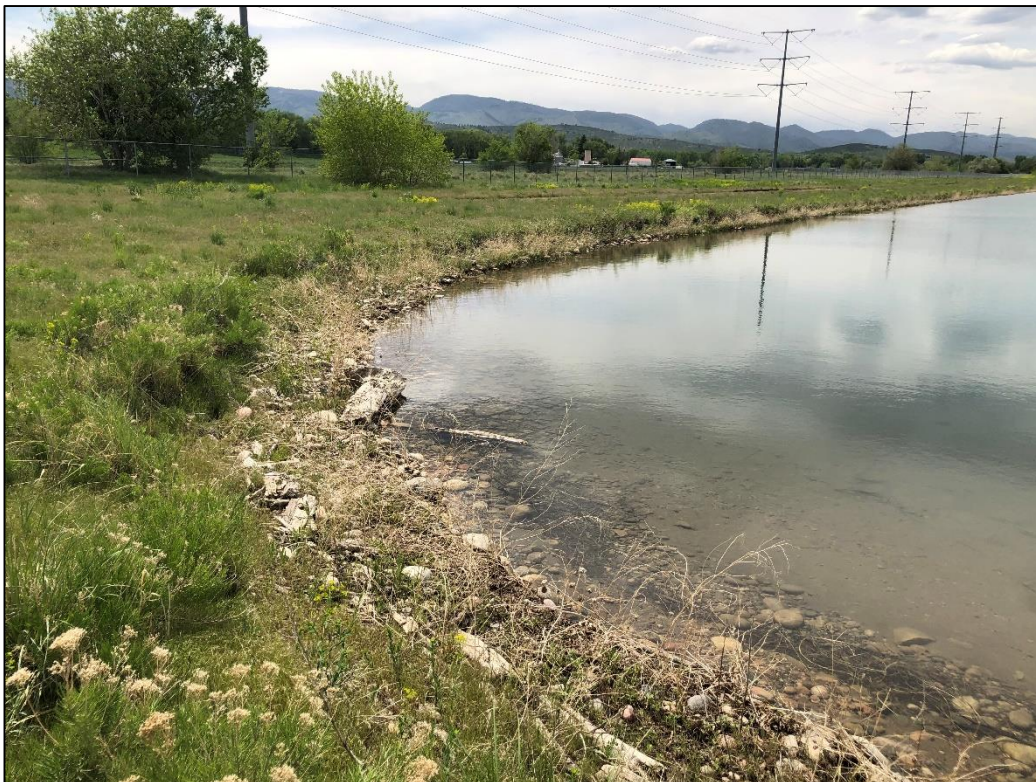
Photo 12. View looking west across southeastern shoreline of South Reservoir, graded 3H:1V or flatter and stable with good vegetative cover. Operator will need to implement weed control plan in this area for state-listed noxious weed species.
