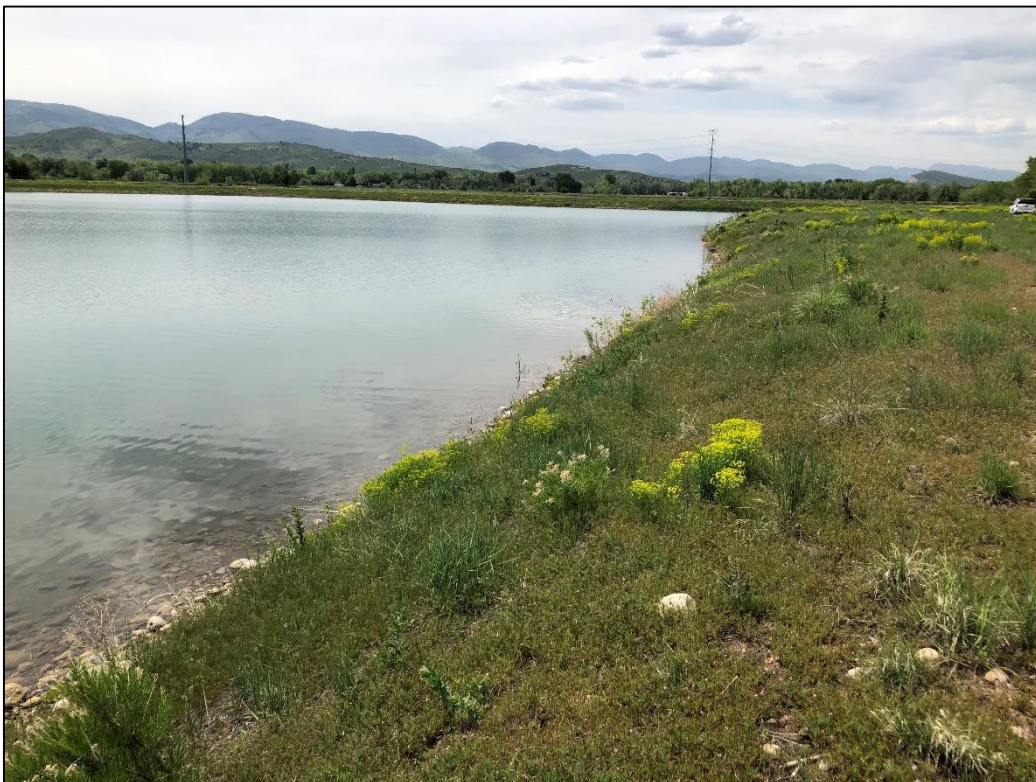
Photo 2. View looking northwest across northern shoreline of South Reservoir, graded 3H:1V or flatter and stable with good vegetative cover. Operator will need to implement weed control plan in this area for state-listed noxious weed species.
