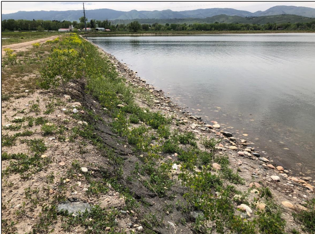
Photo 20. View looking southwest across southeastern shoreline of North Reservoir, graded mostly 3H:1V or flatter with very sparse vegetative cover consisting primarily of volunteer cottonwood trees. Operator will need to remove trees, repair any erosion rilling, and reseed shoreline as needed. Weed control must also be implemented in this area for state-listed noxious weed species.
