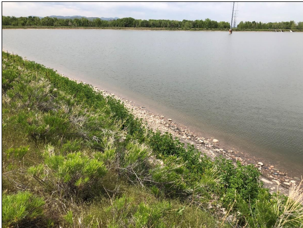
Photo 30. View looking northwest across southwestern shoreline of North Reservoir, graded mostly 3H:1V or flatter with dense cluster of volunteer cottonwood trees. Operator will need to remove trees, repair any erosion rilling, and reseed shoreline as needed. Weed control must also be implemented in this area for state-listed noxious weed species.
