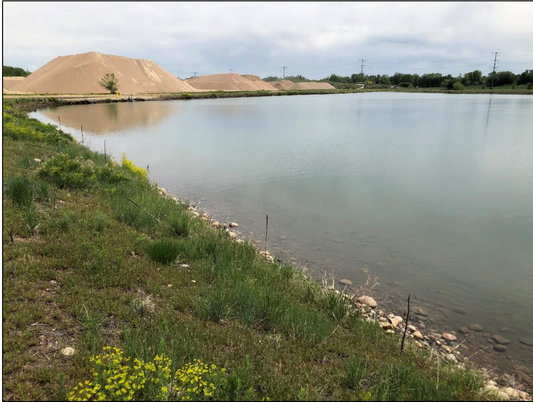
Photo 3. View looking southeast across northern shoreline of South Reservoir, graded 3H:1V or flatter and stable with good vegetative cover. Operator will need to implement weed control plan in this area for state-listed noxious weed species. Large material stockpiles visible in background are part of adjacent Home Office Mine permit.
