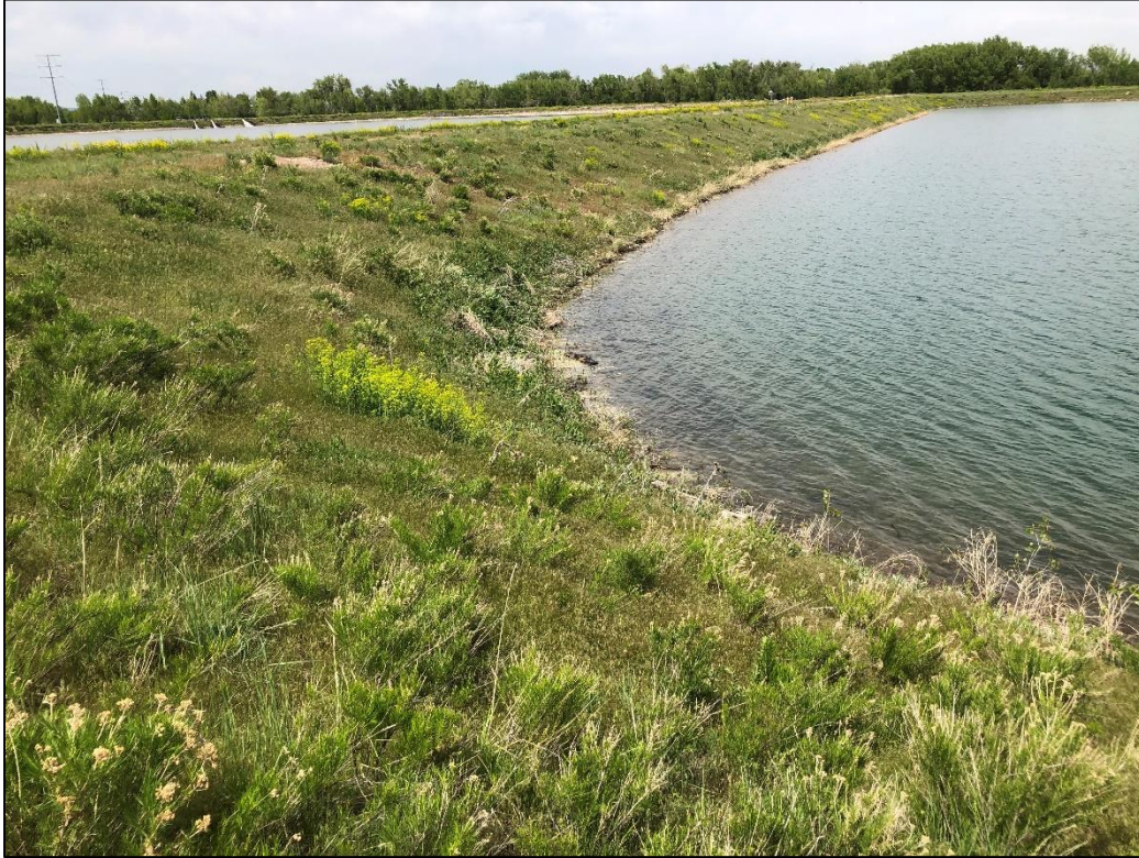
Photo 9. View looking northeast across western shoreline of South Reservoir, graded 3H:1V or flatter and stable with good vegetative cover. Operator will need to implement weed control plan in this area for state-listed noxious weed species.
