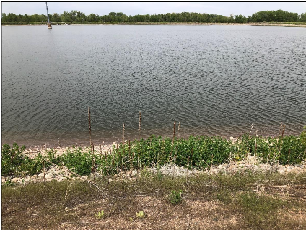
Photo 32. View looking northeast across North Reservoir from its southwestern shoreline. Operator will need to remove trees, repair any erosion rilling, and reseed shoreline as needed. Weed control must also be implemented in this area for state-listed noxious weed species.
