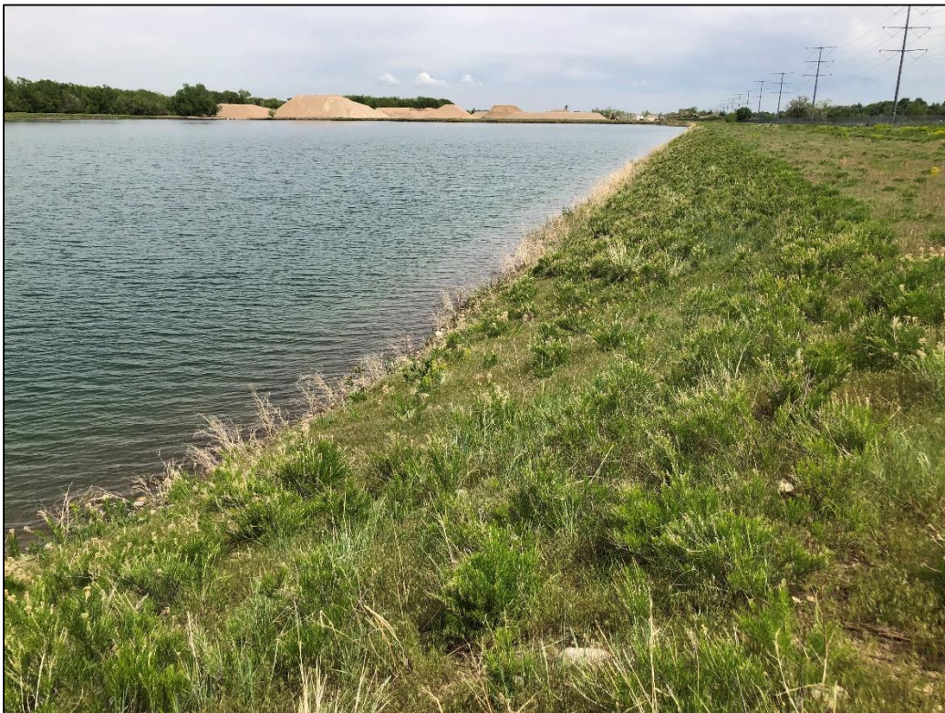
Photo 10. View looking southeast across southern shoreline of South Reservoir, graded 3H:1V or flatter and stable with good vegetative cover. Operator will need to implement weed control plan in this area for state-listed noxious weed species.
