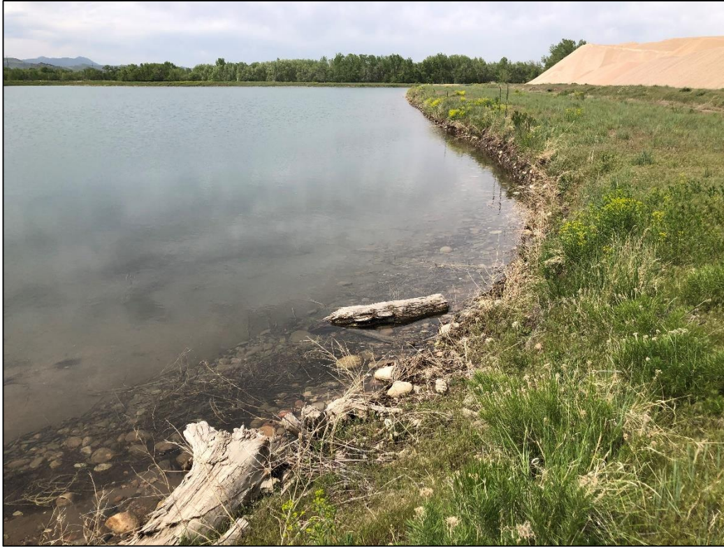
Photo 13. View looking north across eastern shoreline of South Reservoir, graded 3H:1V or flatter and stable with good vegetative cover. Operator will need to implement weed control plan in this area for state-listed noxious weed species.
