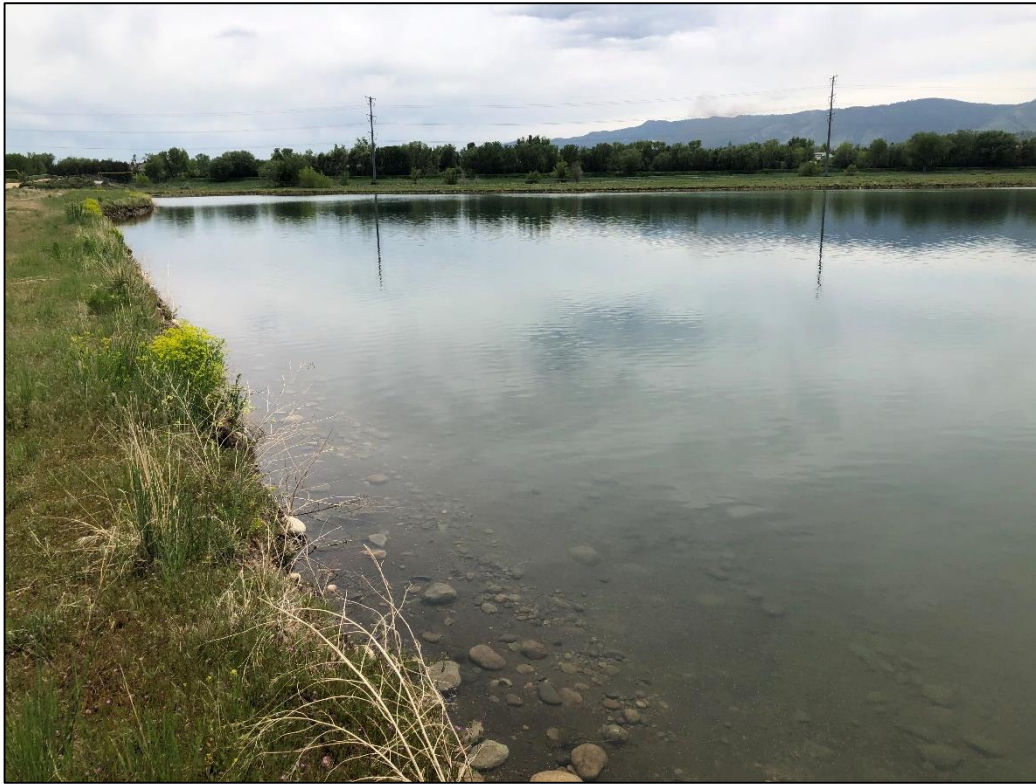
Photo 1. View looking south across eastern shoreline of South Reservoir, graded 3H:1V or flatter and stable with good vegetative cover. Operator will need to implement weed control plan in this area for state-listed noxious weed species.
