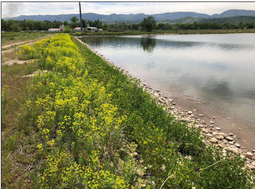
Photo 26. View looking southwest across southeastern shoreline of North Reservoir, graded mostly 3H:1V or flatter with dense cluster of volunteer cottonwood trees. Operator will need to remove trees, repair any erosion rilling, and reseed shoreline as needed. Weed control must also be implemented in this area for state-listed noxious weed species.
