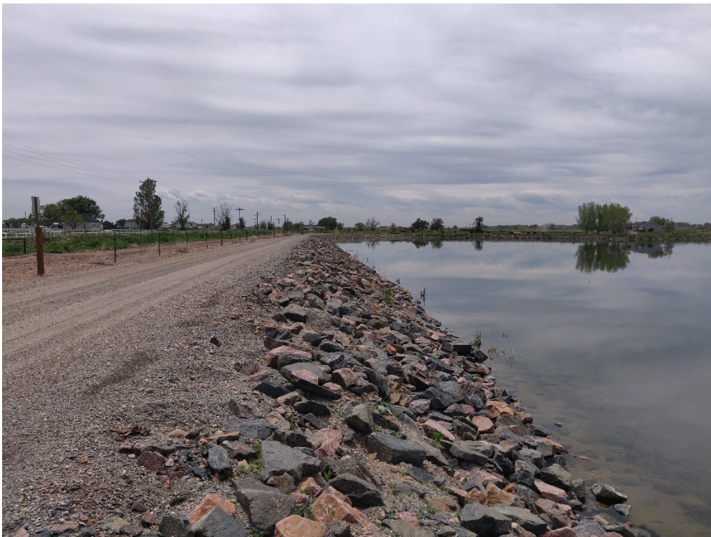
View of the riprapped eastern shoreline looking south
