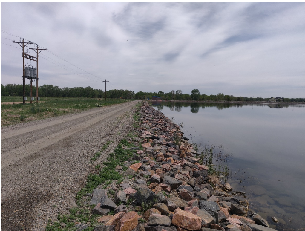
View of riprapped northern shoreline looking east
