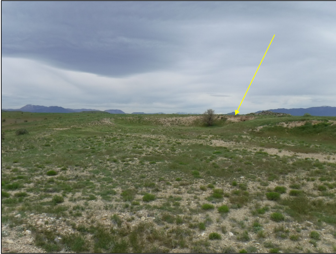
Photo 3: Looking west across the pit area from the east side, yellow arrow indicates highwall are needing grading, the tamarisk tree will also require removal
