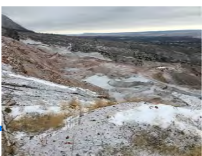
4. FILL DEPOSITED AT TOE OF SLIDE AREA
