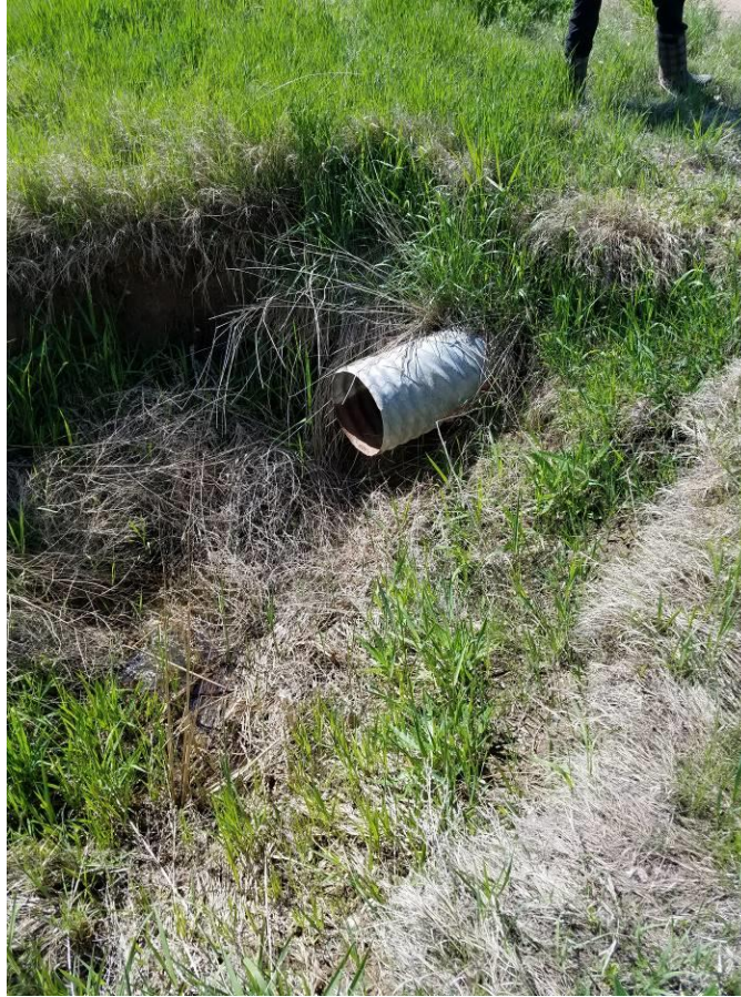
Figure 9. Culvert from the Cell No. 4 area to the Big Thompson River.
