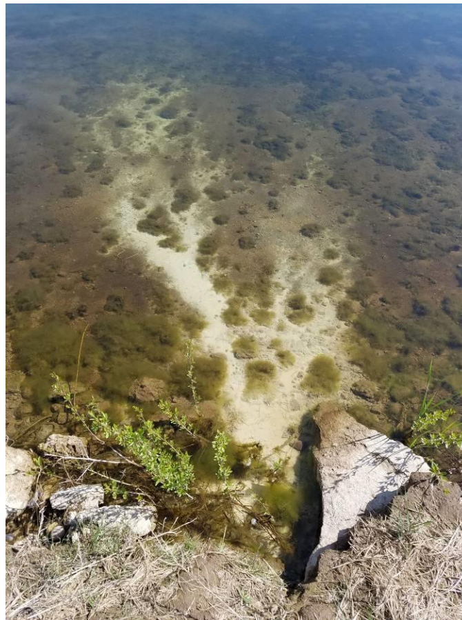
Figure 6. "White Spot" along southern shore where water is likely seeping in from the adjacent wetland through the concrete rip-rap depositing fine sediment.
