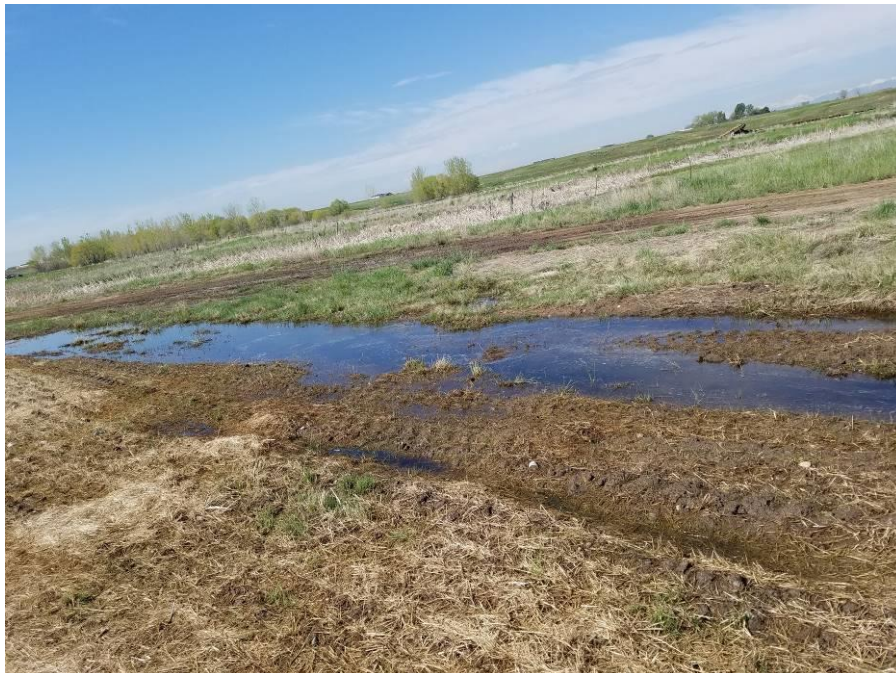
Figure 2. "Sink Hole" or depression near the northwest corner of the site.
