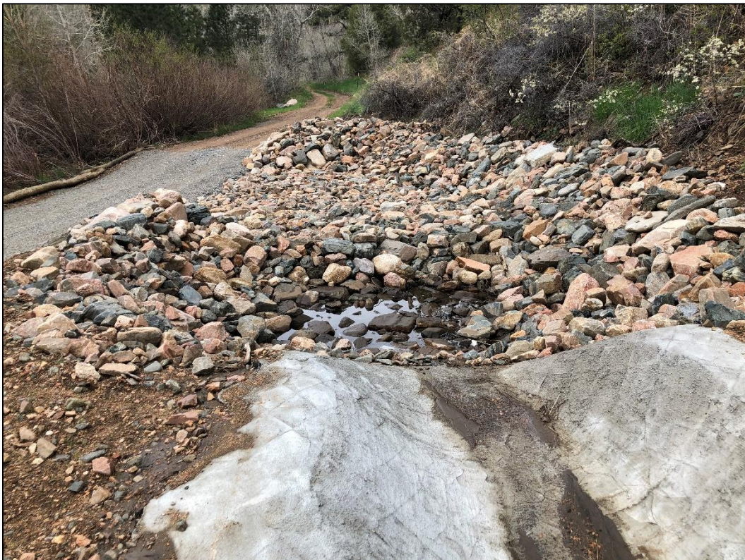
Photo 14. View looking west/northwest at riprap-lined energy dissipation basin constructed at downgradient end of NWRP diversion channel, showing some water ponded in basin during inspection.
