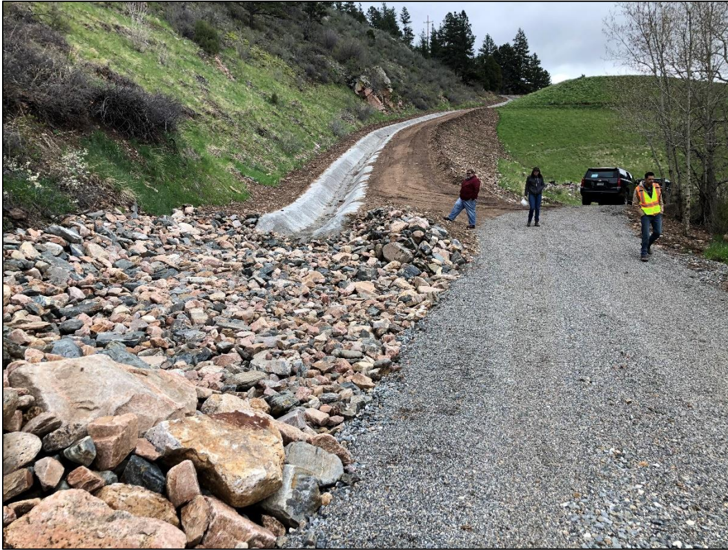
Photo 13. View looking east/southeast at riprap-lined energy dissipation basin (at left) constructed at downgradient end of NWRP diversion channel and road crossing (at right) constructed of gravel-filled Geoweb system.
