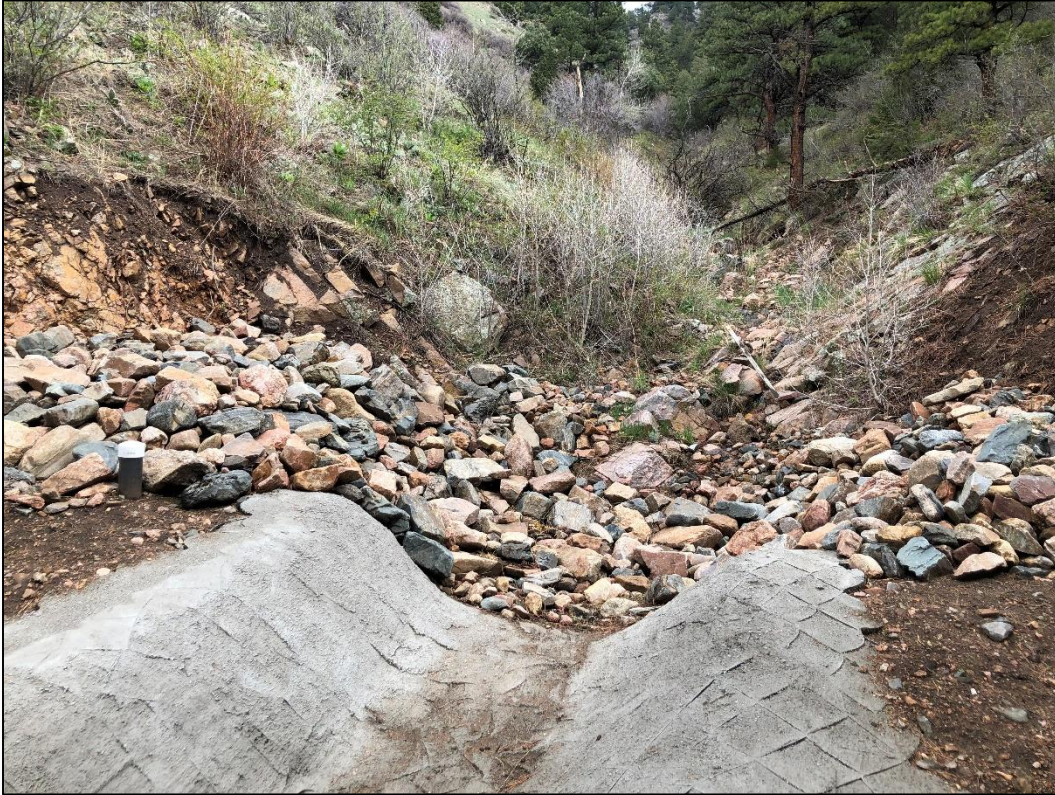
Photo 11. View looking north/northeast at riprap-lined water intake structure constructed at upgradient end of NWRP diversion channel in ephemeral drainage above pile.
