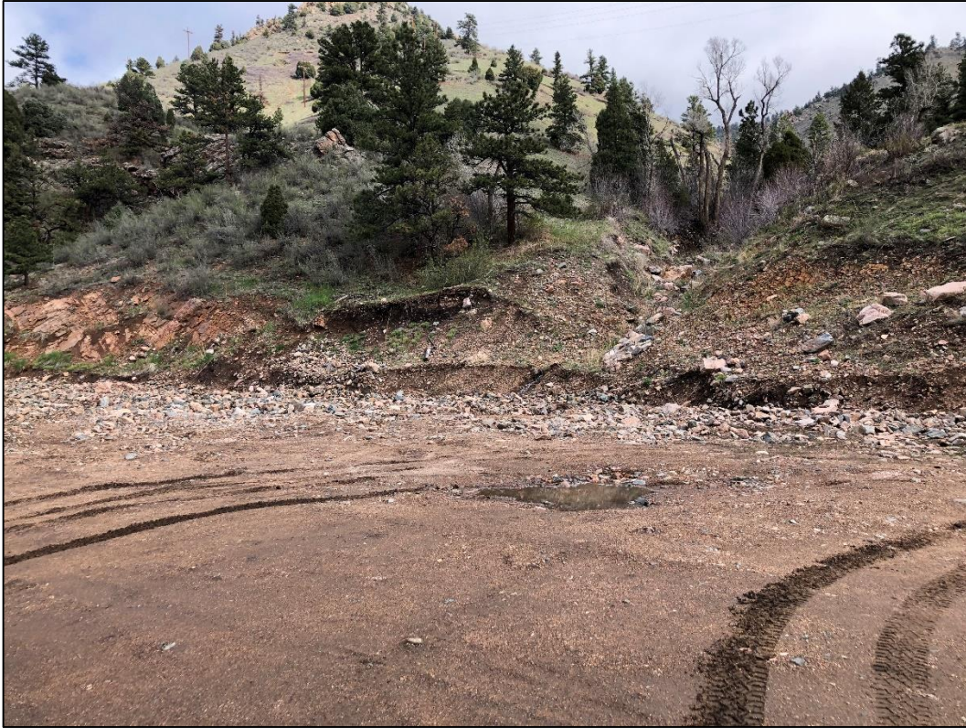
Photo 15. View looking north across borrow area located up valley from NWRP where rock and fill material was excavated from flood deposit for diversion channel project. Mining activities have ceased in this area and reclamation will be completed under operator's USACE permit.
