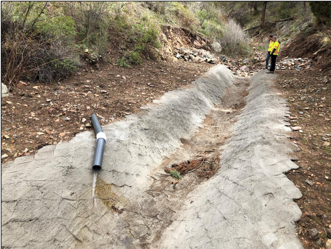
Photo 10. View looking north/northeast (upgradient) at upper section of NWRP diversion channel, showing pipeline from water intake structure which daylights to discharge into channel approx. 50 feet downgradient from seal wall. Note water flowing from pipeline during inspection (at estimated 5 gpm).
