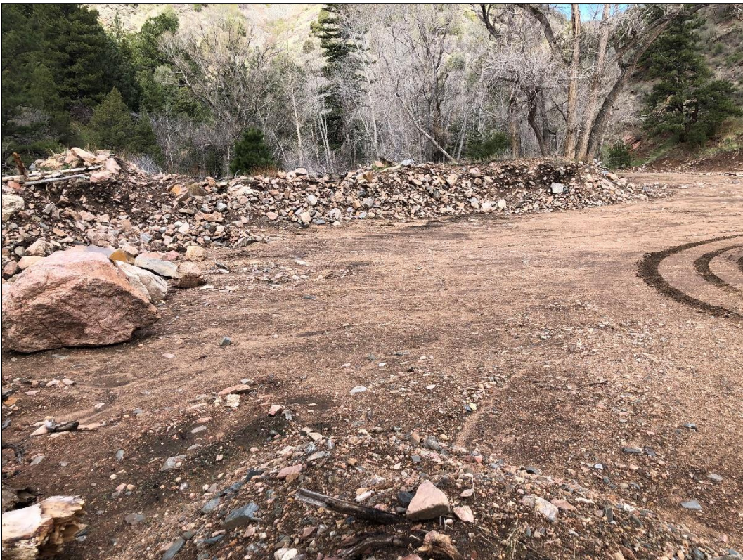
Photo 16. View looking south across borrow area located up valley from NWRP where rock and fill material was excavated from flood deposit for diversion channel project. Mining activities have ceased in this area and reclamation will be completed under operator's USACE permit.
