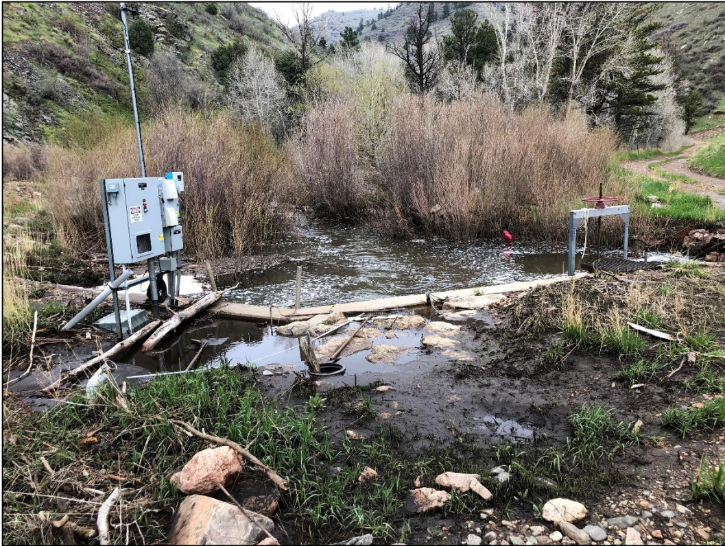
Photo 7. View looking upstream at upgradient cutoff wall/headgate in Ralston Creek. Note creek running high upstream from cutoff wall and standing water present in area during inspection.
