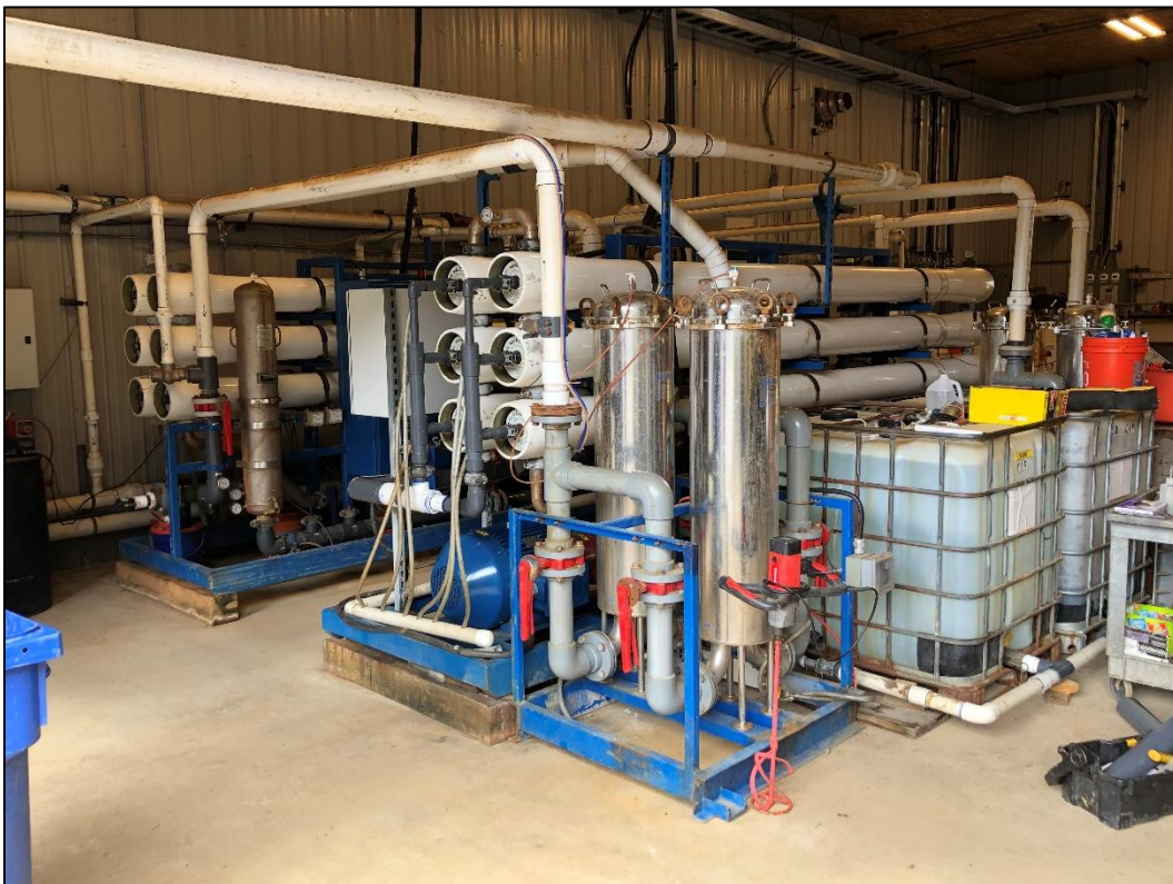
Photo 2. View of Reverse Osmosis System present inside water treatment plant.
