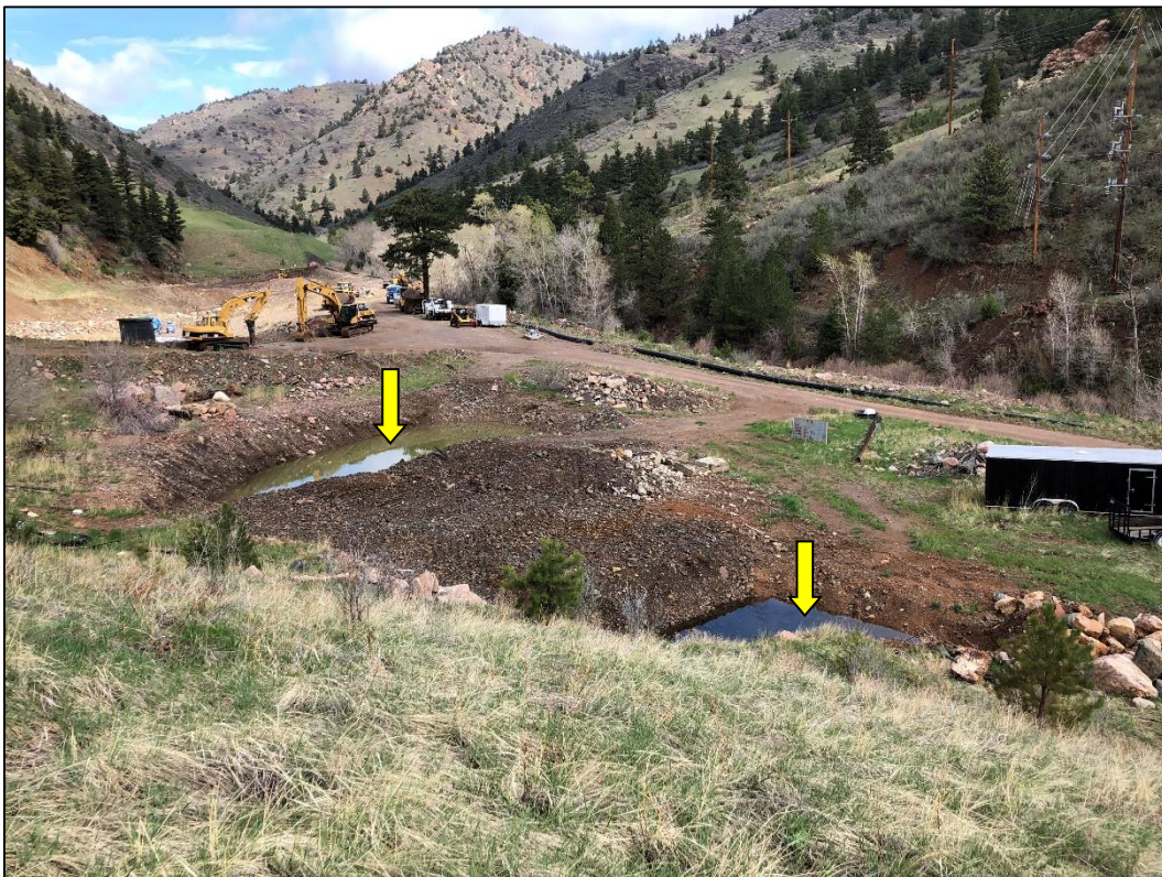
Photo 4. View looking northwest from top of mesa across valley excavation project area. Note standing water in excavated pits (indicated) from recent storm events. This water will be pumped to plant for treatment (if needed) and ultimately discharged at operator's permitted outfall.
