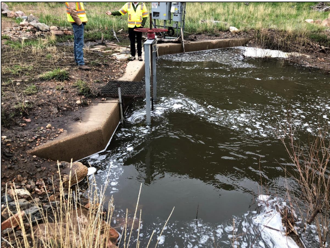
Photo 8. View looking south at upgradient cutoff wall/headgate in Ralston Creek, showing creek running high upstream of cutoff wall during inspection.
