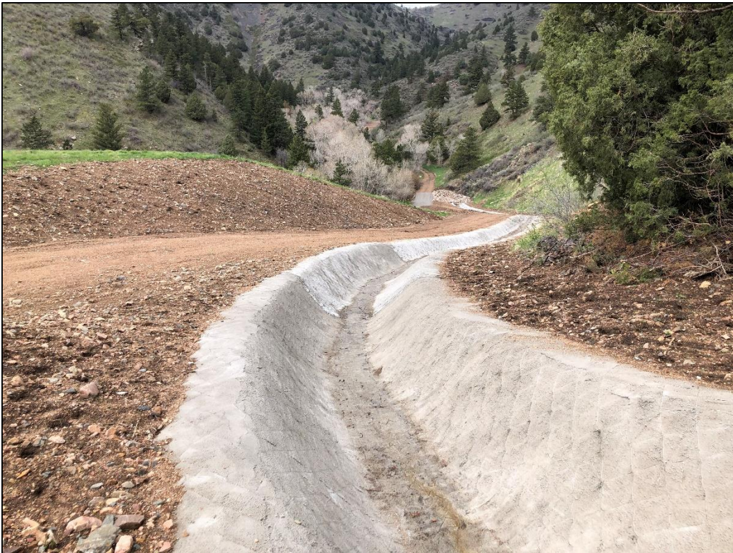
Photo 12. View looking southwest (downgradient) at section of NWRP diversion channel which curves around hillside. Note channel free of debris and functioning as designed.
