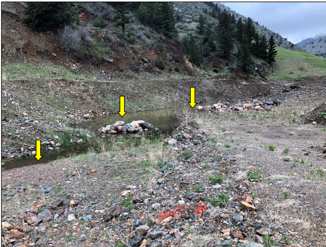
Photo 6. View looking northwest across central portion of valley excavation project area. Note standing water in excavated pit (indicated) from recent storm events. This water will be pumped to plant for treatment (if needed) and ultimately discharged at operator's permitted outfall.
