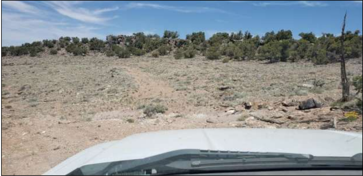
Figure 6: A gully eroded across the roadway. This will need to be filled in with rocks prior to crossing, and the drive-around blocked off. During reclamation, any fill should be removed, but the drive-around should be left. May be a good place for a large boulder in the road. 38.131742, -108.821510
