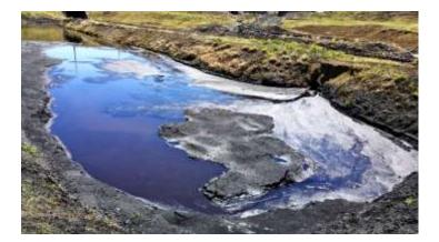
The oil waddles between the first and second pond have moved past the channel between the two cells (pictured below). These were determined to be necessary due to oil sheen that has been observed in the first cell, as pond B discharges directly to the creek. Please replace these or provide another solution. No oil sheen was observed during this inspection.
