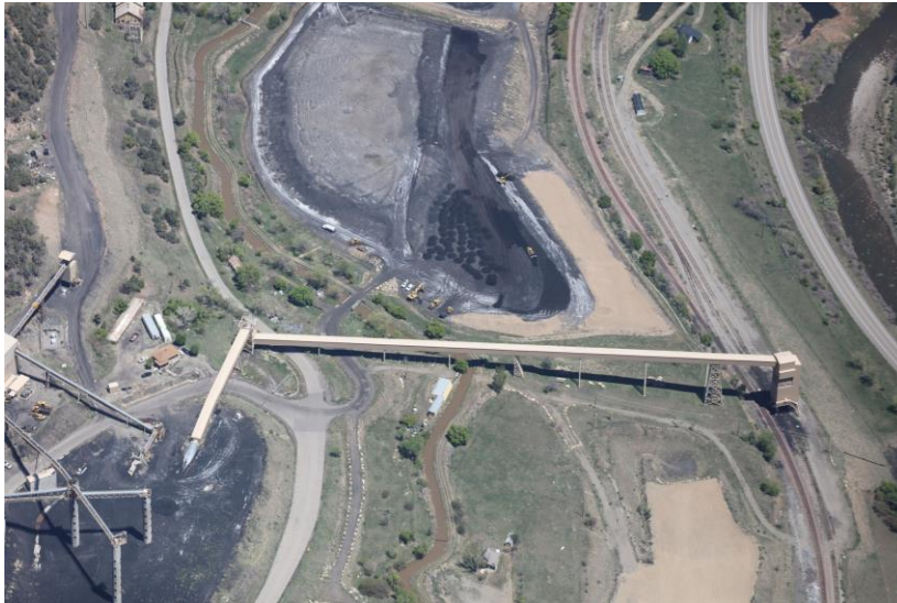
Gob Pile #3, lower conveyor, and Coal Stockpile Pad
