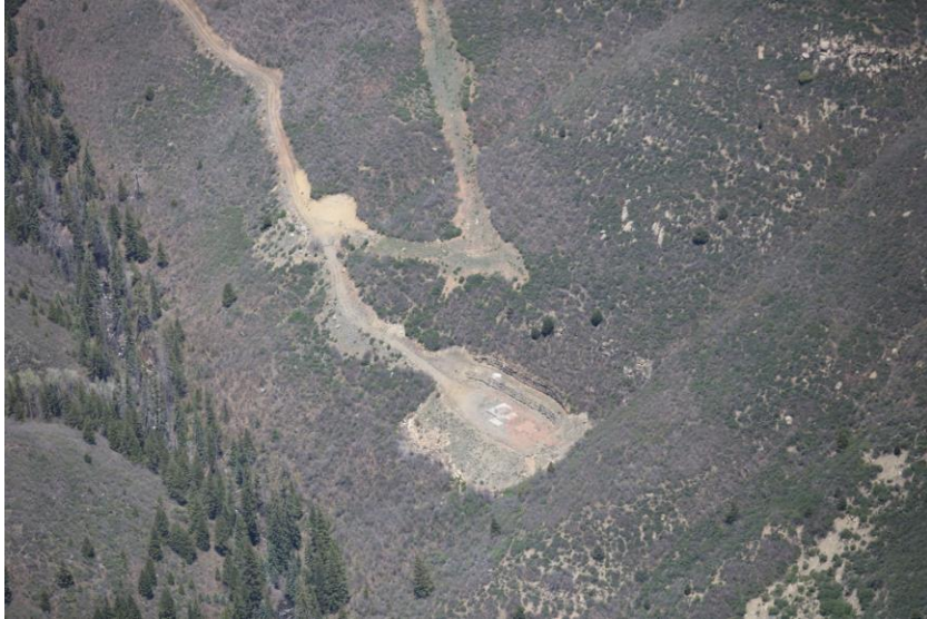
Pad for Terror Creek Vent Shaft
