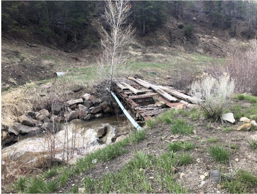
Pipe attached to bridge
