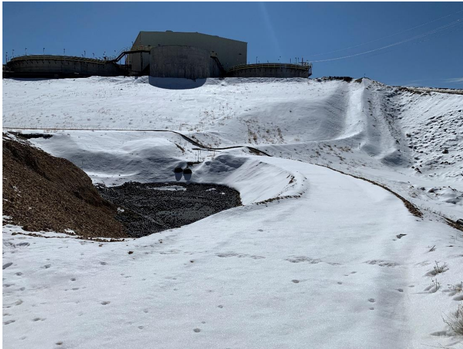
Photo 1 – PSES pond larger embankment
