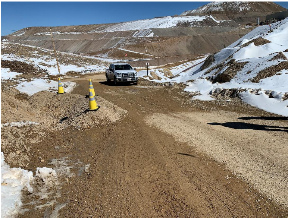
Photo 2 – Water bar and sump across the access road
