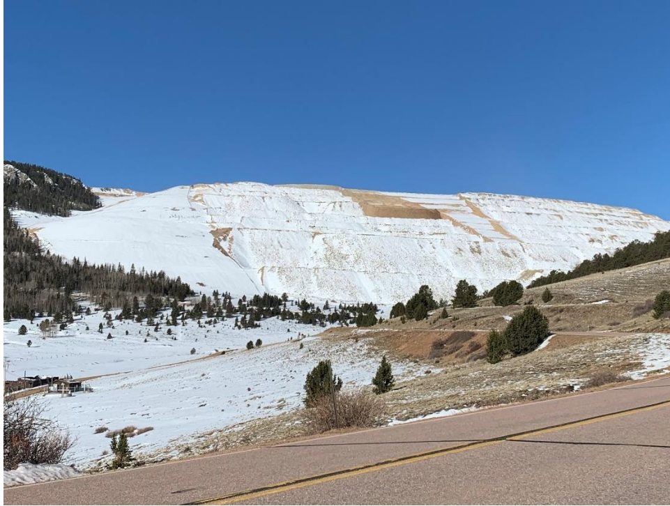
Photo 3 – Grading work on ECOSA
