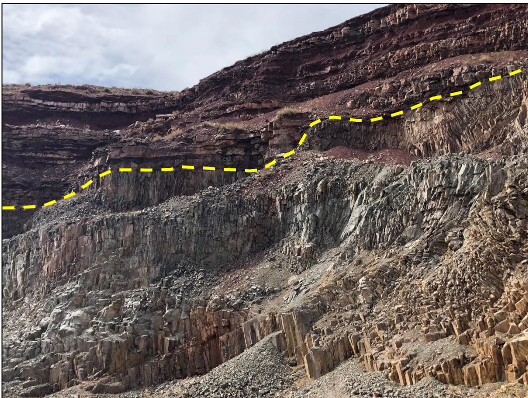
Photo 4. View looking south at Quarry 1, showing closer view of its western (northeast-facing) highwall. Note dacite rocks (lower half of highwall) are heavily fractured and dipping toward the quarry in some areas. The approximate contact between the lower dacite and the upper sedimentary rock units is delineated with a yellow dashed line.
