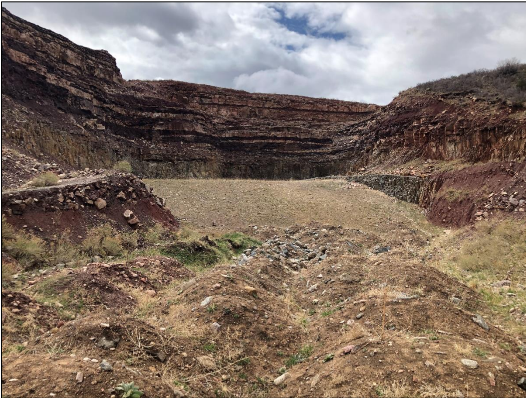
Photo 18. View looking southeast at Quarry 2, which was partially backfilled with imported material in 2017/2018. Highwalls above the backfill are approximately 100 feet tall with slope gradients ranging from near vertical (dacite) to 1.5H:1V (sedimentary overburden). Note majority of remaining highwalls consists of sedimentary overburden rocks.
