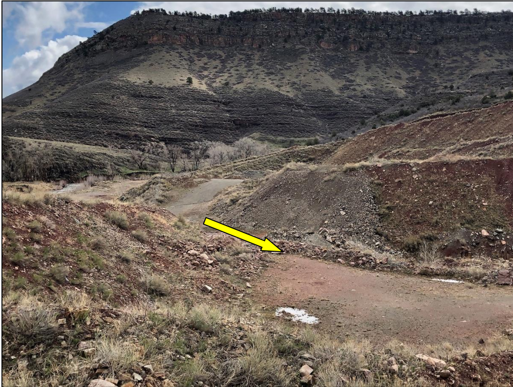
Photo 11. View looking east at Quarry 1, showing "swale"/quarry access (indicated with arrow) that exists between Quarry 1 backfill material on pit floor (at right) and Quarry 2 access ramp (at left). In TR-5, the operator proposes backfilling this "swale" to create a rockfall catchment berm.
