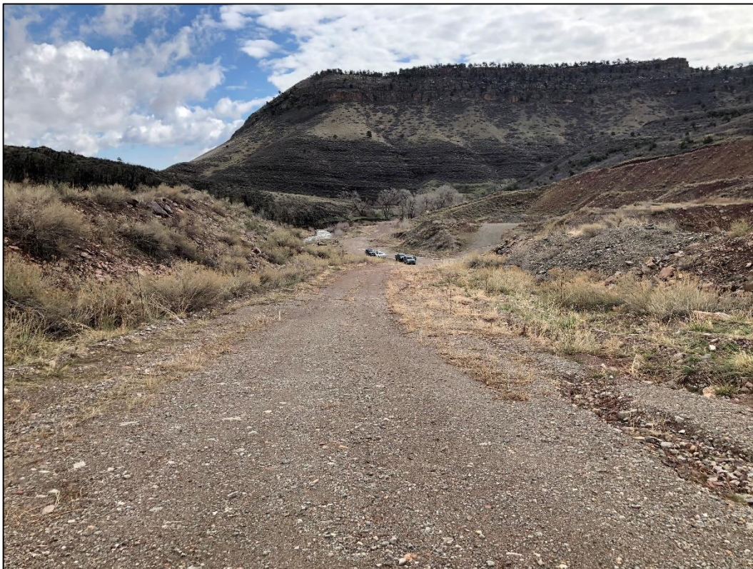
Photo 12. View looking east (toward Quarry 1) down road ramp constructed out of overburden material in early 2000's for Quarry 2 access.
