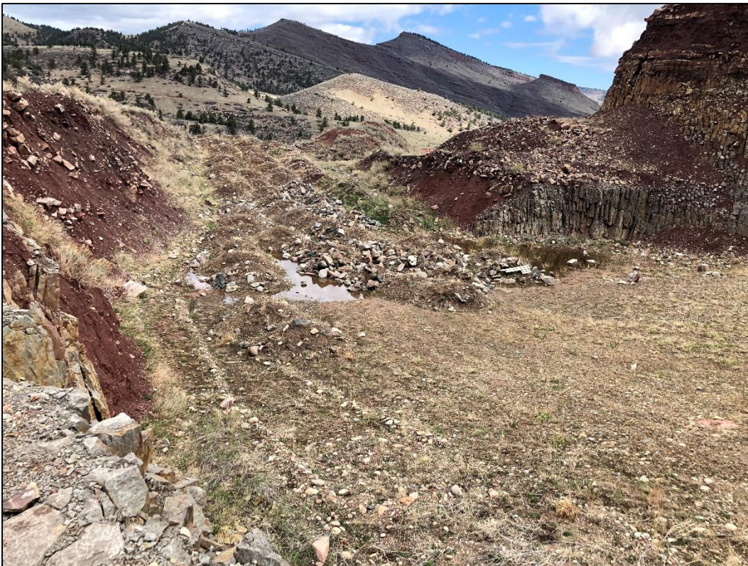
Photo 24. View looking north at Quarry 2 entrance (from inside quarry) where imported backfill material was placed in 2017/2018. Ponding shown in photo was from recent storm event.
