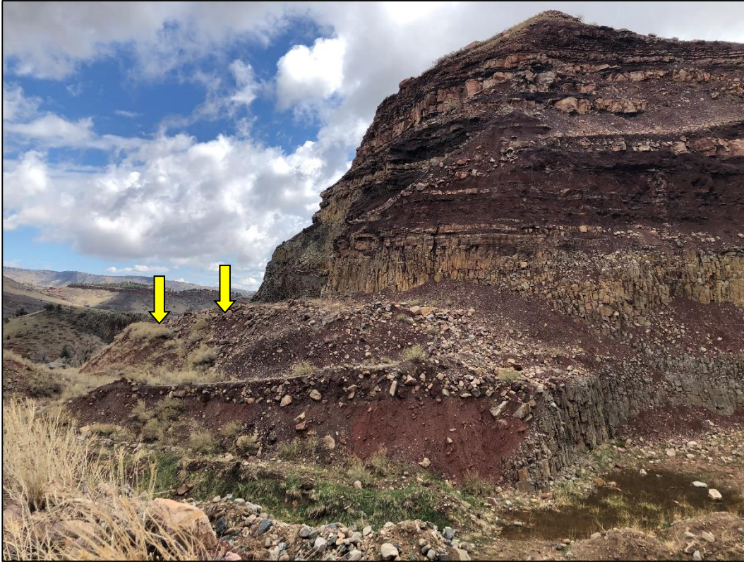
Photo 17. View looking east at western edge of northwest-facing highwall. In TR-5, the operator proposes constructing a rockfall catchment berm (for which space appears limited) and chain-link fencing along the top of the backfill area (indicated).
