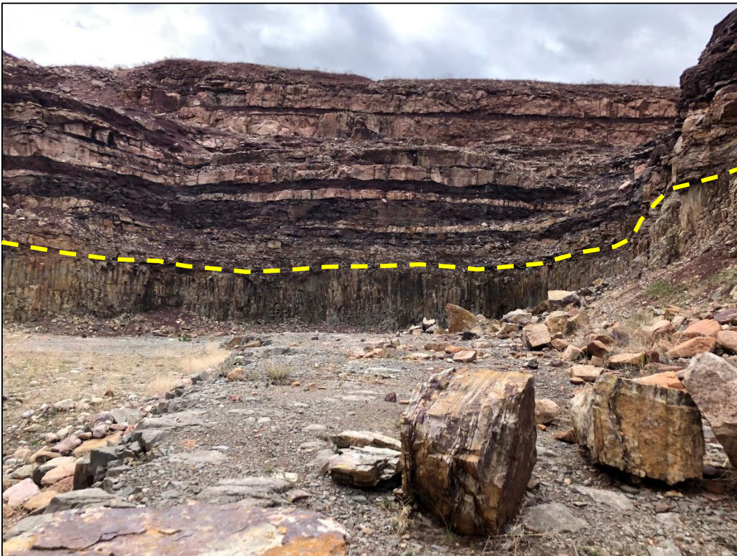
Photo 20. View looking southeast at Quarry 2, showing its southern (northwest-facing) highwall. The approximate contact between the lower dacite and the upper sedimentary rock units is delineated with a yellow dashed line. Note rocks in foreground which fell from western highwall. Larger boulders are derived from overburden sandstone unit.
