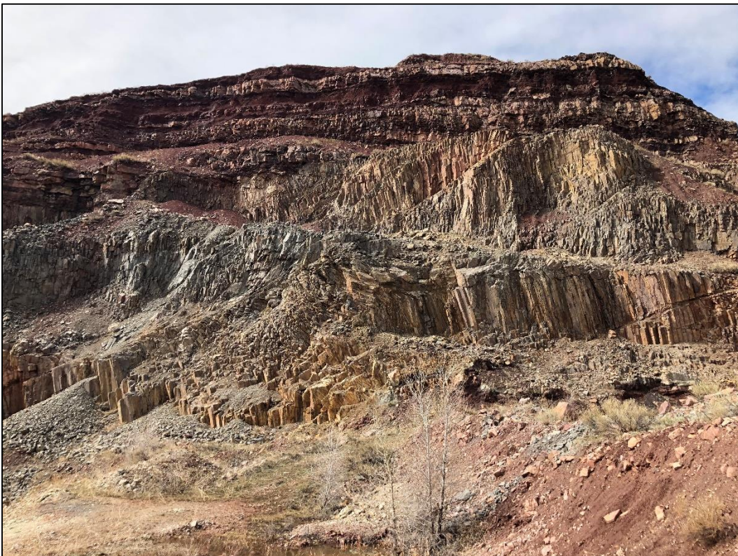
Photo 2. View looking south at Quarry 1, with approximately 300 foot tall highwalls and slope gradients ranging from near vertical (dacite) to 1.5H:1V (sedimentary overburden).
