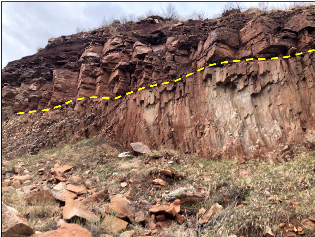
Photo 22. View looking southwest at Quarry 2, showing closer view of western (northeast-facing) highwall. Note dacite rocks (lower portion of highwall) are heavily fractured, and overburden sandstone rocks are overhanging the dacite. The approximate contact between the lower dacite and the upper sedimentary rock units is delineated with a yellow dashed line. Talus at foot of highwall includes rocks of various sizes, with larger boulders (up to 5 feet in length) typically derived from sandstone unit above dacite. Dacite rocks are typically smaller than 2 feet in length.
