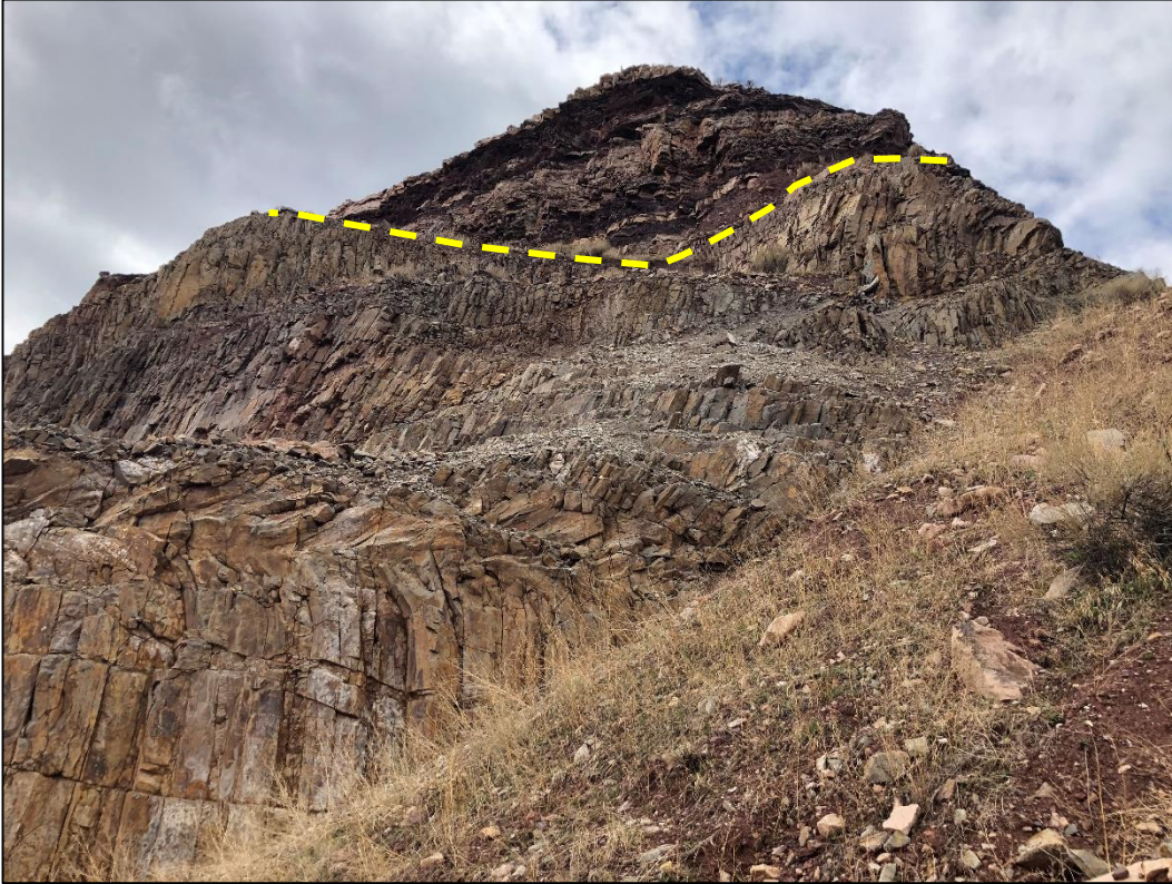
Photo 7. View looking south at Quarry 1, showing western edge of its northeast-facing highwall. Note dacite rocks (lower half of highwall) are heavily fractured but dip mainly away from the quarry in this area. The approximate contact between the lower dacite and the upper sedimentary rock units is delineated with a yellow dashed line.
