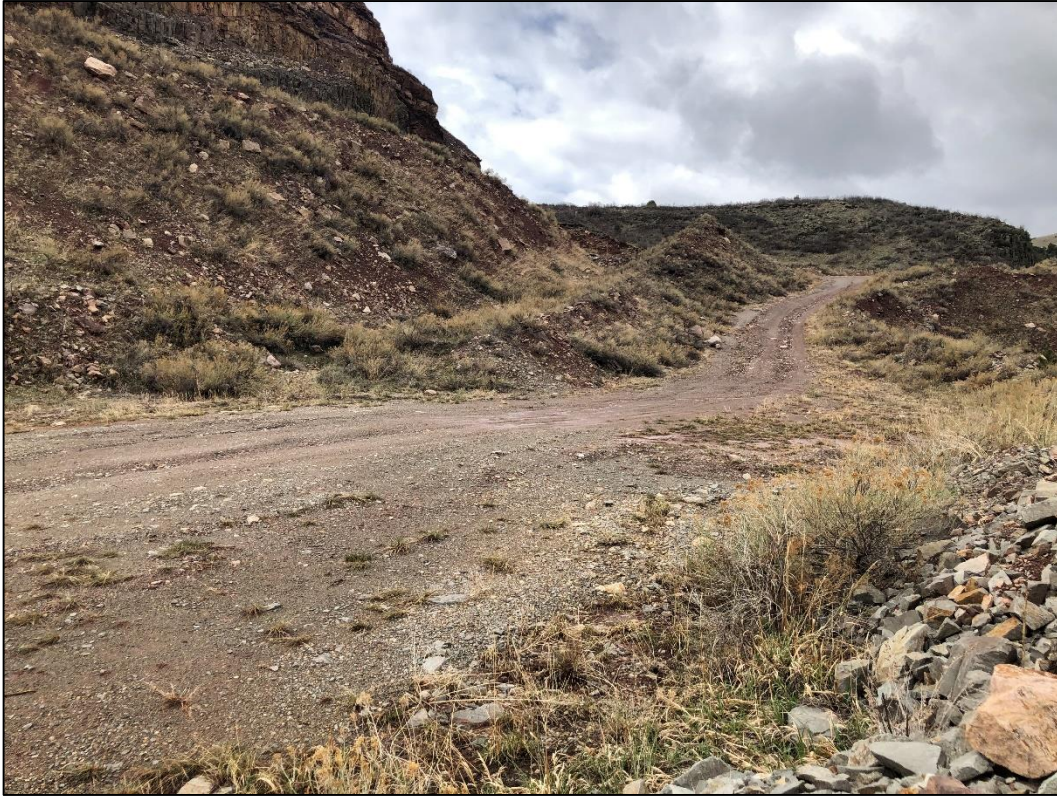
Photo 13. View looking west (toward Quarry 2) up road ramp constructed out of overburden material in early 2000's for Quarry 2 access.
