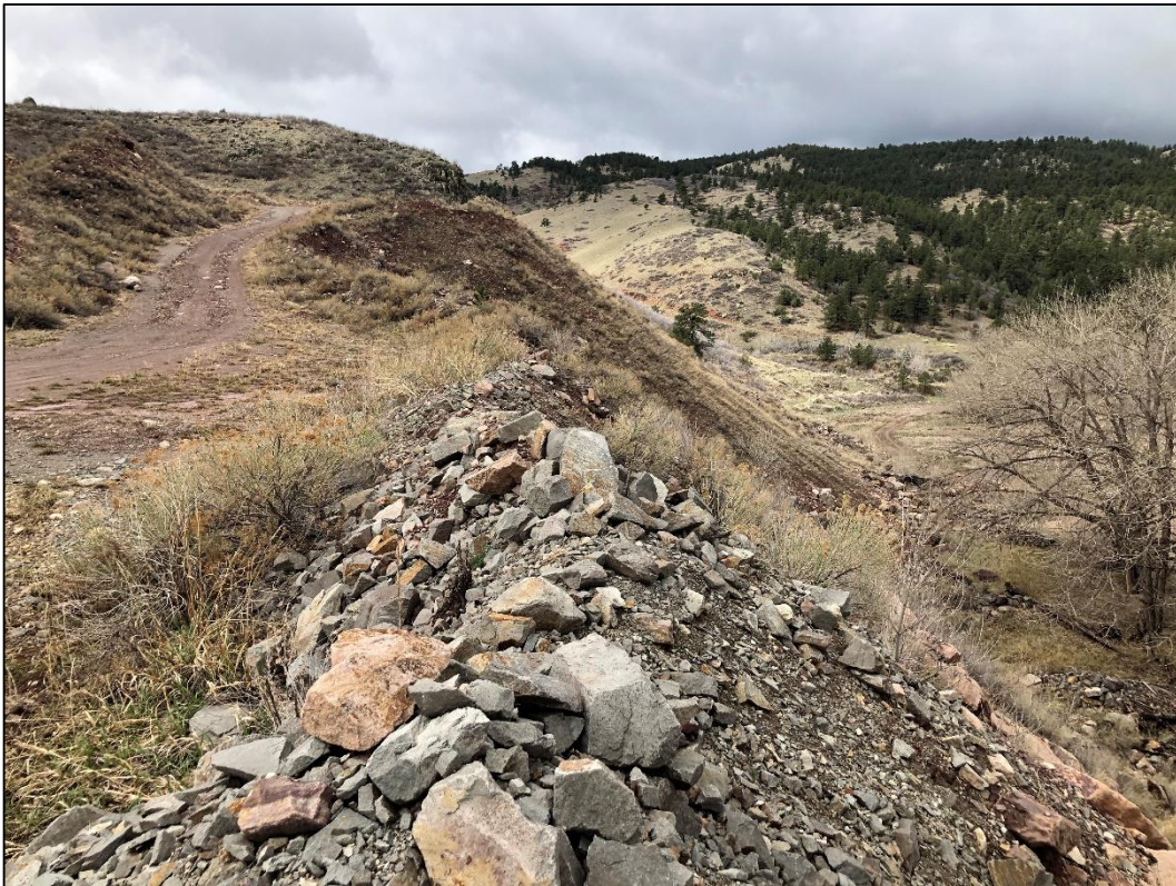
Photo 14. View looking west at northern side slope of road ramp constructed out of overburden material in early 2000's for Quarry 2 access, with slope gradients of approximately 1.5H:1V.
