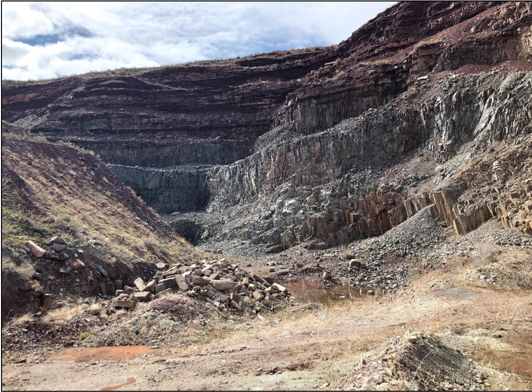
Photo 1. View looking southeast at Quarry 1, with approximately 300 foot tall highwalls and slope gradients ranging from near vertical (dacite) to 1.5H:1V (sedimentary overburden). Note western edge of Quarry 1 backfill visible at left edge of photo. Ponding shown in photo was from recent storm event.
