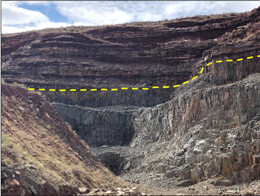
Photo 3. View looking southeast at Quarry 1, showing closer view of its eastern (north-facing) highwall. Note dacite rocks (lower half of highwall) are heavily fractured (making rock bolt use for stabilization challenging) and dipping toward the quarry in some areas. The approximate contact between the lower dacite and the upper sedimentary rock units is delineated with a yellow dashed line.
