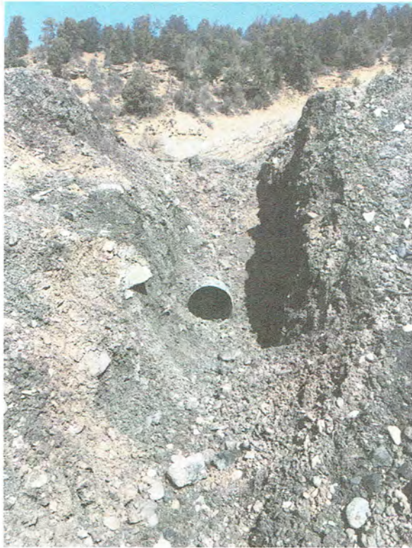
Pic. 3 – Culvert at new switchback with soil sloughing needing repair.
