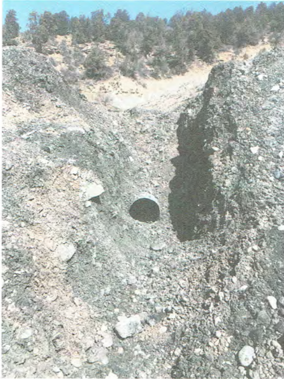
Pic. 5 – New switchback culvert with soil sloughing (downstream end).
