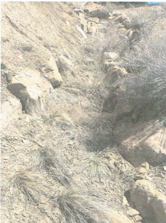
Pic. 6 –Clean water ditch (Reach 1) with sediment.
