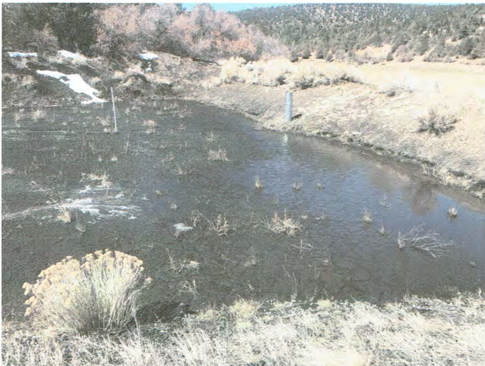
Pic. 2 – West pond sediment gage appears near the required maintenance mark.
