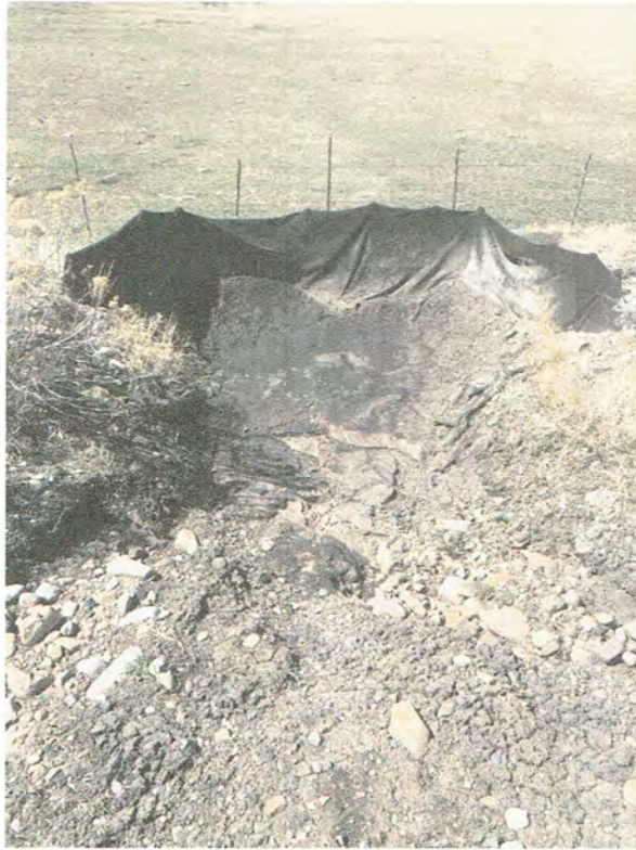
Pic. 3 – Sediment trap at driveway.
