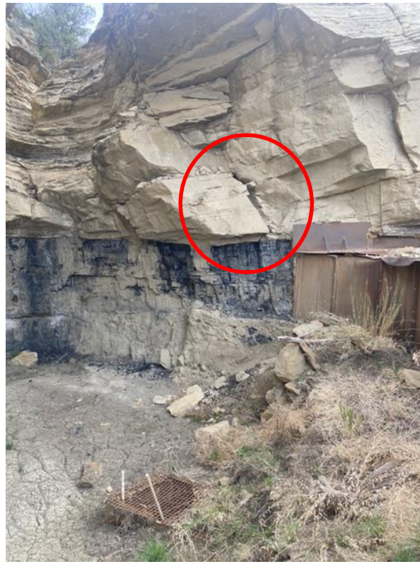
Photo 3: The eastern sump at the portals bench. The large crack in the bedrock above the sump is identified in a red circle.
