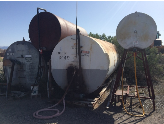
Inproper Fuel Storage- secondary containment
