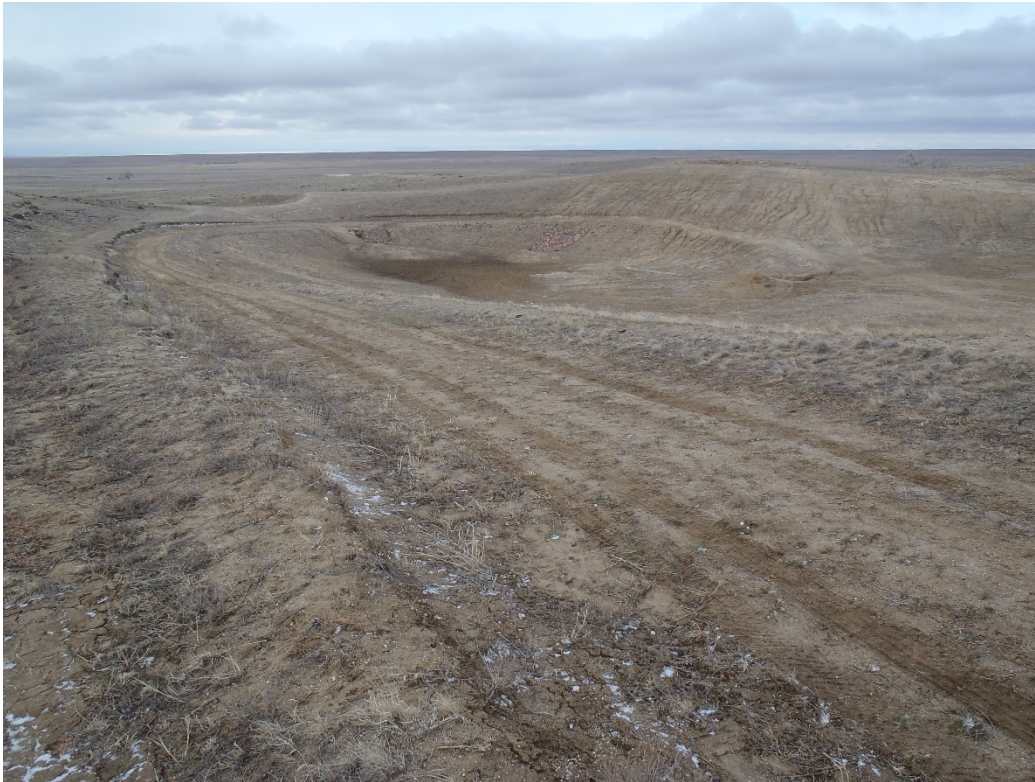
Photo 2. Access road into pit and graded slopes: \leq 3H:1V (looking south).
