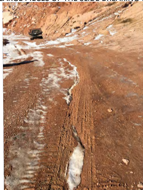
2. RECENT CRACKING LIKELY FROM SETTLEMENT
