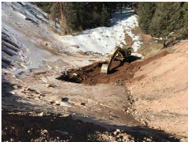
1. AREA UPSTREAM OF CULVERT GETTING CLEARED OF DEBRIS
