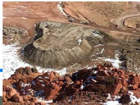
4. FILL DEPOSITED AT TOE OF SLIDE AREA
