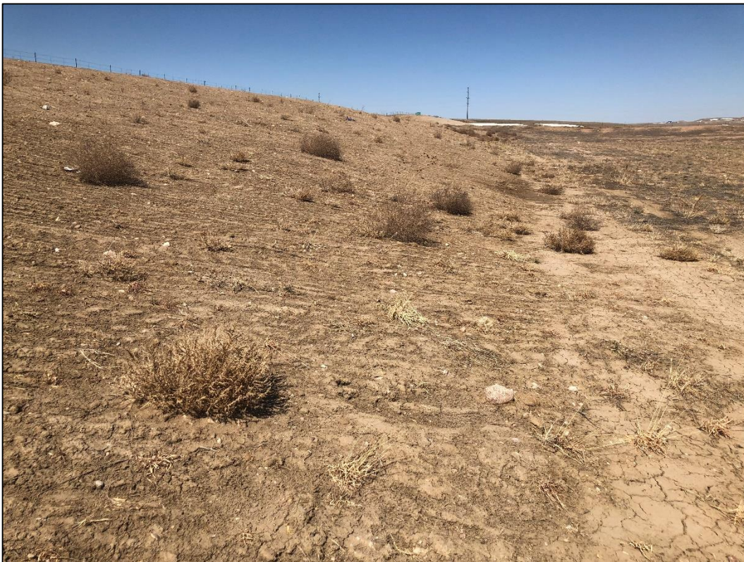
Photo 6. View looking north across pit slope in south mining area, showing slope graded to 3H:1V or flatter. Very little grass growth is present on this slope compared with the pit floor.
