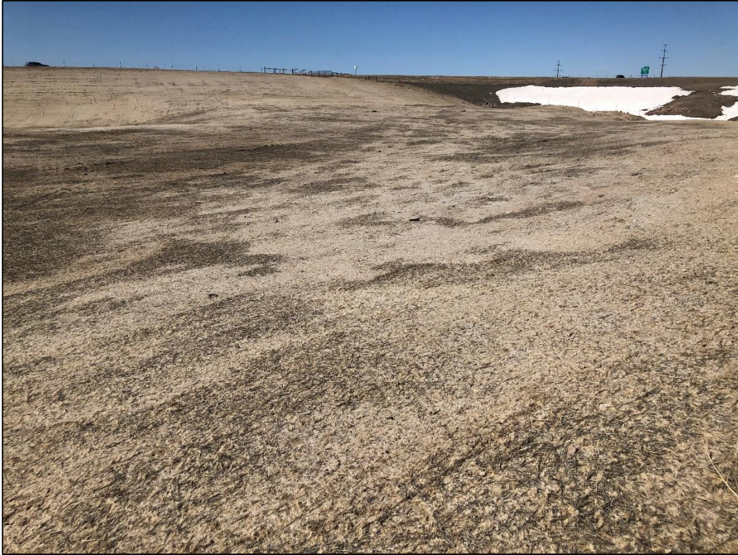
Photo 15. View looking northwest across pit floor of north mining area, showing slopes graded to 3H:1V or flatter. Very little grass growth is present in this area at this time.
