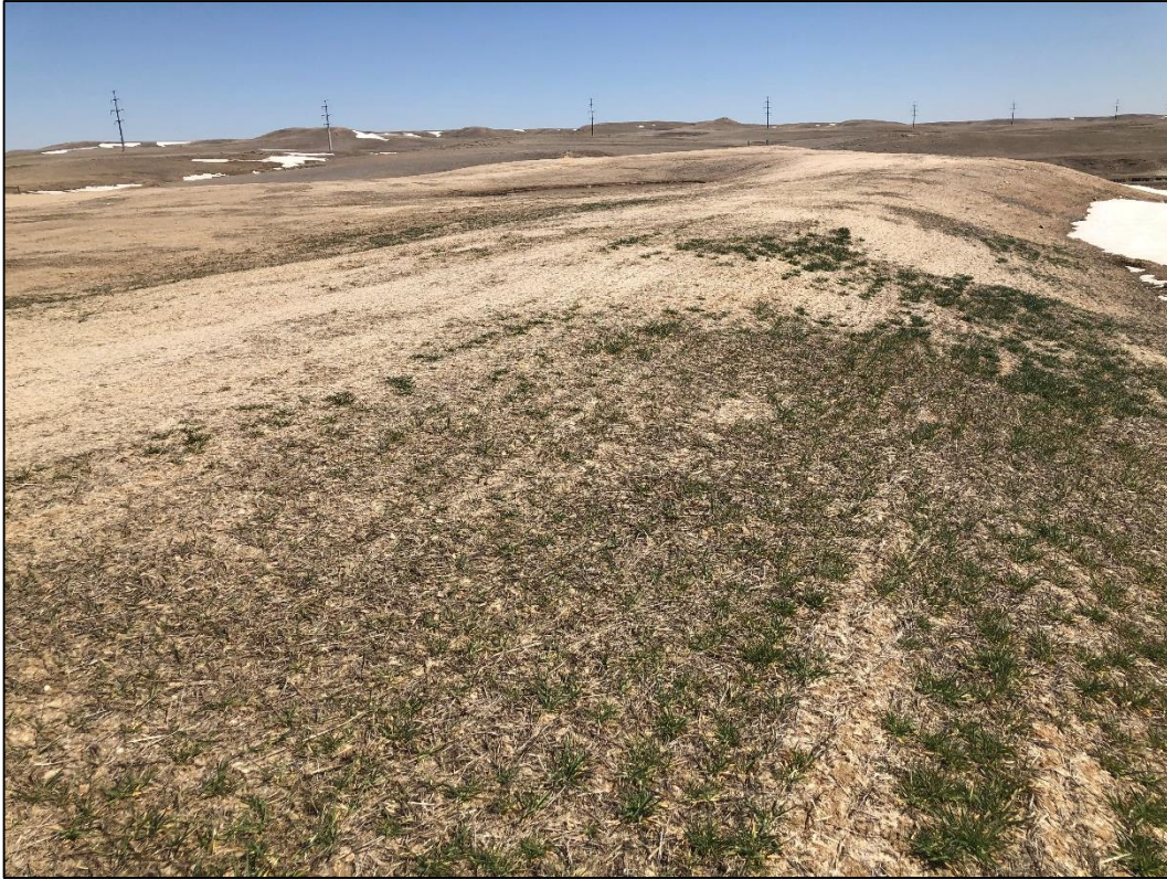
Photo 19. View looking east across southern edge of north mining area, showing slopes graded to 3H:1V or flatter and a bit more grass growth in this area.
