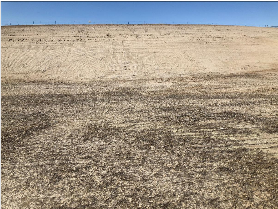
Photo 12. View looking west at pit wall in north mining area, showing slopes graded to 3H:1V or flatter. Very little grass growth is present in this area at this time, especially on the pit slope.
