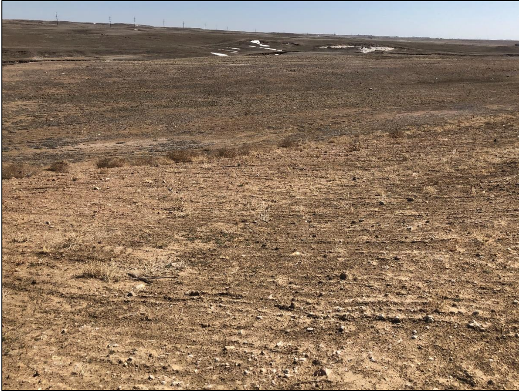
Photo 9. View looking northeast across northern edge of south mining area, showing slopes graded to 3H:1V or flatter. Very little grass growth is present in this area at this time.
