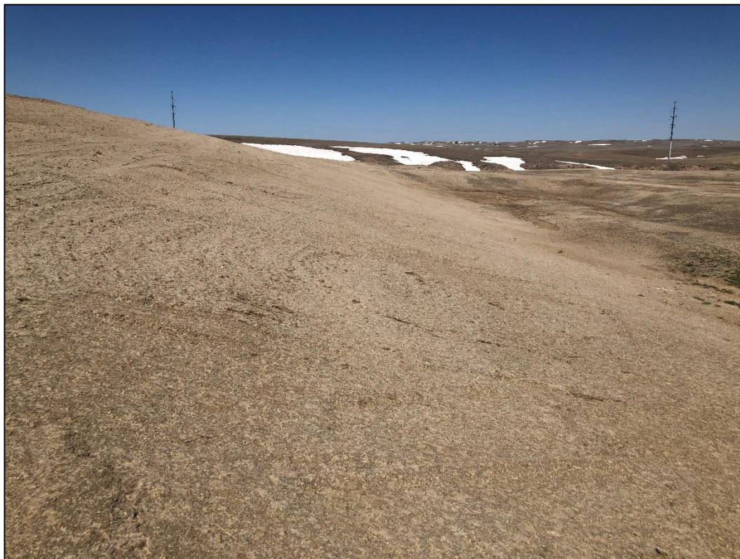
Photo 14. View looking north across pit wall in north mining area, showing slopes graded to 3H:1V or flatter. Very little grass growth is present on the pit slope at this time.
