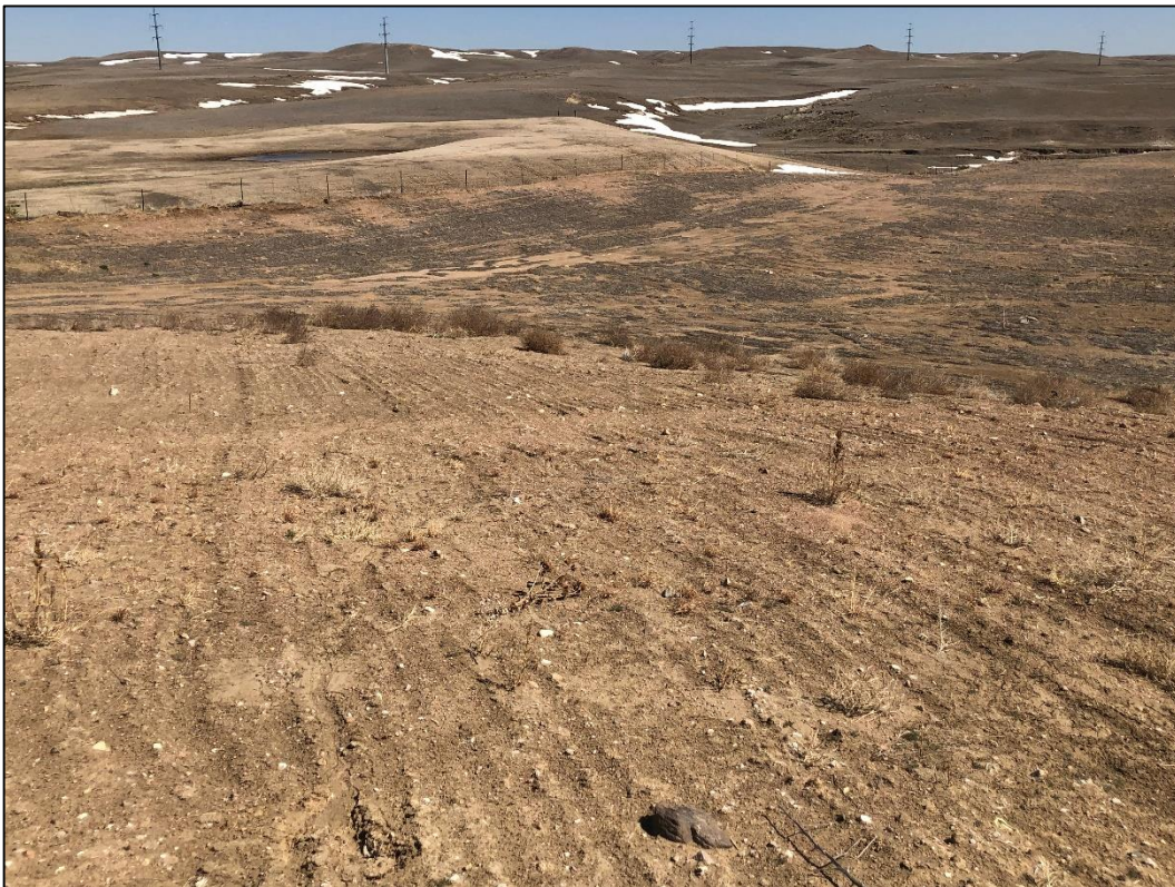
Photo 8. View looking northeast across northern edge of south mining area, showing slopes graded to 3H:1V or flatter. Very little grass growth is present in this area at this time.
