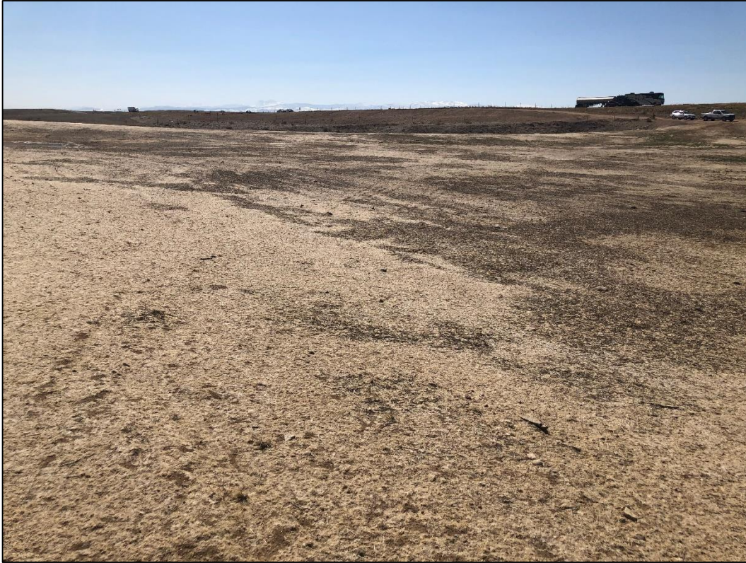
Photo 17. View looking southwest across pit floor of north mining area, showing slopes graded to 3H:1V or flatter. Very little grass growth is present in this area at this time.
