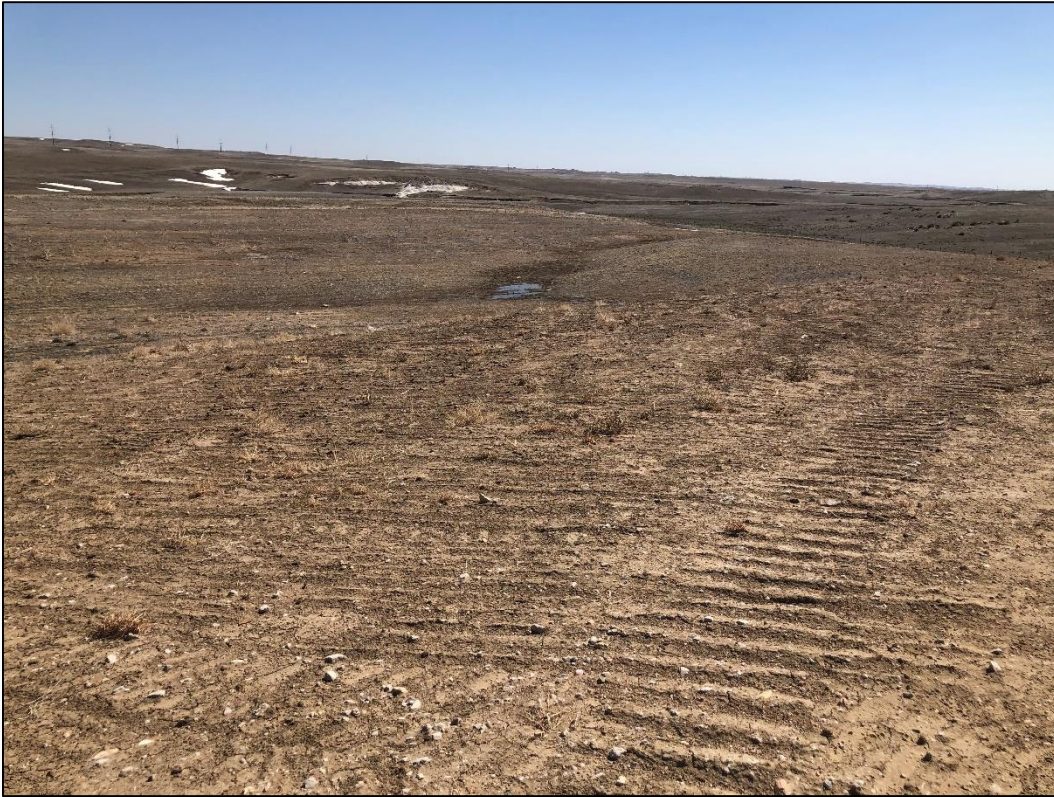
Photo 1. View looking southeast across southern edge of south mining area, showing slopes graded to 3H:1V or flatter. Very little grass growth is present in this area at this time.
