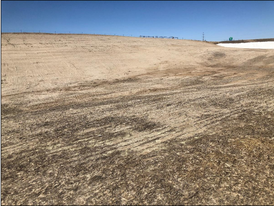
Photo 11. View looking northwest at pit wall in north mining area, showing slopes graded to 3H:1V or flatter. Very little grass growth is present in this area at this time, especially on the pit slope.
