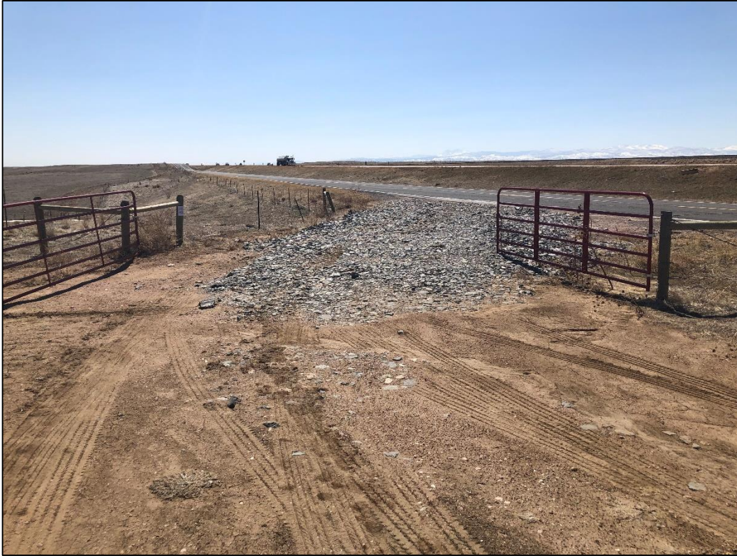
Photo 7. View looking southwest at gated entrance/access road constructed off I-25 frontage road to enter south mining area. This entrance/road will remain for reclamation per the landowner's request.
