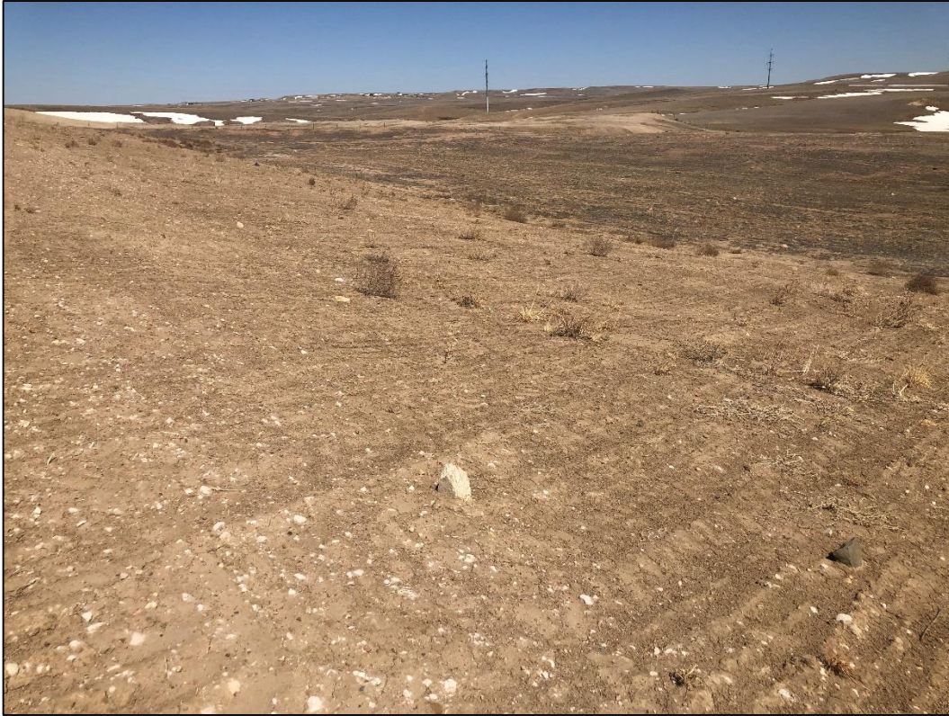
Photo 3. View looking northeast across south mining area, showing slopes graded to 3H:1V or flatter. Very little grass growth is present in this area at this time.
