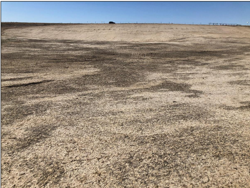
Photo 16. View looking west across pit floor of north mining area, showing slopes graded to 3H:1V or flatter. Very little grass growth is present in this area at this time.
