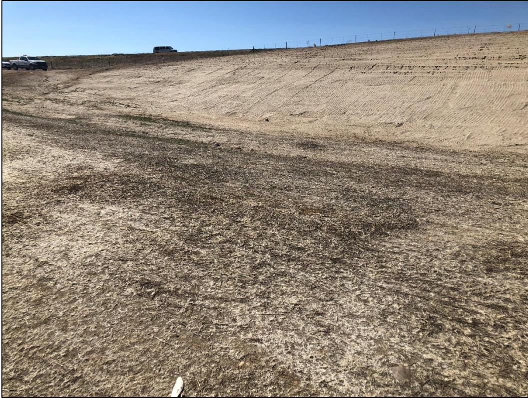
Photo 13. View looking southwest at pit wall in north mining area, showing slopes graded to 3H:1V or flatter. Very little grass growth is present in this area at this time, especially on the pit slope.
