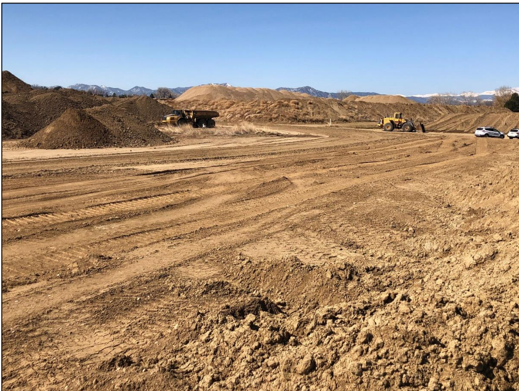
Photo 28. View looking west across topsoil/overburden storage area located west of Reservoir #2 pit and directly south of new (unauthorized) reservoir pit.
