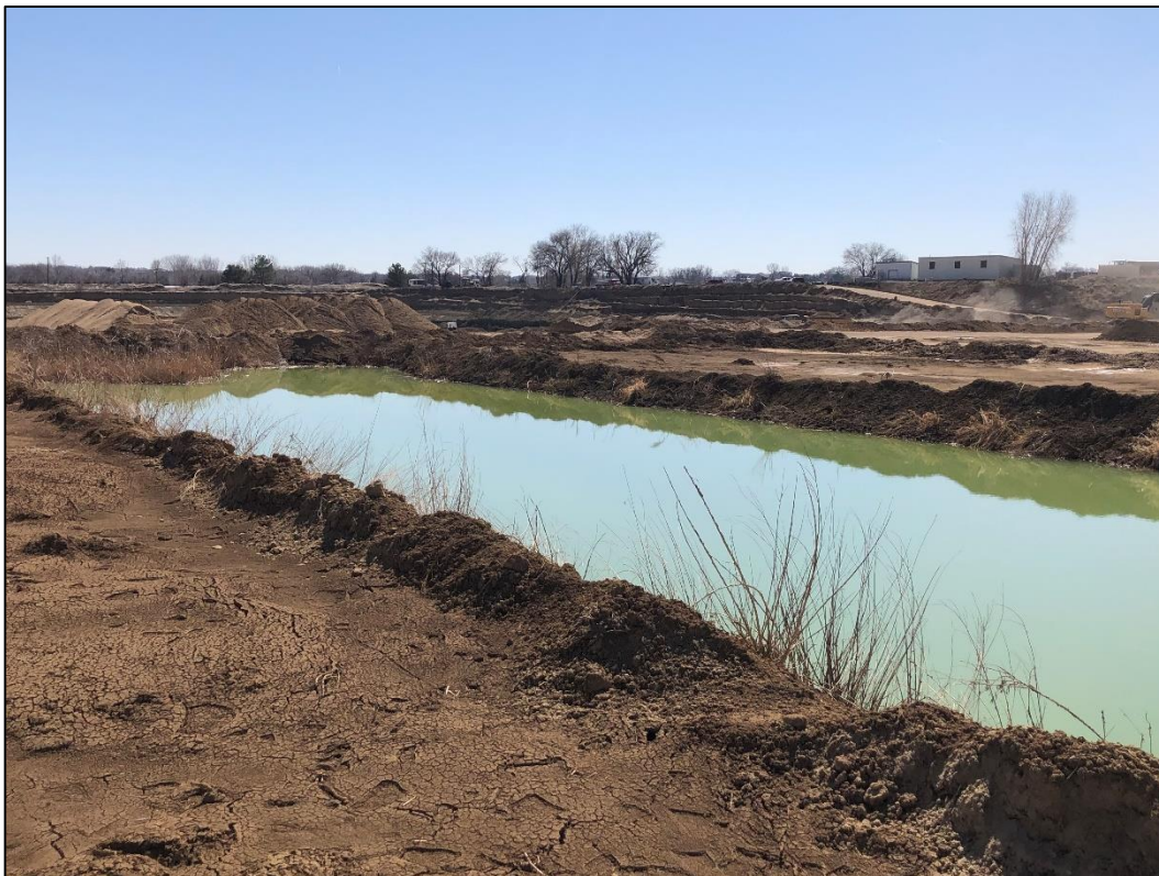
Photo 8. View looking southeast across one of two settling ponds present in northwestern portion of Reservoir #4 pit. Water from settling ponds is routed north of site to eventually discharge into Boulder Creek.
