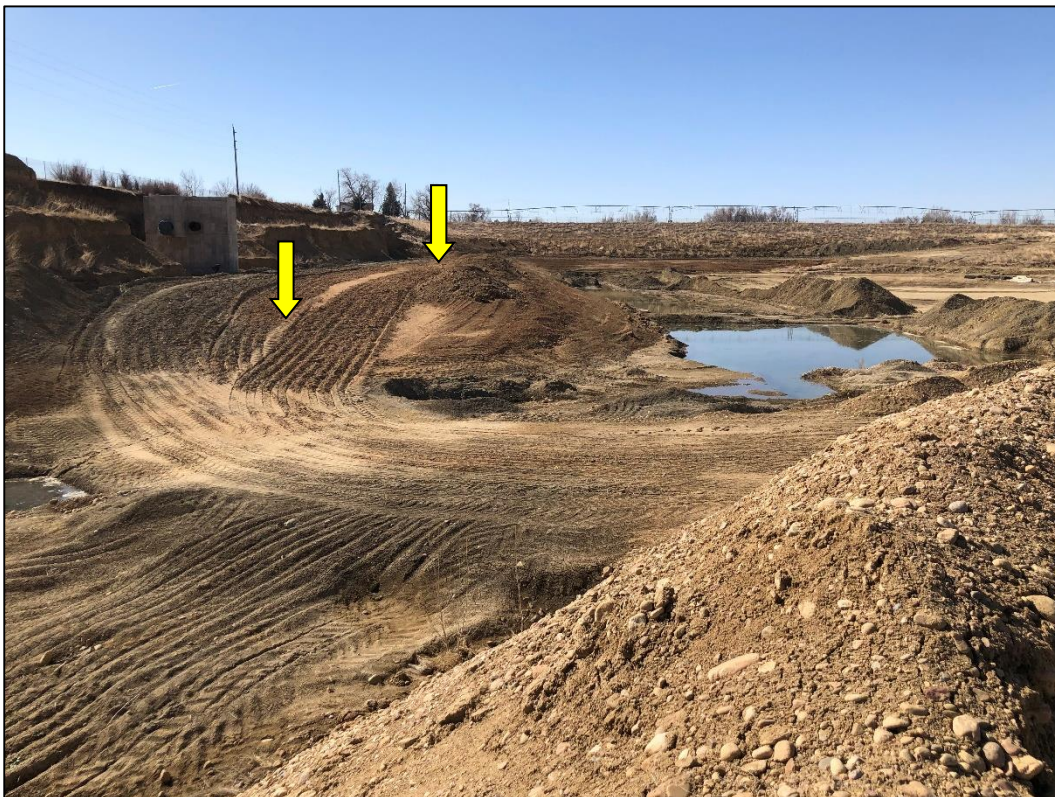
Photo 14. View looking south across eastern edge of Reservoir #2 pit, showing partially installed clay liner (indicated with arrows). Note standing water on pit floor.
