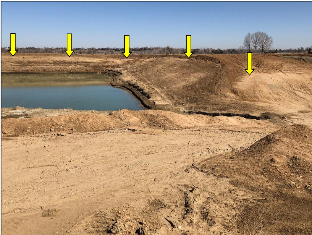
Photo 18. View looking north across eastern portion of new (unauthorized) reservoir pit, showing partially installed clay liner (indicated with arrows) forming “dam” and standing water on pit floor. Note inside slopes of clay liner at 3H:1V or flatter.
