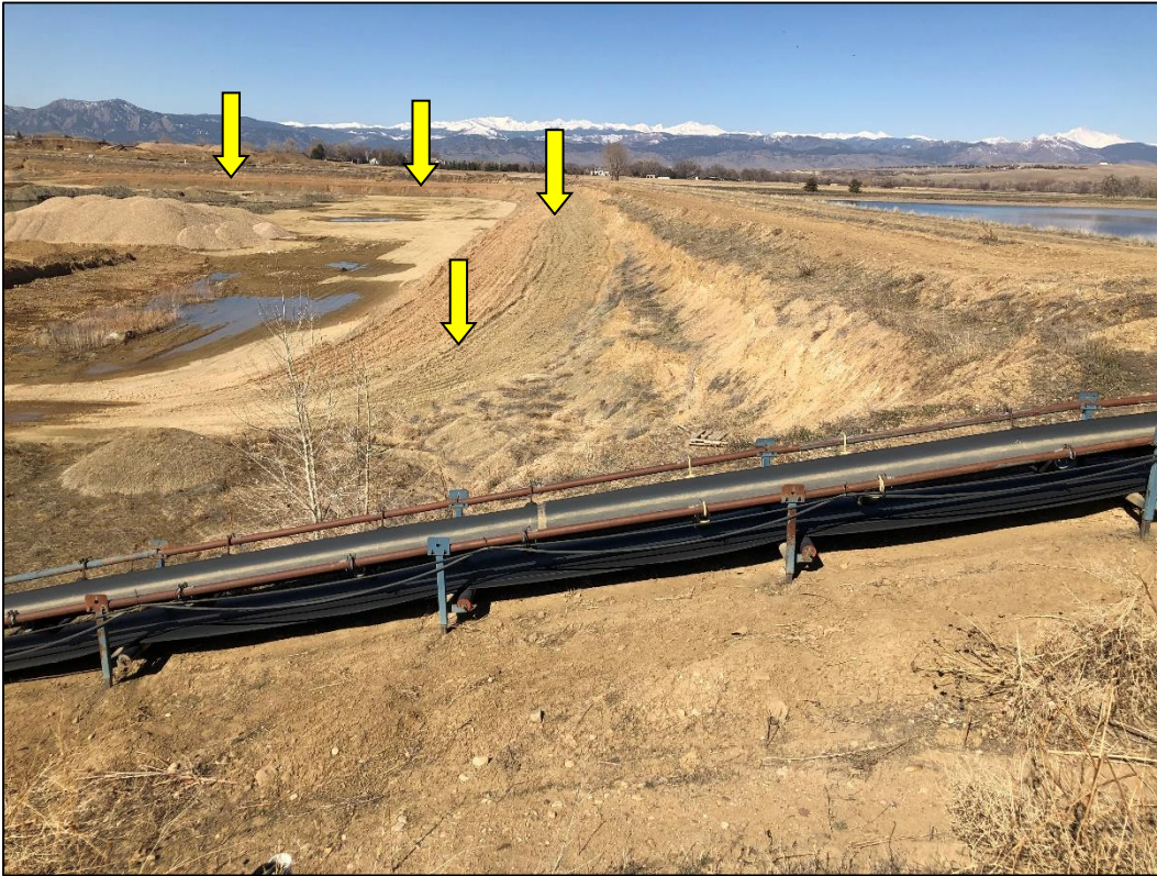
Photo 11. View looking west across northern edge of Reservoir #2 pit. Note partially installed clay liner (indicated with arrows).
