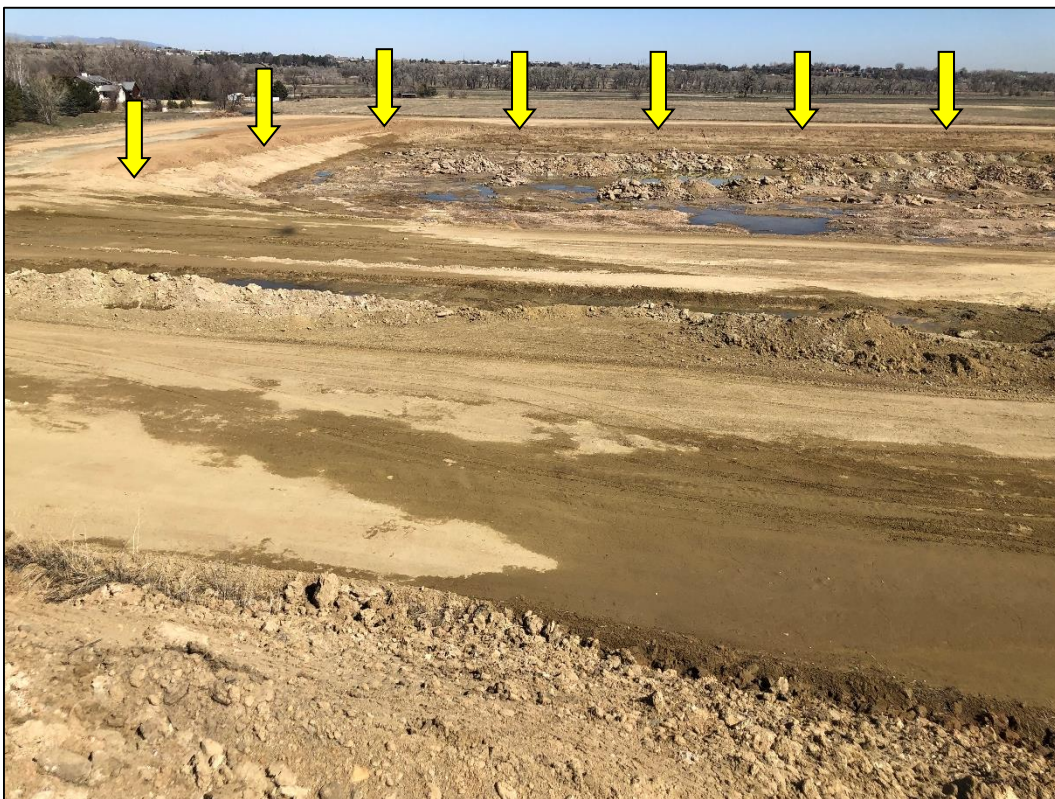
Photo 24. View looking north across western edge of new (unauthorized) reservoir pit, showing partially installed clay liner (indicated with arrows) and standing water on pit floor. Note inside slopes of clay liner at 3H:1V or flatter.
