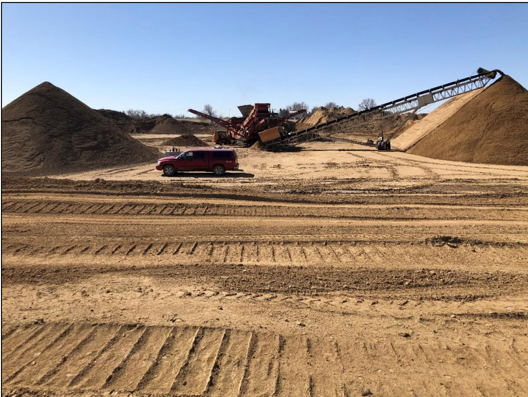
Photo 26. View looking south across topsoil/overburden storage area located west of Reservoir #2 pit and directly south of new (unauthorized) reservoir pit. It appears this area is also being used to process material for pit liner construction.
