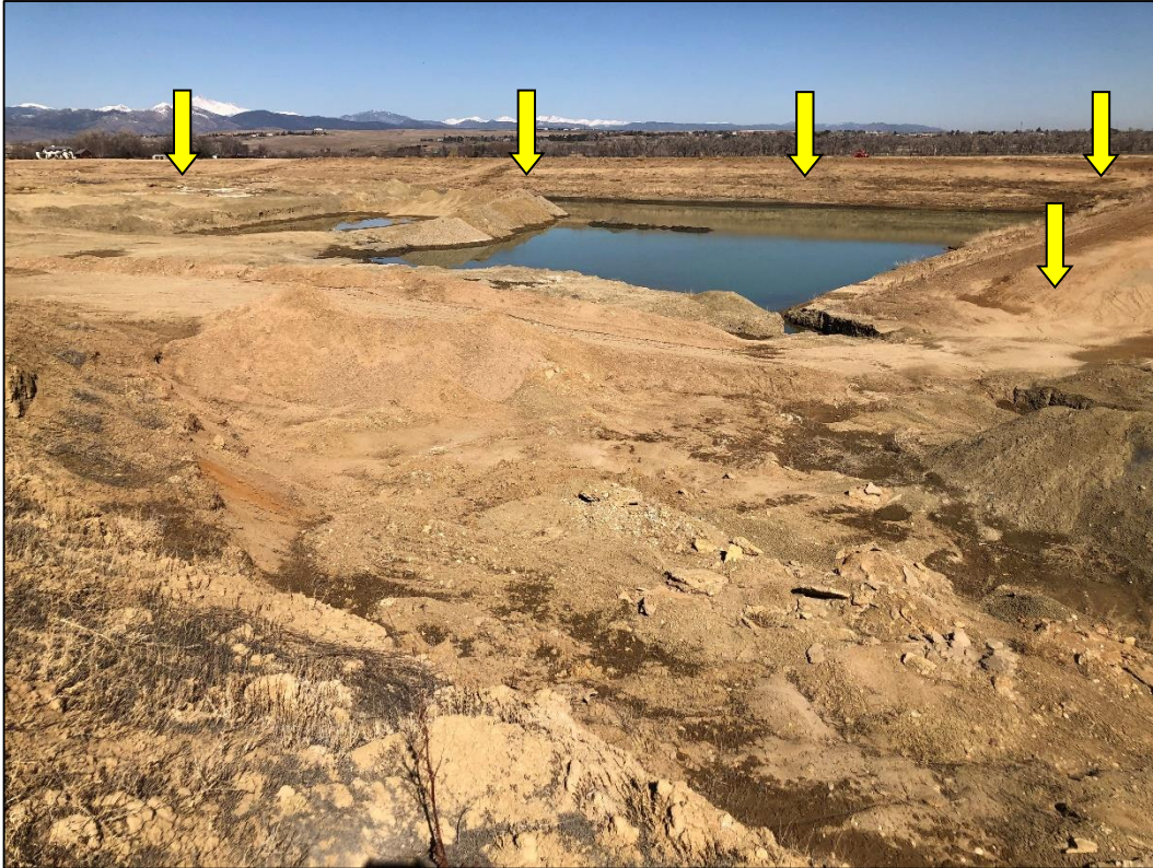
Photo 19. View looking northwest across eastern portion of new (unauthorized) reservoir pit, showing partially installed clay liner (indicated with arrows) and material stockpiles on pit floor. Note standing water on pit floor.
