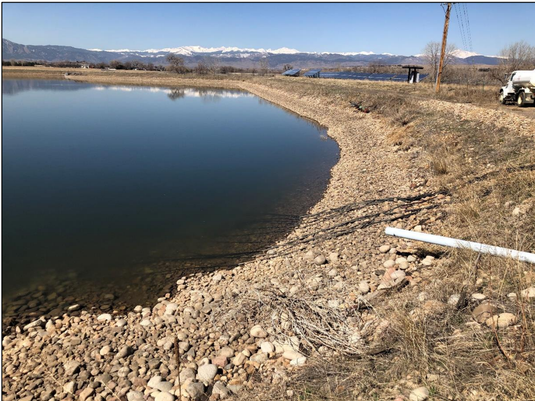
Photo 30. View looking west across northern edge of existing clay-lined Reservoir #1 located in northwestern portion of permit area.
