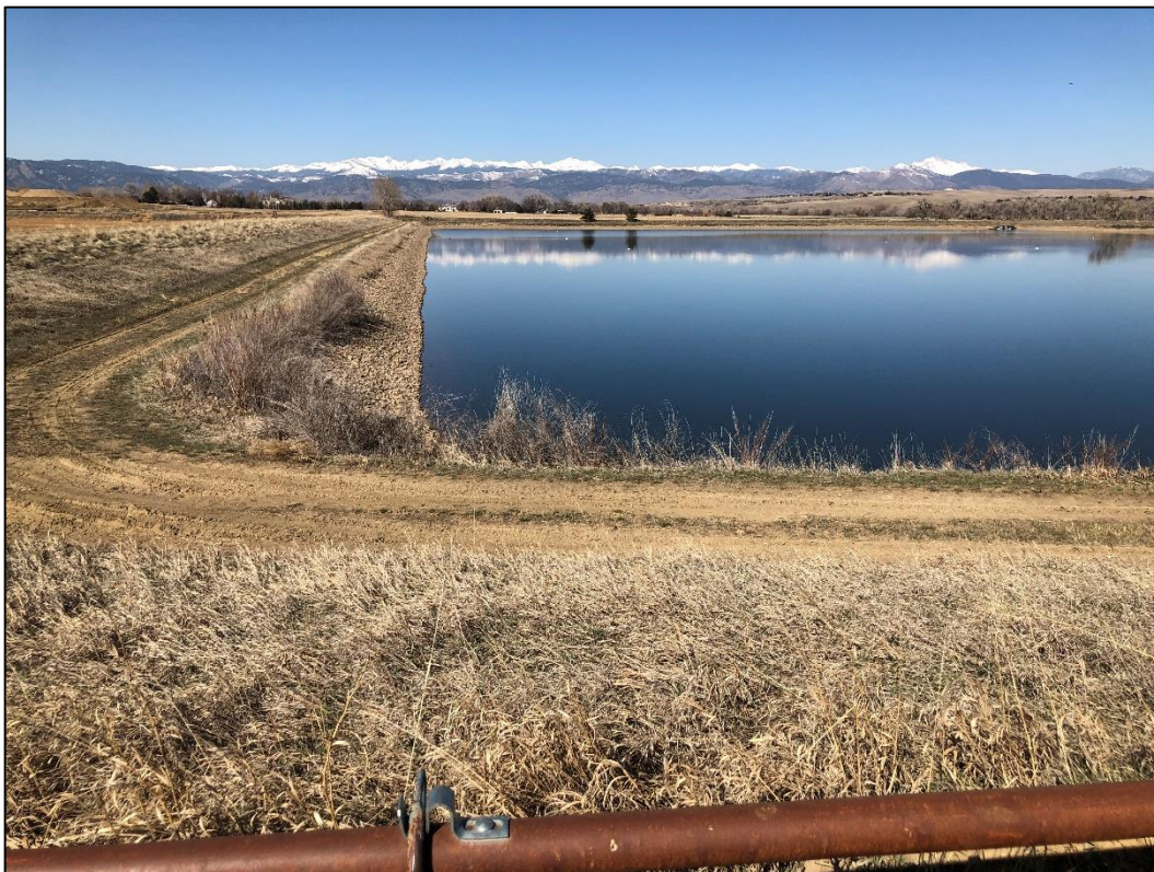
Photo 32. View looking west across southern edge of existing clay-lined Reservoir #1 located in northwestern portion of permit area.
