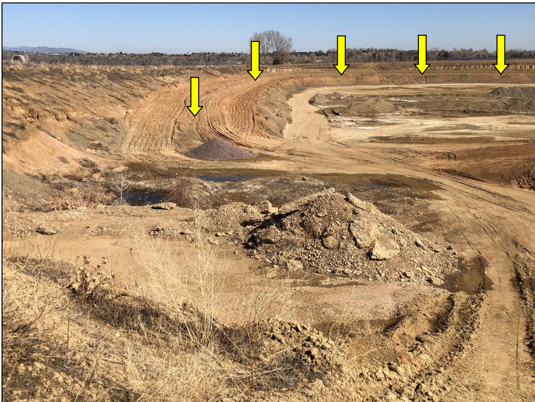
Photo 16. View looking north across western edge of Reservoir #2 pit, showing partially installed clay liner (indicated with arrows).
