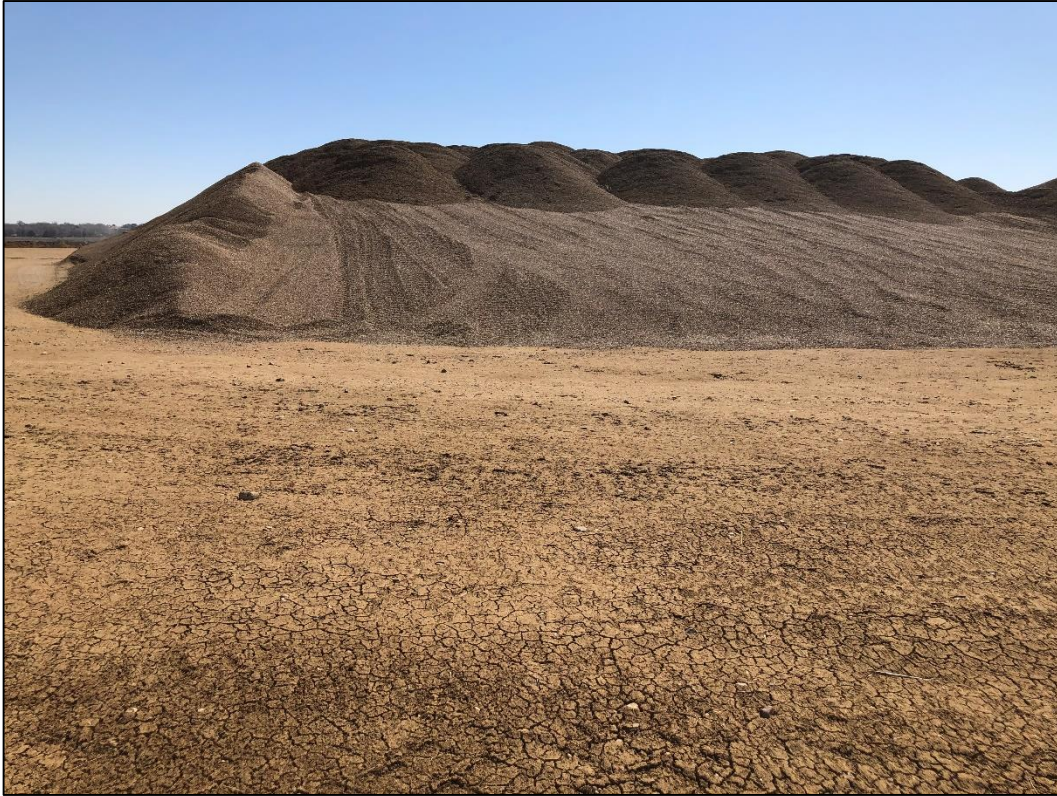
Photo 29. View looking east at large gravel stockpile stored at western edge of topsoil/overburden storage area. This material will be used to construct the protective upper shell along the upper portion of clay-lined reservoir slopes.
