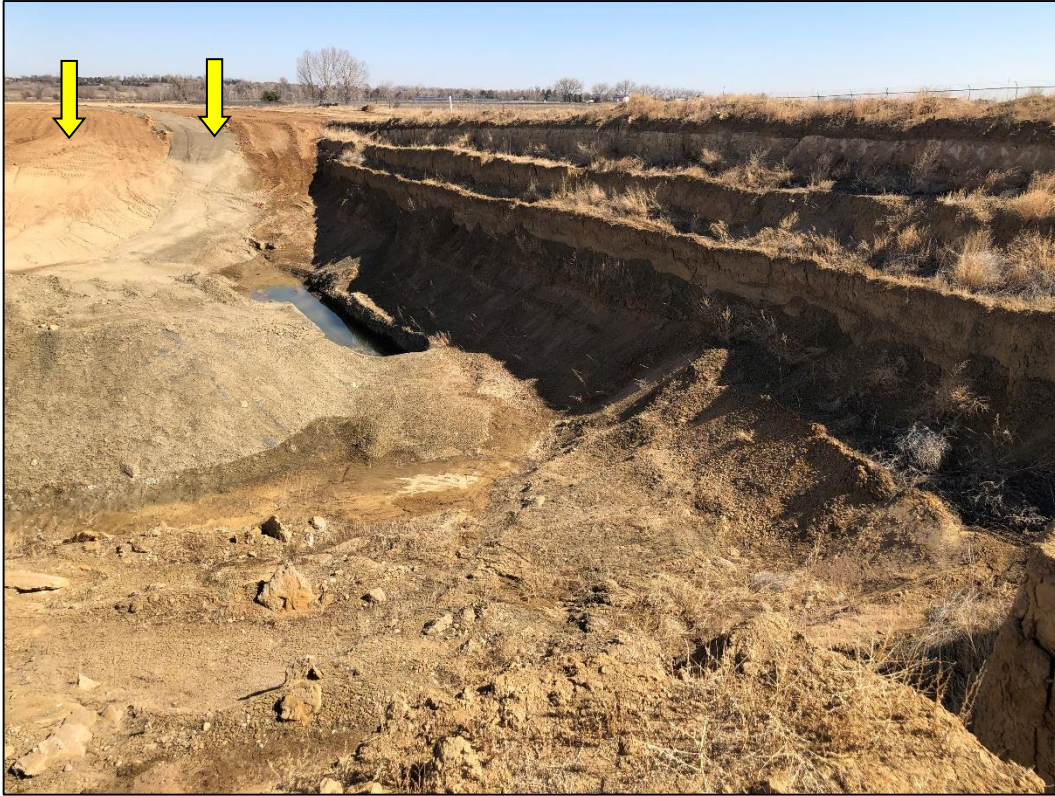
Photo 17. View looking north across eastern edge of new (unauthorized) reservoir pit, showing near vertical highwalls and partially installed clay liner (indicated with arrows) forming “dam”.
