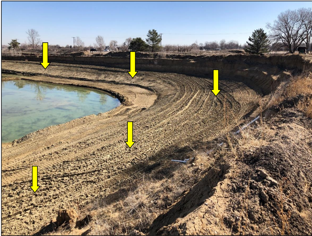
Photo 1. View looking east across southeastern edge of Reservoir # 4 pit, showing partially installed clay liner (indicated with arrows) with slopes of 3H:1V or flatter. Note standing water on pit floor.
