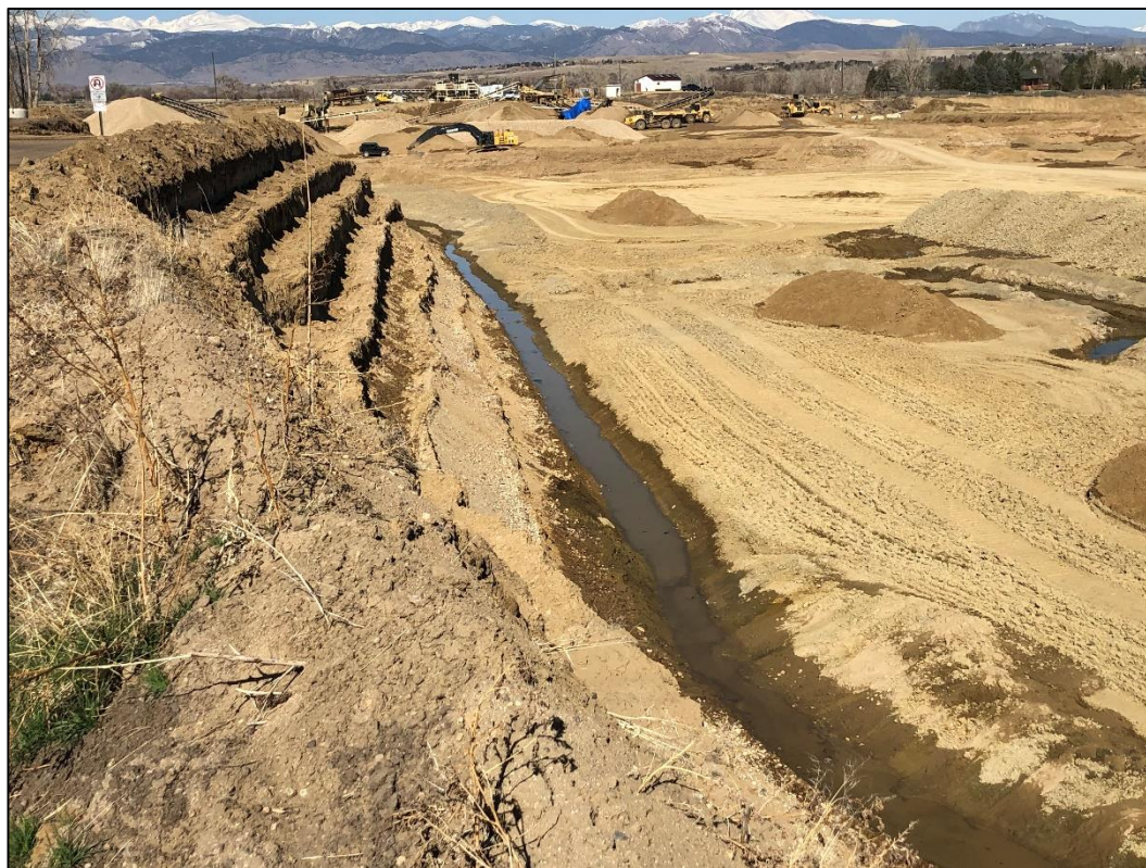
Photo 4. View looking west across southern edge of Reservoir # 4 pit. Note dewatering trench present along inside perimeter of pit and clay liner not yet installed in this area.
