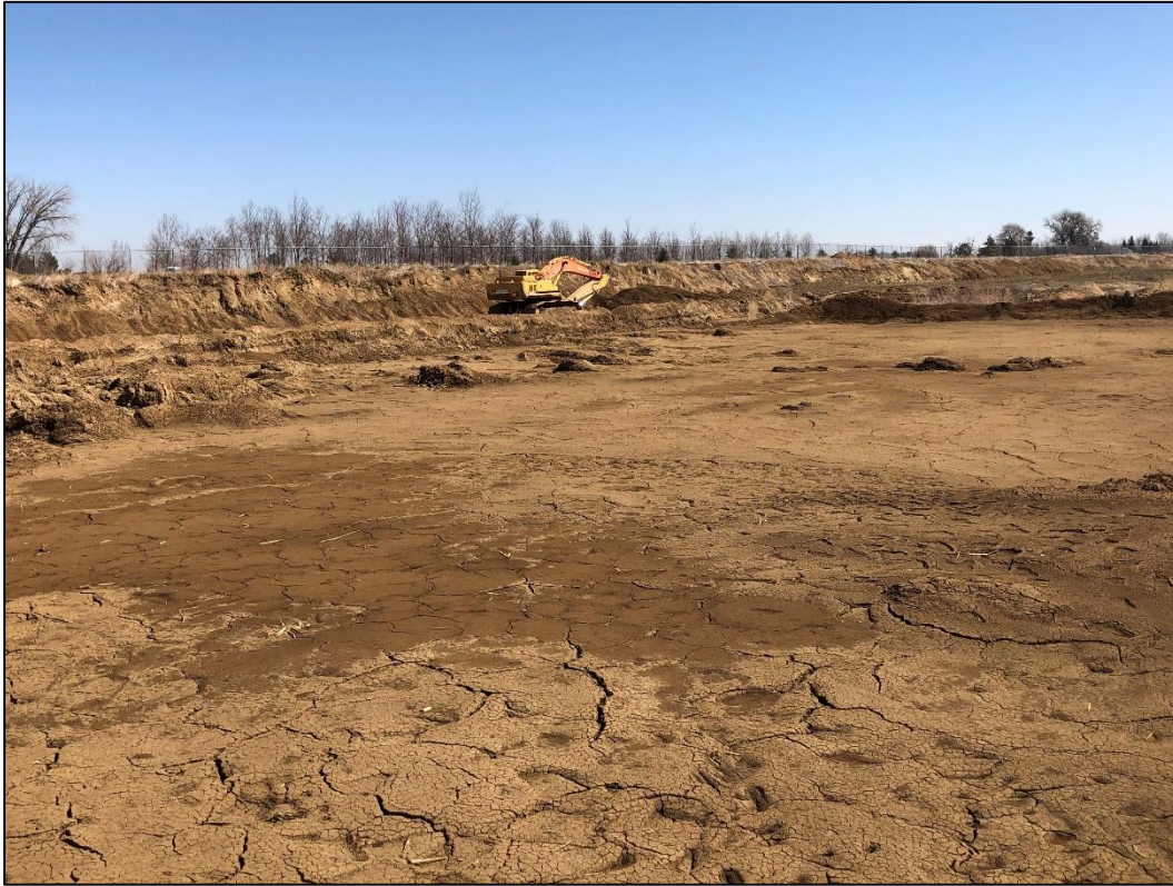
Photo 7. View looking northeast across northwestern portion of Reservoir #4 pit. This portion of the pit will be mined deeper. The clay liner has not yet been installed in this area.
