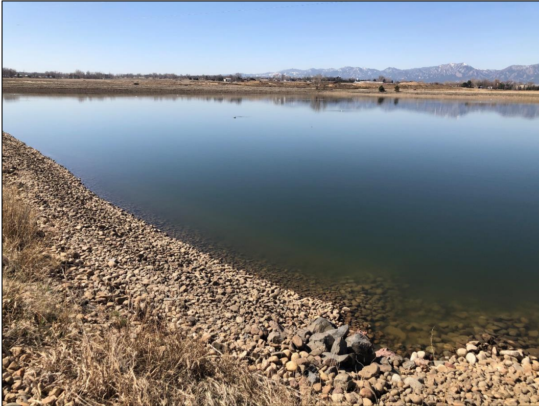
Photo 31. View looking southwest across existing clay-lined Reservoir #1 located in northwestern portion of permit area.
