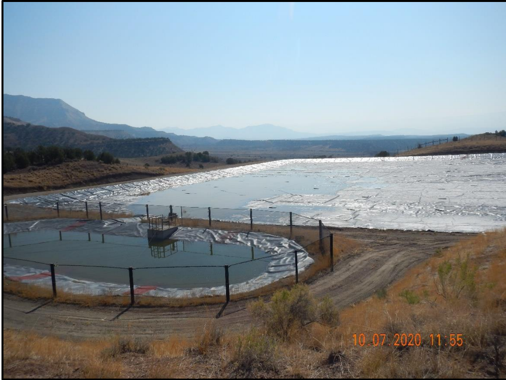
Photo 5. Settling Pond and Evaporation Pond, October, 2020.
