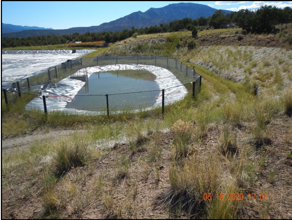
Photo 1. Settling Pond with installed bird netting, June, 2020.
