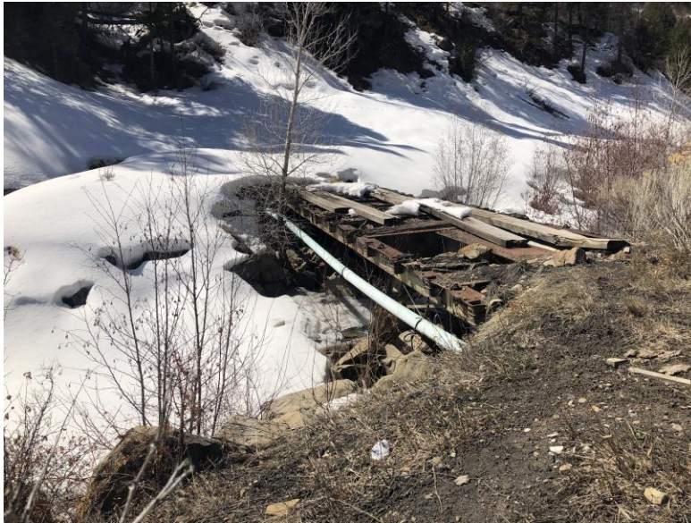
Pipe crossing creek on bridge
