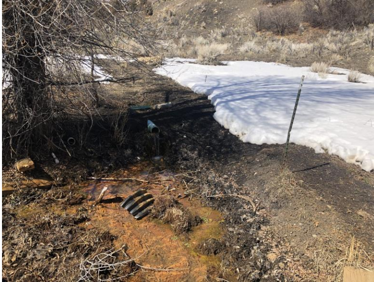
Discharge pipe at top of treatment system
