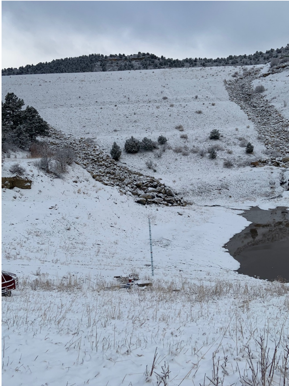
Refuse Disposal Area – Reclaimed Benches and Armored Drainage
