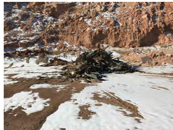
5. DEMOLITION DEBRIS PLACED AT TOE OF SLIDE
