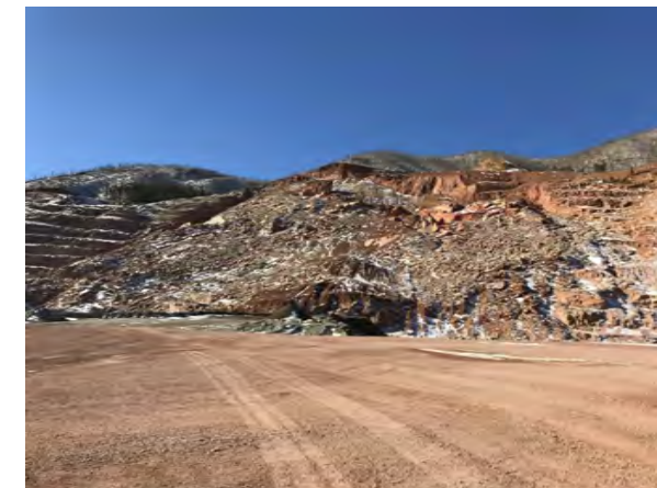
4. FILL DEPOSITED AT TOE OF SLIDE AREA
