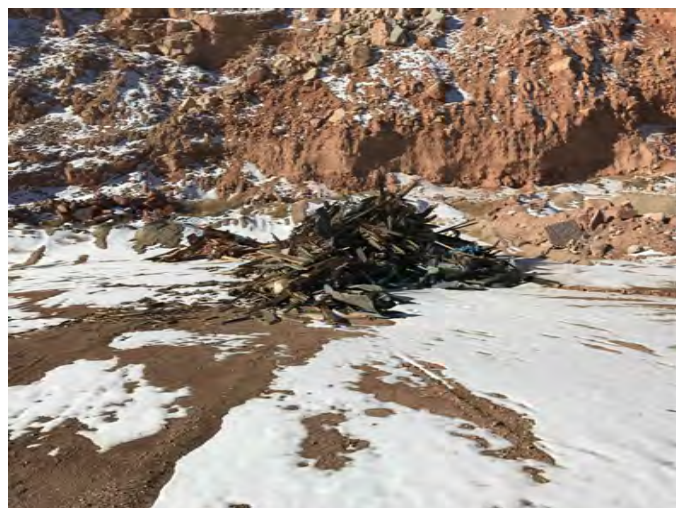
5. DEMOLITION DEBRIS PLACED AT TOE OF SLIDE
