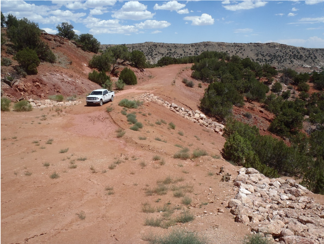
Photo 7. Riprap channels constructed on south edge of fines area & from lower access road.
