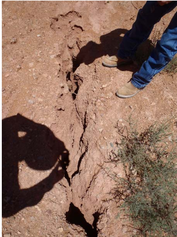
Photo 5. Hydraulic sink near terrace channel intersection with riprap channel.
