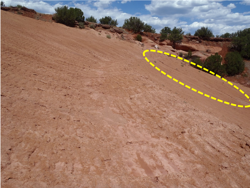
Photo 3. Terrace bench/channel & minor erosion rill (circled).
