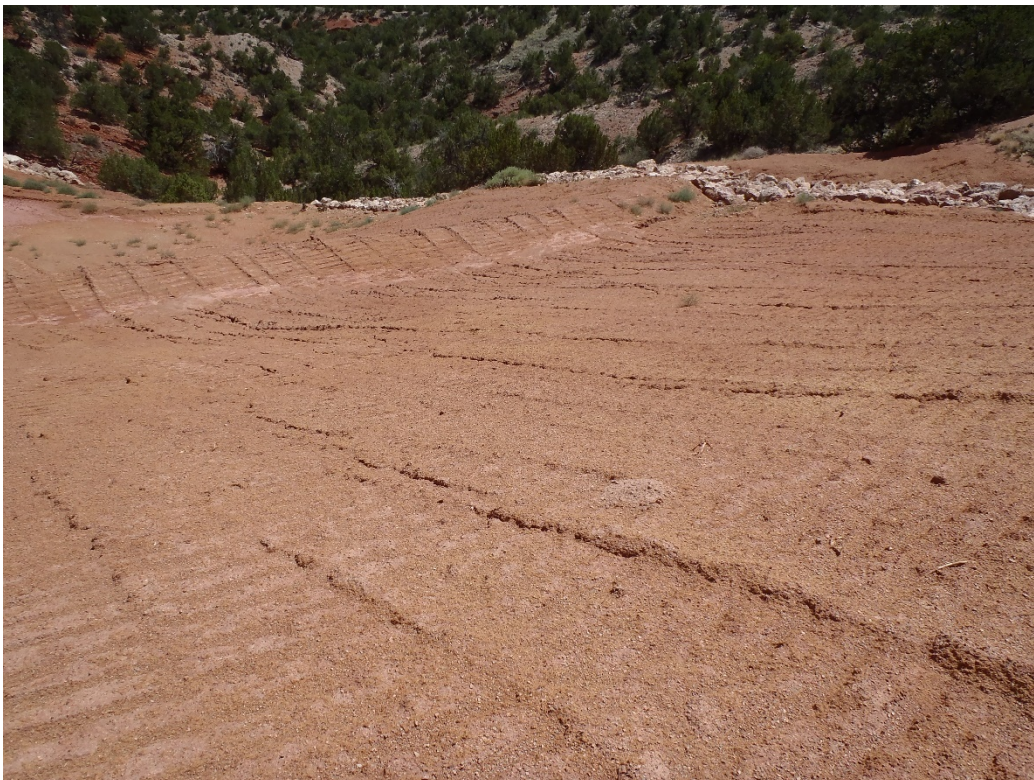
Photo 4. Dozer tracked surface above terrace channel (looking SE from crest).
