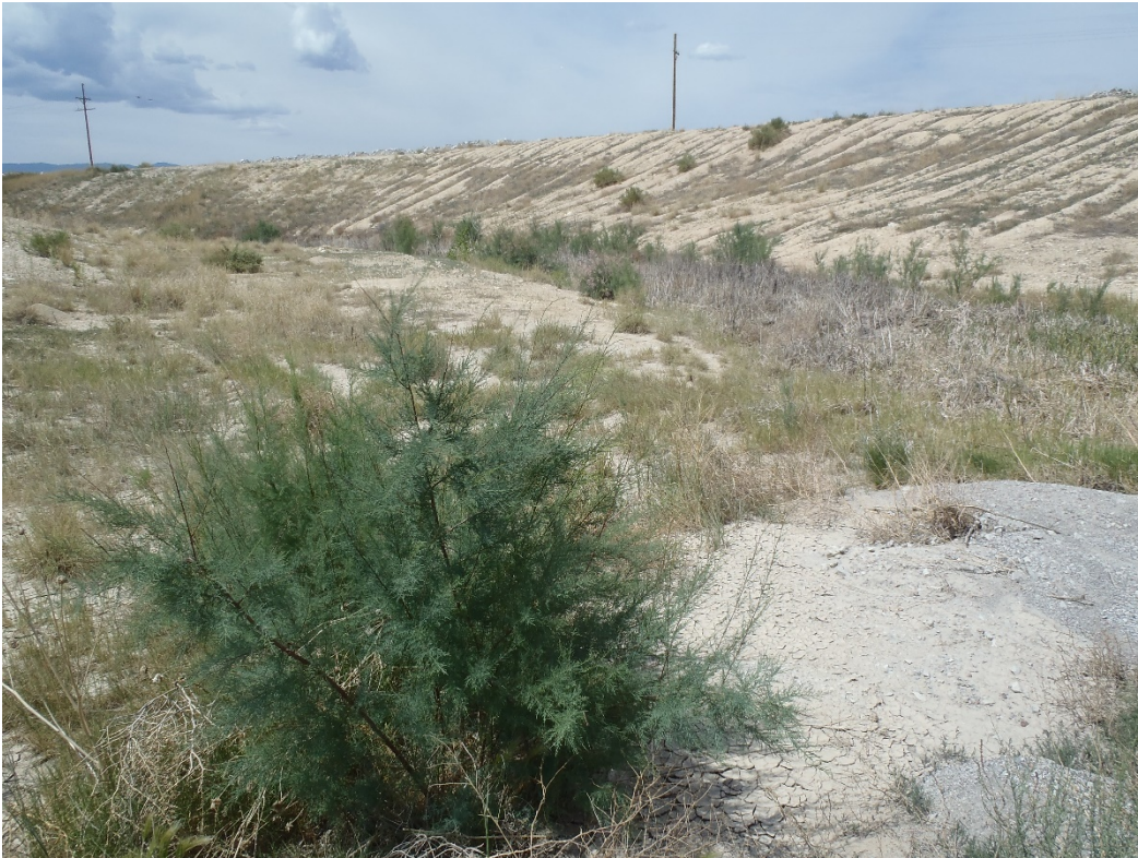
Photo 5. Tamarisk (foreground) and minor erosion rills on slope above diversion channel (looking south from north access road).
