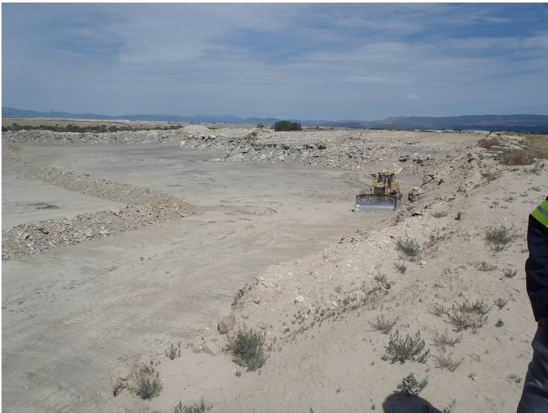
Photo 2. Overburden removal on NE corner of active pit (looking NW).
