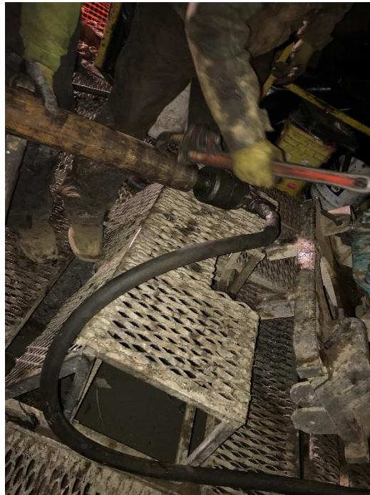
6. Grout injection head mounted on top of HQ rod
