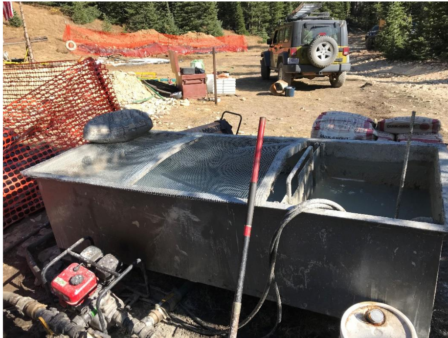
5. Grout mixing tank
