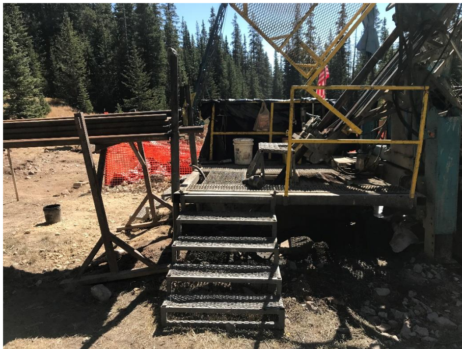
2. WP-6 borehole location with drill rig and HQ rod prior to abandonment
