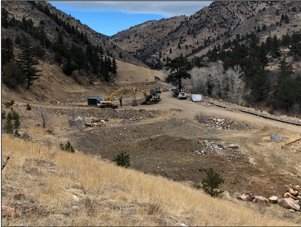
Photo 1. View looking northwest across valley from top of mesa (with new water treatment plant). Old structures have been removed from site (including old water treatment plant and concrete basins) so underlying radionuclide-impacted soils can be excavated.
