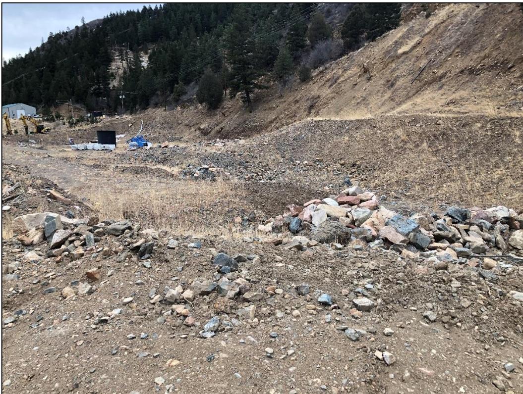
Photo 4. View looking south across northwestern portion of valley where activities have been primarily focused for valley excavation project. According to operator, the deepest excavation depths were in this area along the southern edge of the valley, at approximately 12-13 feet deep.
