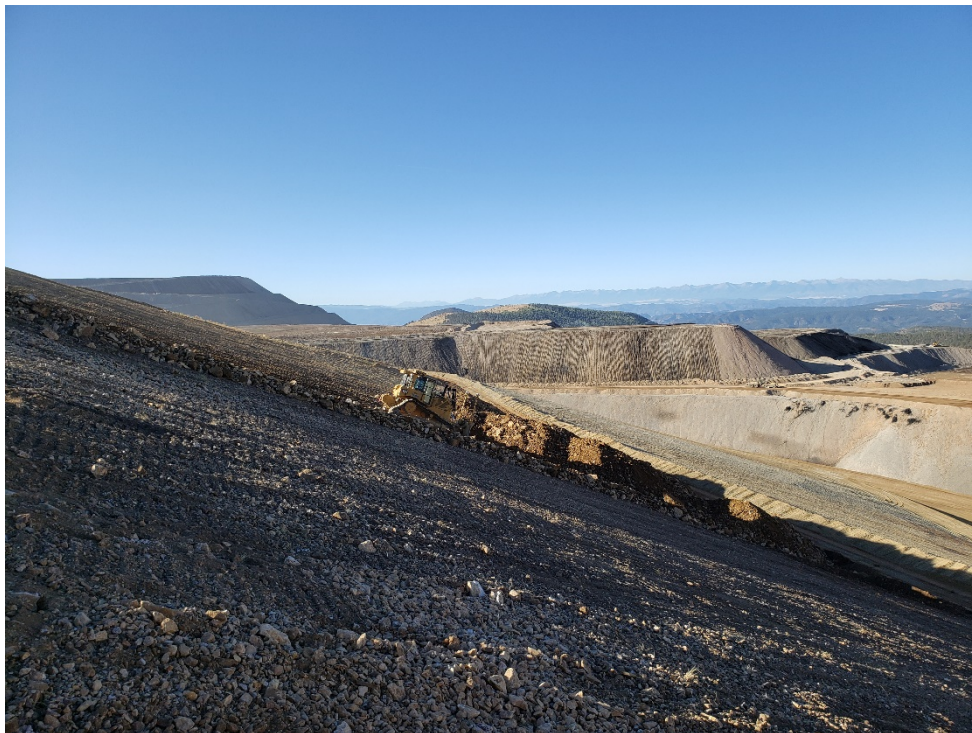
September 25, 2019 – Finish grading of the Phase 2B slope (TGW)
