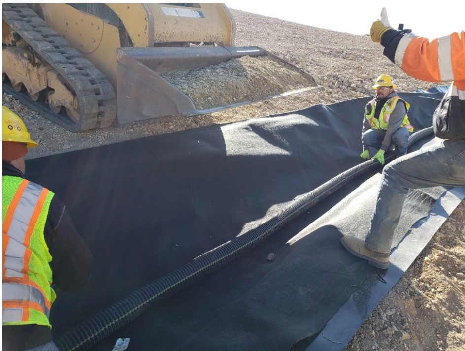
October 8th, 2019 – Installation phase 2B leak detection trench (TGW)
