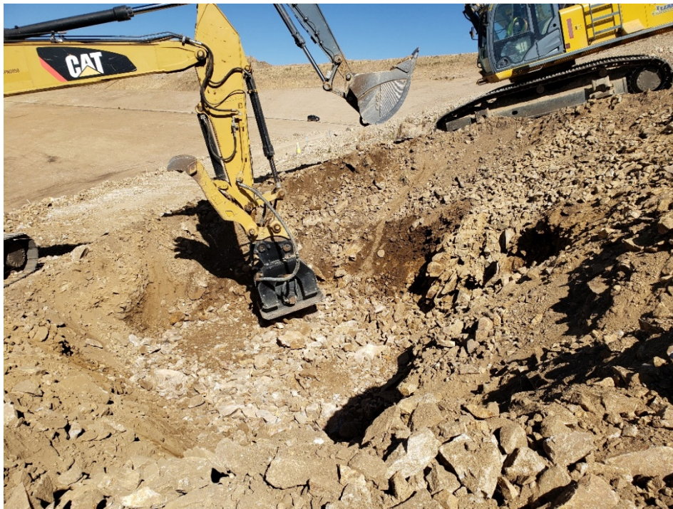
October 8th, 2019 – Structural fill placement on UG #6699 (TGW)
