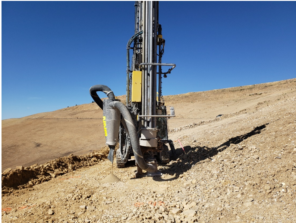
September 24, 2019 – Confirmatory drilling of UG #6617 (TGW)
