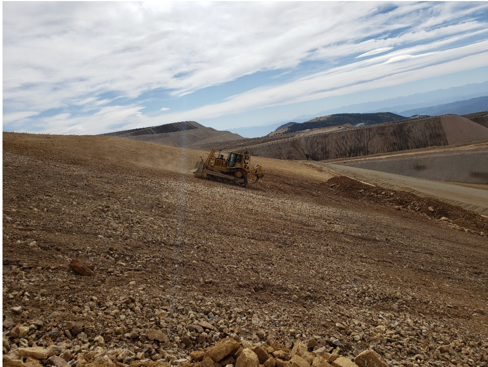
September 26, 2019 – Finish grading of the Phase 2B slope (TGW)
