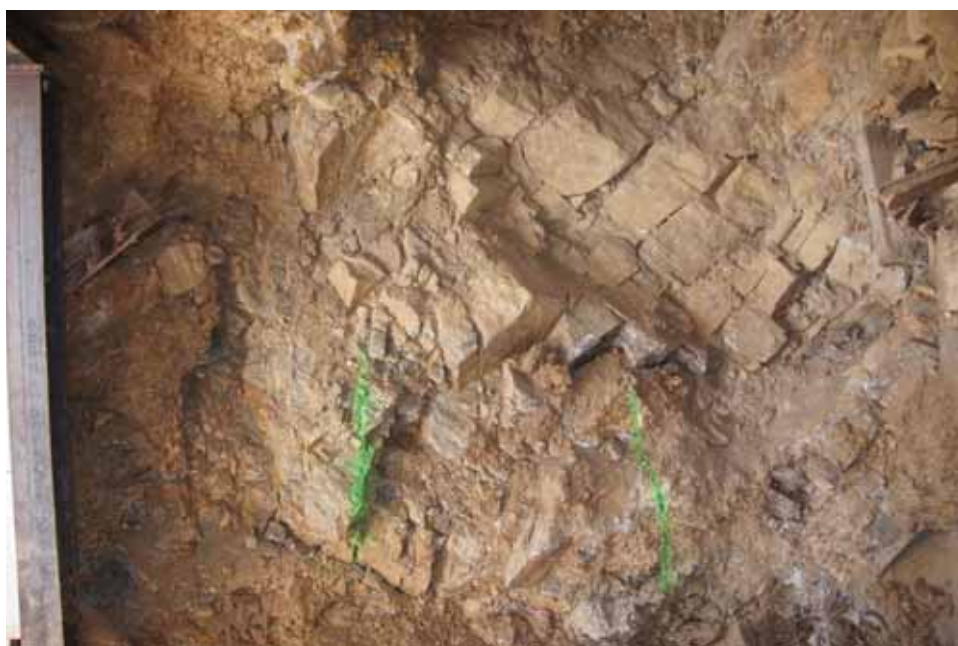
Photograph 3 – Weathered and fractured gneiss in the left rib beneath the portal collapse. Green paint marks at 4-ft intervals mark the approximate location for the next steel sets.
