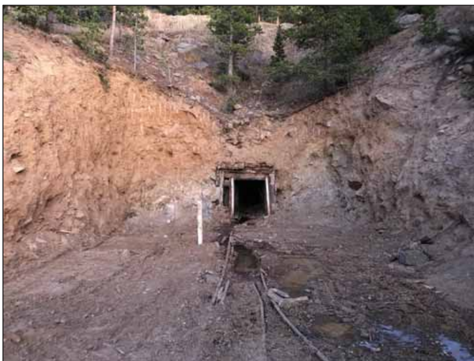
Photograph 7 – Idaho Tunnel Portal following excavation
