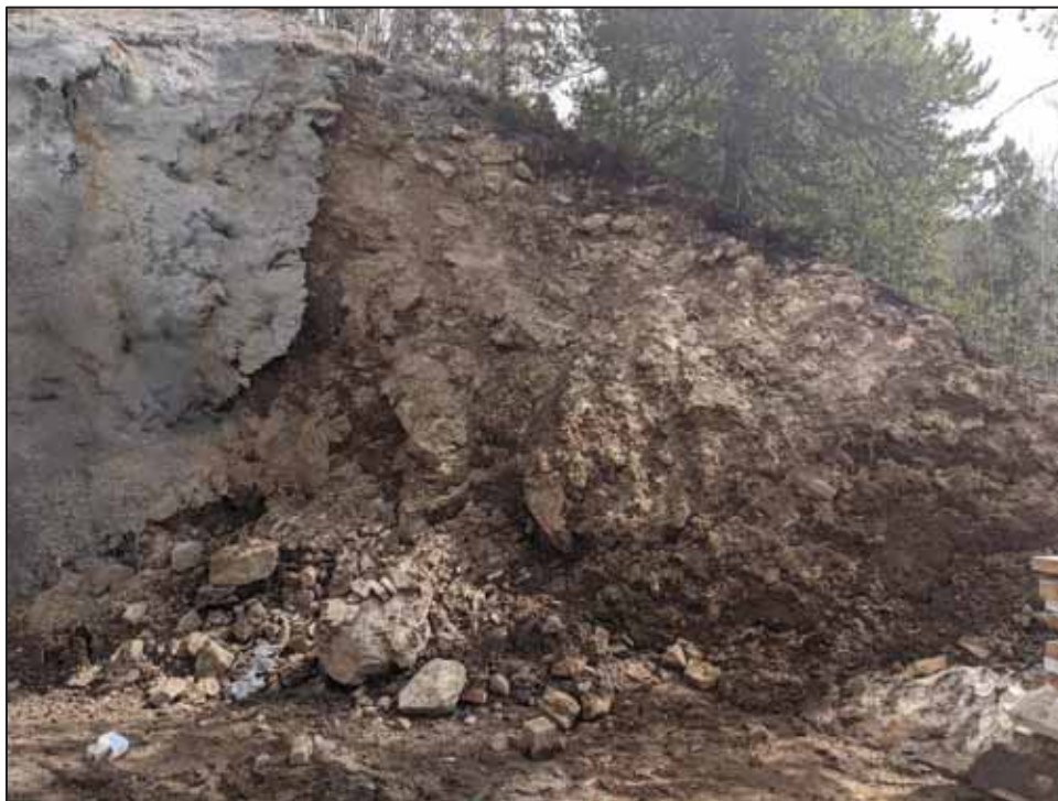
Photograph 6 – Regolith and colluvium exposed in the right (north) wing wall of the portal excavation.
