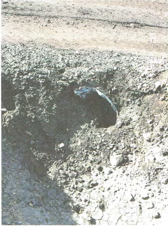
Pic. 5 – Damaged culvert at top of embankment pile (upstream end).
