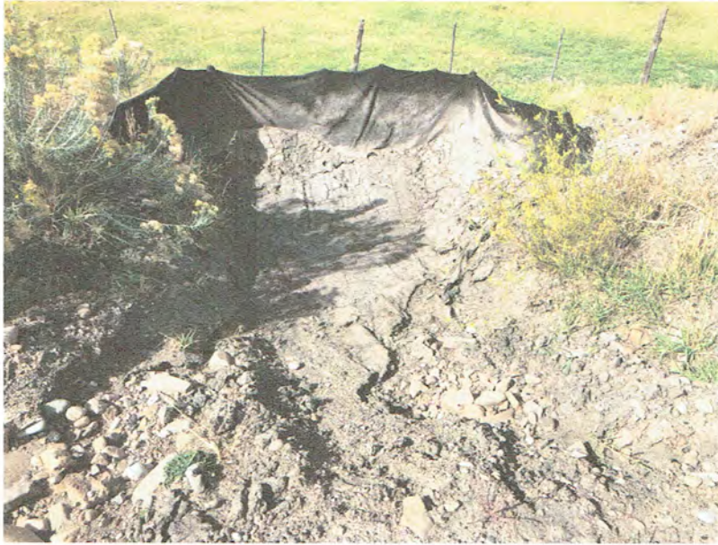
Pic. 3 – Sediment trap at driveway.
