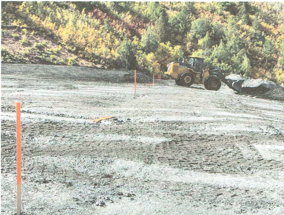
Pic 4 – Staking for the extension of haul road at top of pile.
