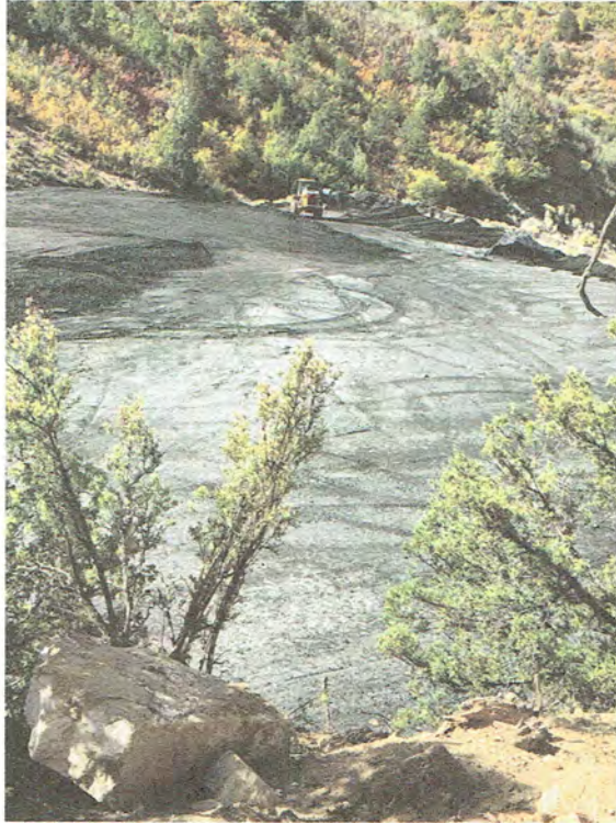
Pic. 3 – Waste material being installed at top of waste embankment pile.
