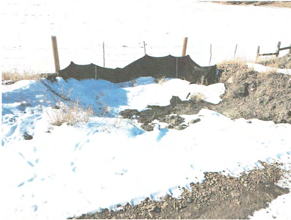
Pic. 3 – Sediment trap at driveway.
