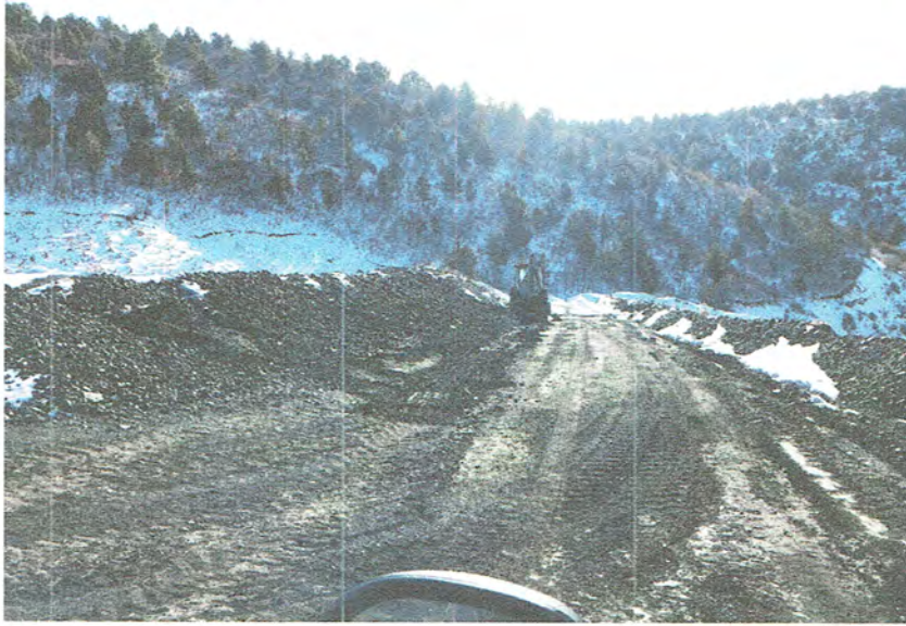
Pic. 5 – Ditch being constructed along haul road above new switchback.
