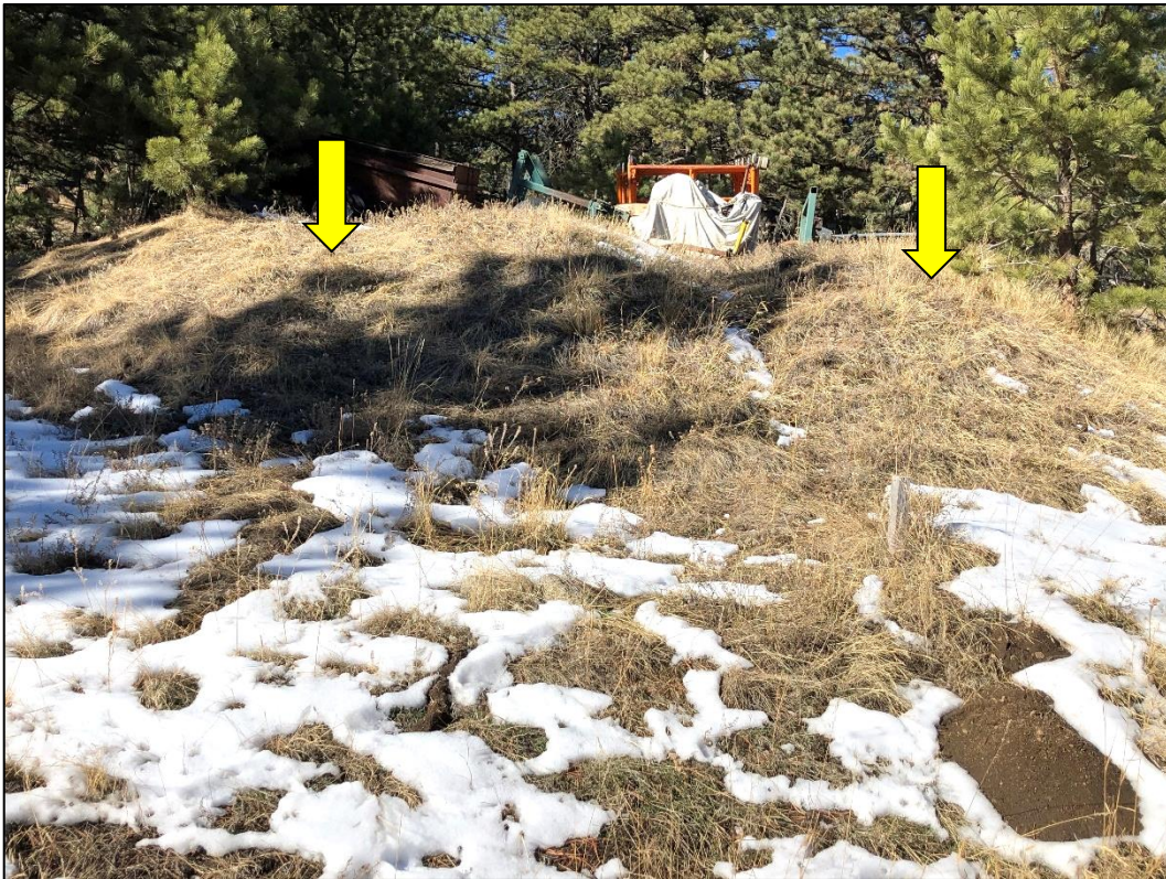
Photo 10. View looking southwest at topsoil stockpile (indicated) stored at northern edge of permit area, outside of fenced enclosure. Note stockpile stable with good grass cover.
