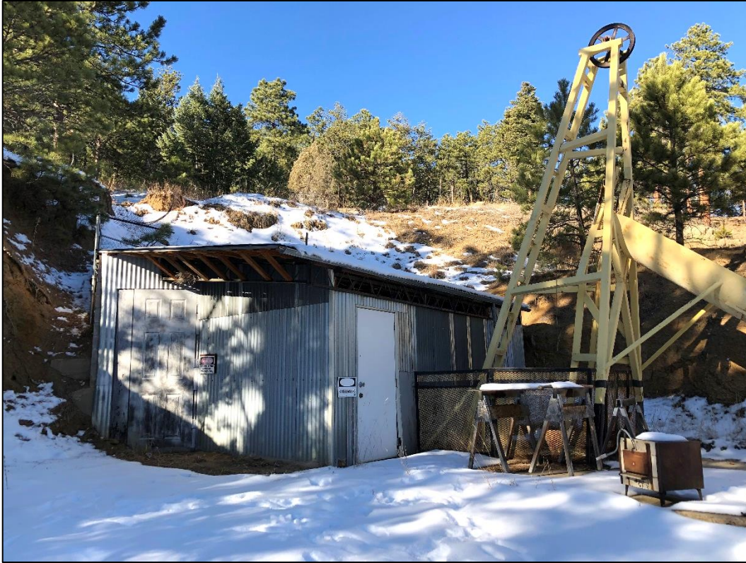
Photo 3. Closer view of fenced mine shaft, steel headframe above shaft, and winch house constructed of corrugated metal, located at southwestern edge of mining area.
