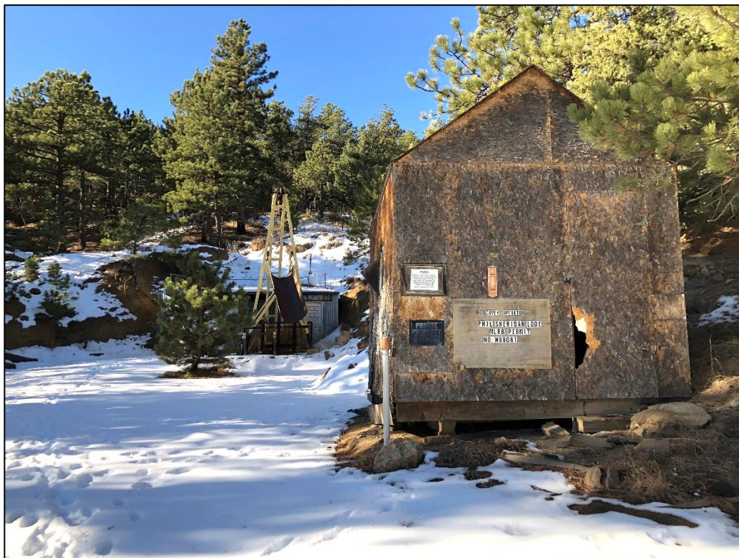
Photo 2. View looking southwest across mining area, showing equipment shed constructed of particle board (in foreground) and mine shaft, headframe, and winch house (in background).
