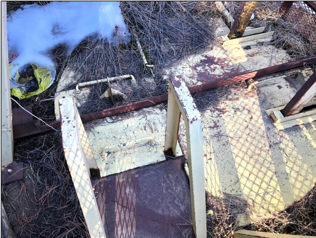
Photo 4. Closer view of mine shaft collared in concrete slab and secured by covered locking device.
