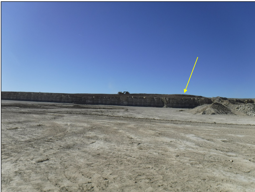
Photo 6: Scraper transporting overburden material to be placed, yellow arrow indicate topsoil stockpile, note highwall below scraper
