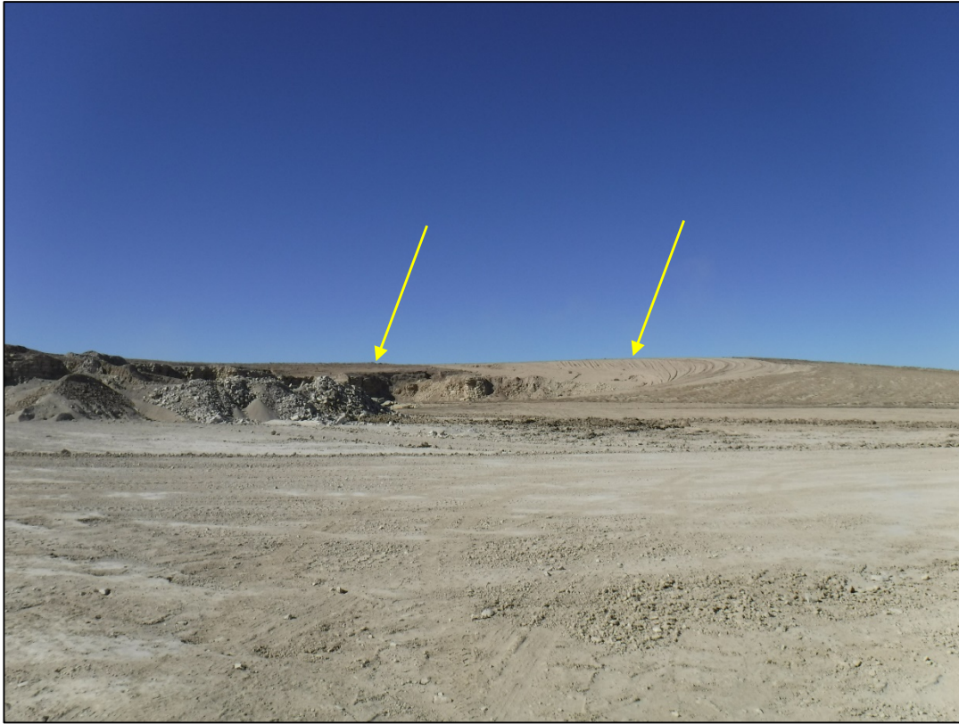
Photo 5: Reclaiming activities, yellow arrows indicate mine face and concurrent reclamation
