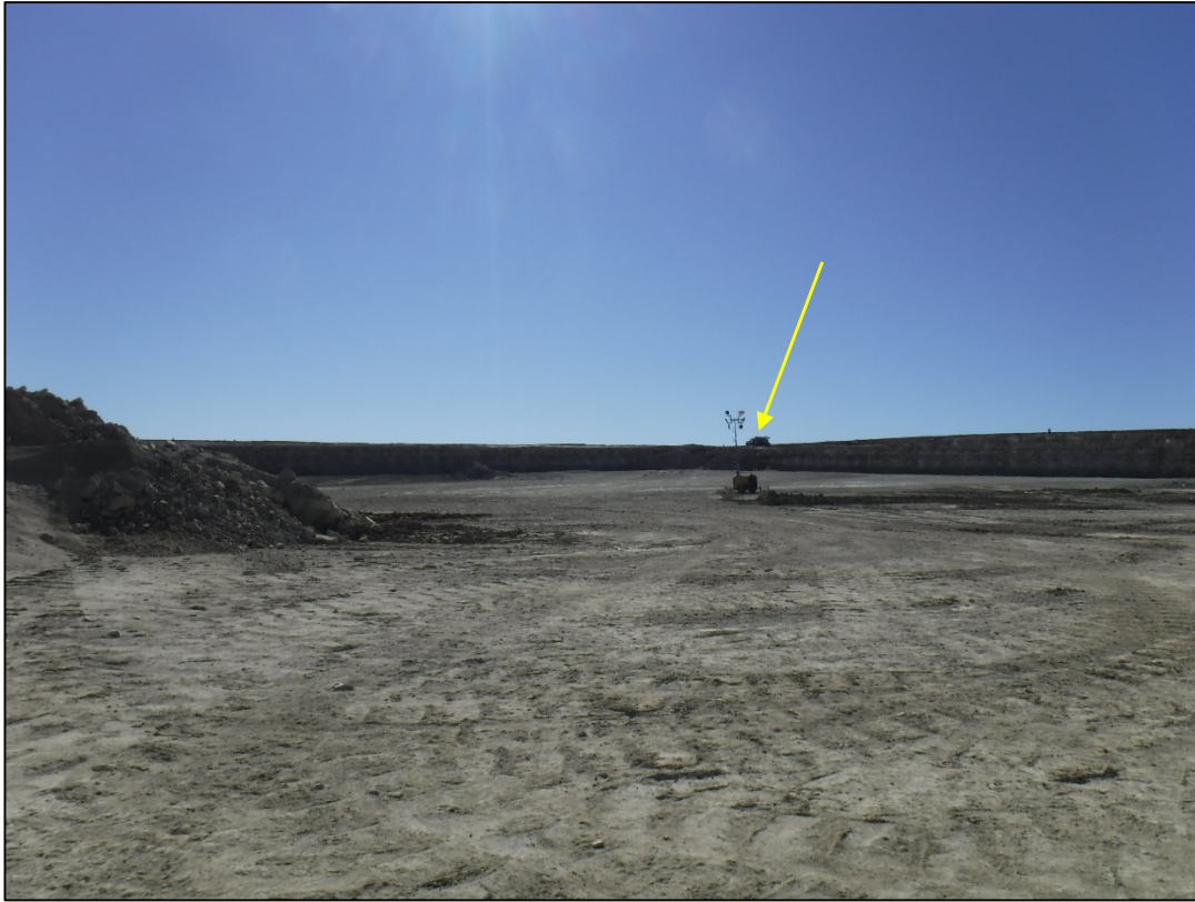
Photo 7: Active highwall area, yellow arrow shows ANFO truck loading blast holes
