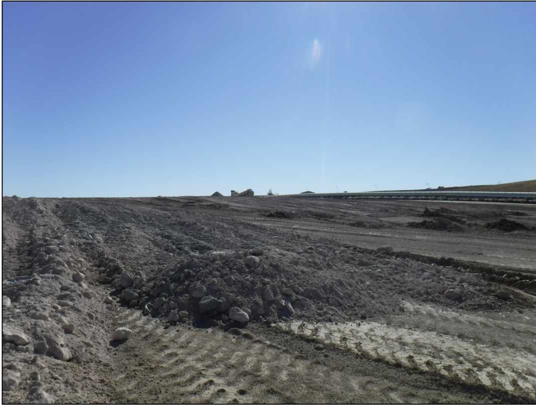
Photo 13: Bag house dust material being beneficially reused
