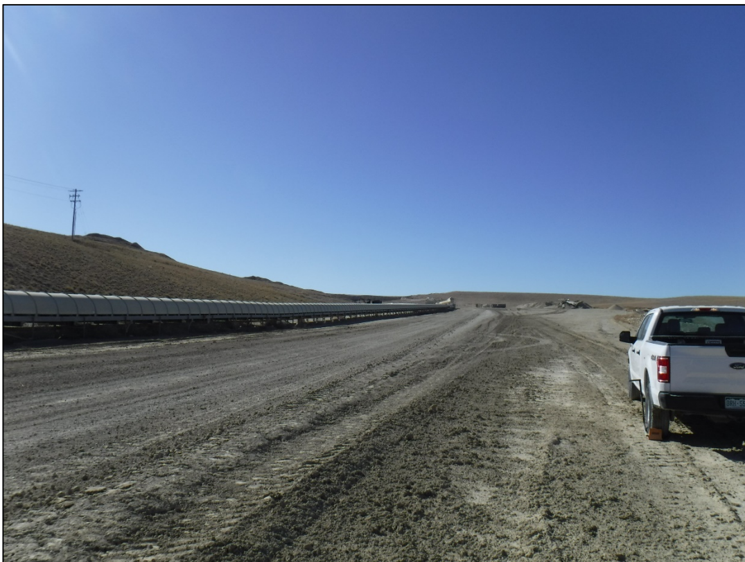
Photo 2: Conveyor leading to the active mining area
