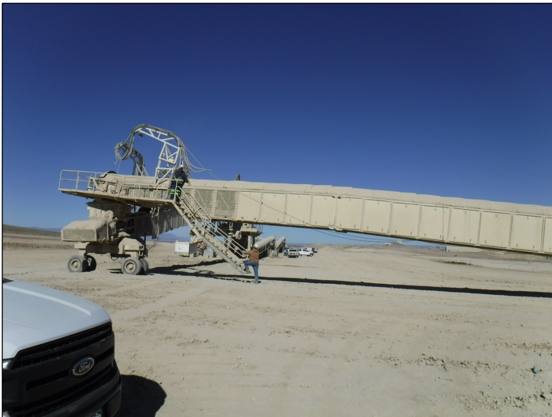
Photo 10: Mobile conveyor belt segments
