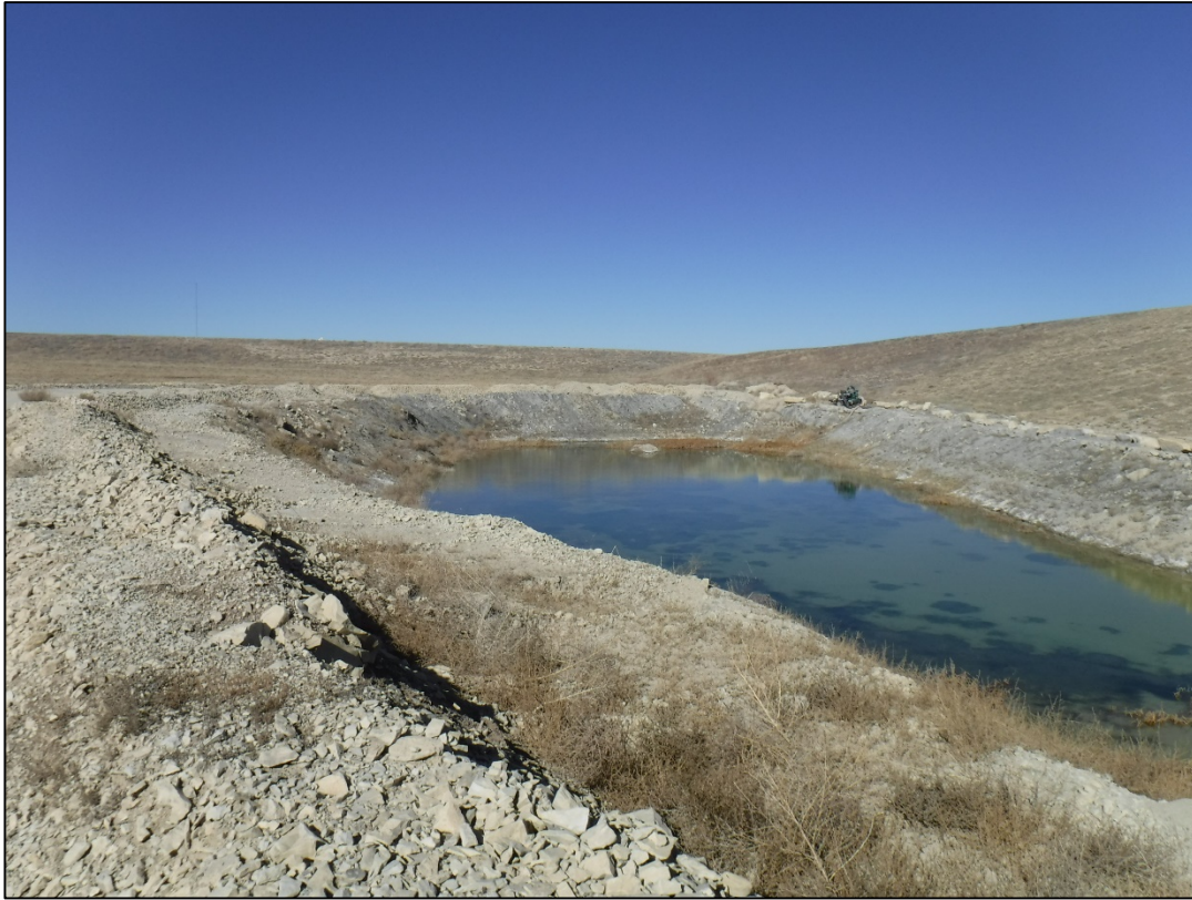
Photo 3: Stormwater detention basin, water from recent storm event
